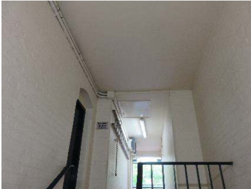
Access hatch to roof space in Beaumont Buildings
