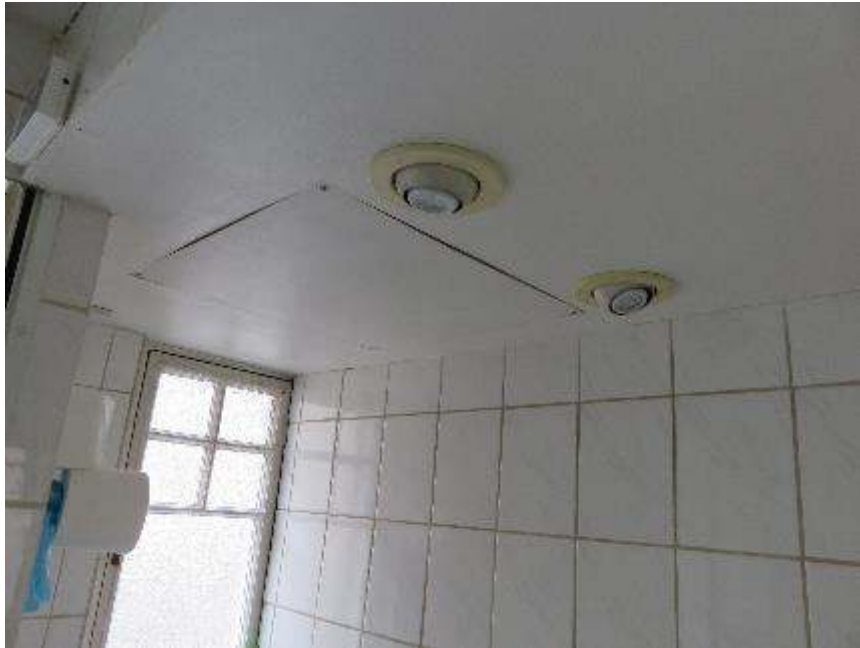
Hatch to access pipework above ceiling in flat in Sheridan Buildings.
