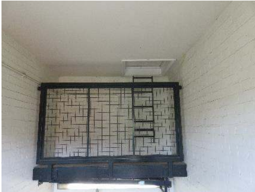
Arrangements for gaining access to roof space in Fletcher Buildings
