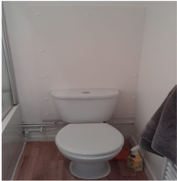
Fire Rated Panel Installation behind toilet cistern
