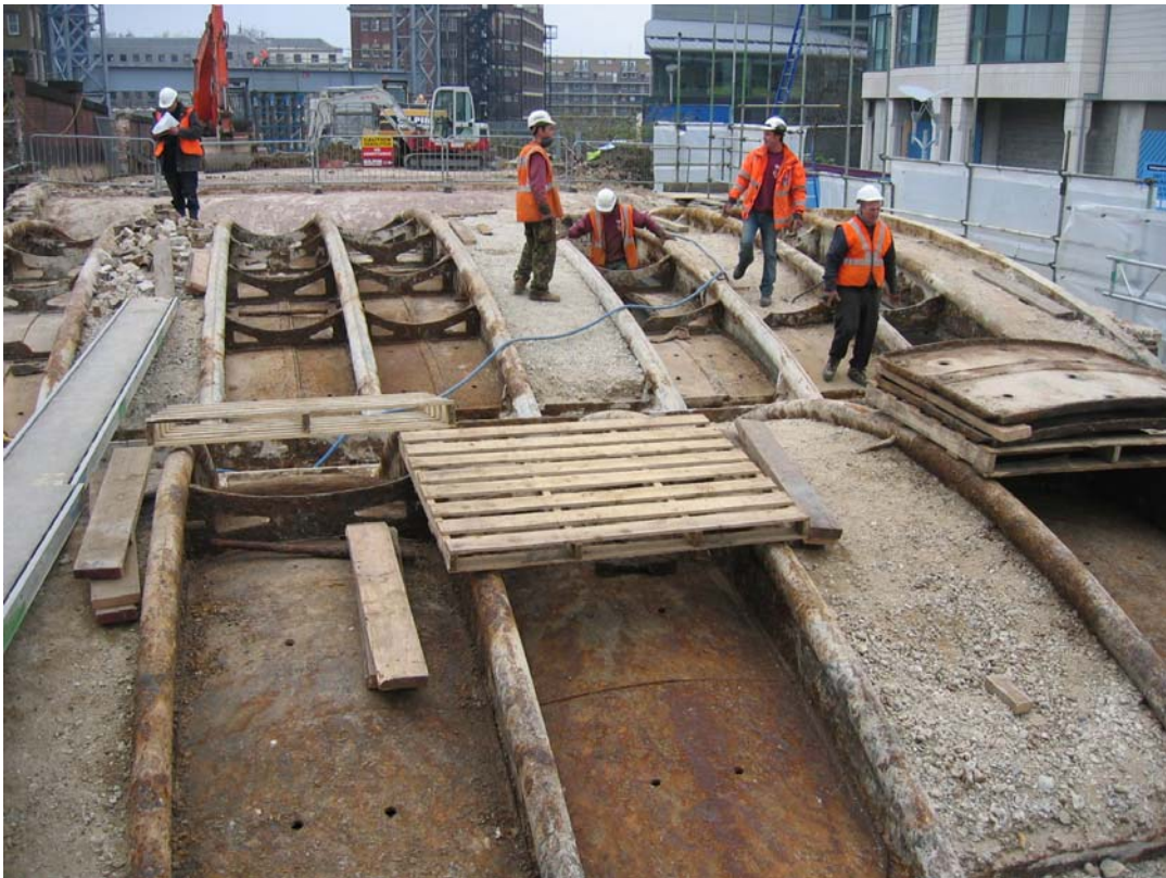
The structure of Brunel's bridge being uncovered prior to removal to storage.
