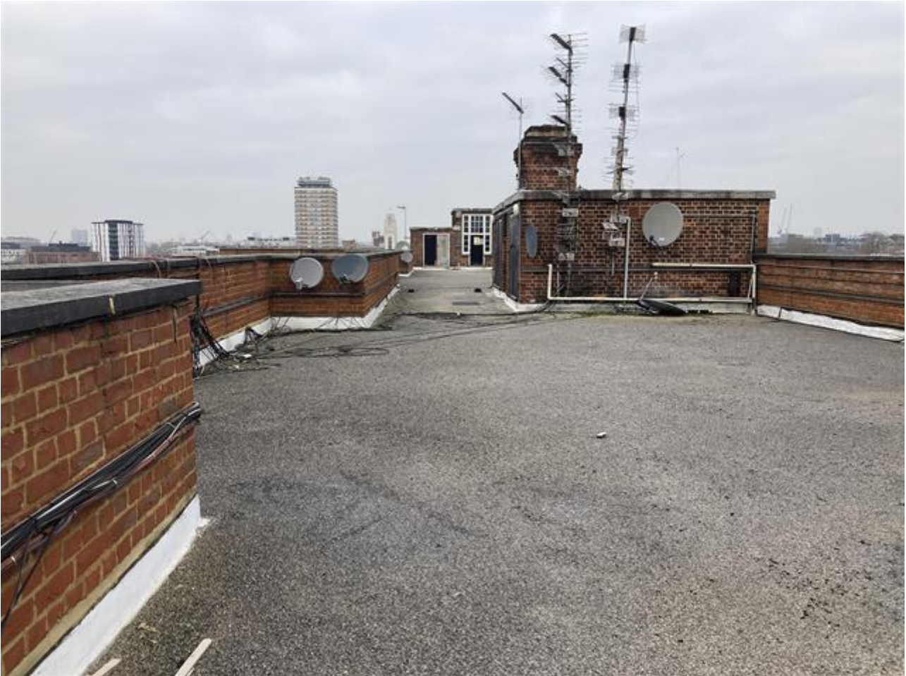
Overview of main roof.
