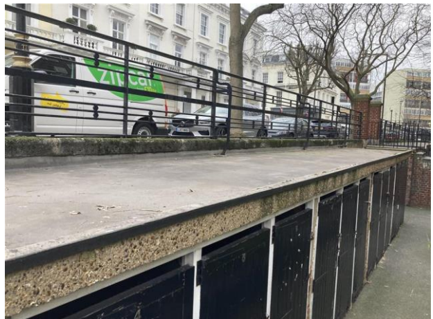
Pram shed roofs currently considered suitable to overlay.
