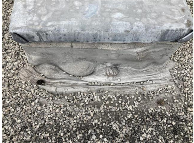
The exposed asphalt is badly blistered and slumping in areas.
