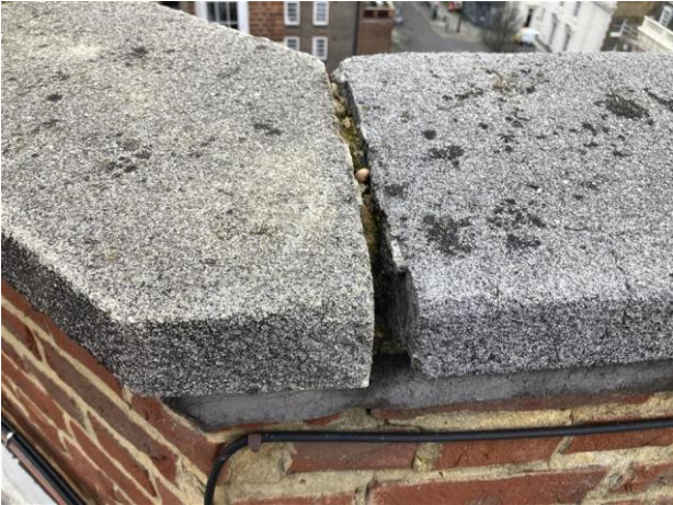
Advisory - coping stones should be repointed or encapsulated.
