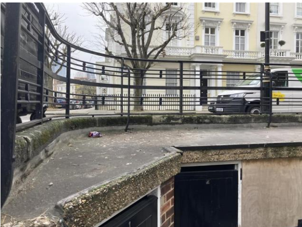
Overview of pram shed roofs.
