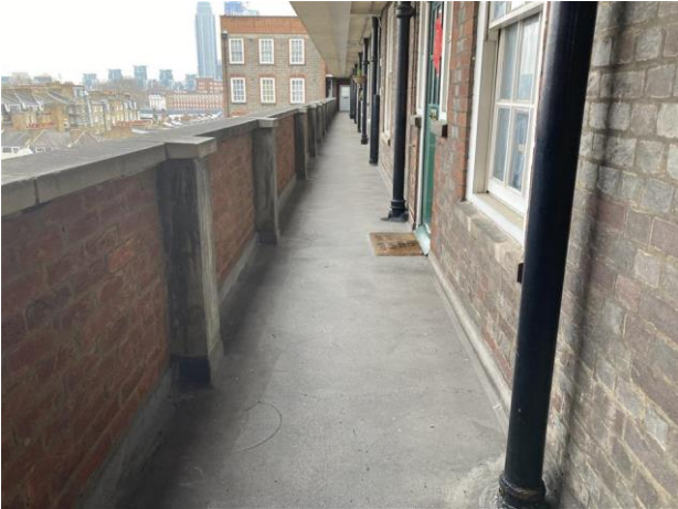
Overview of typical walkway.
