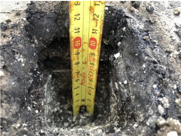
Existing insulation cut-to-falls.
