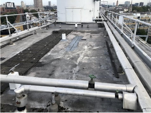
Overview of main roof.
