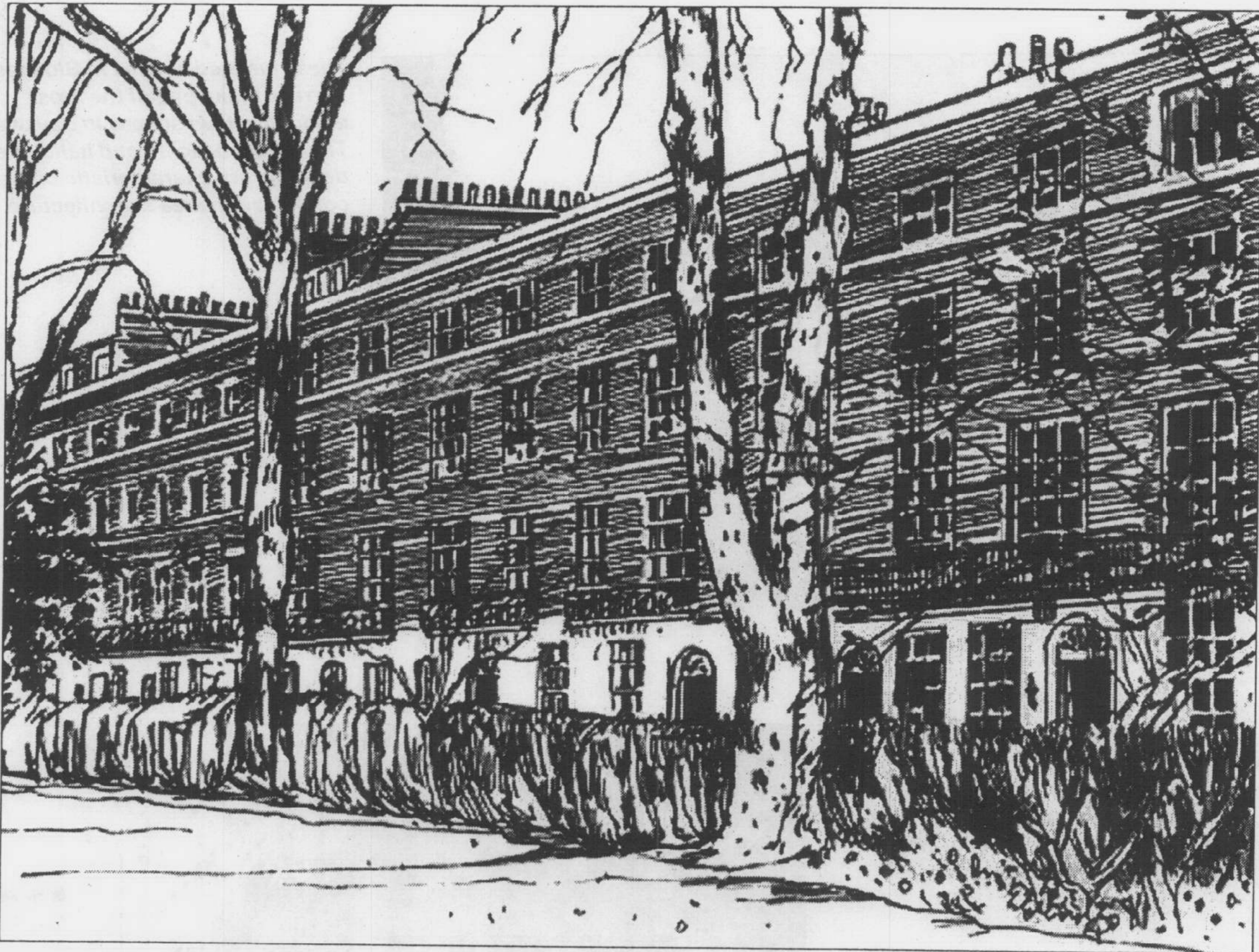
Connaught Square, developed from 1807 by S. P. Cockerell for the Church Commissioners, is a very late example of Georgian estate development, with high quality facing brick to the upper floors and render below.
