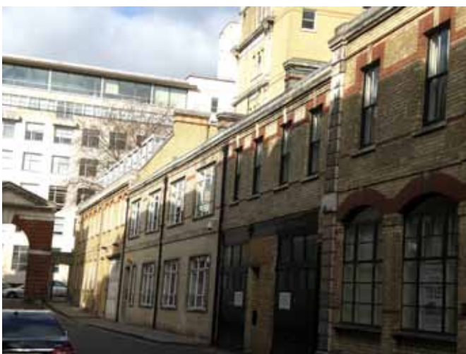
Figure 26: Mews buildings on Headfort Place
