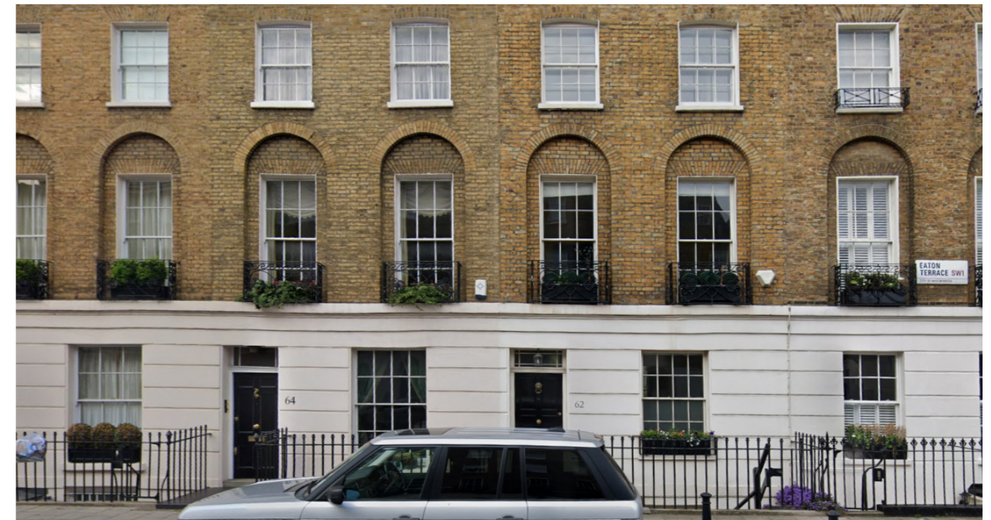
Fig 65. Round headed first floor brick window reveals (shown above) are a feature on buildings along the west side of Eaton Terrace and the north side of Chester Row. Whilst a typical feature of the period elsewhere, these round headed reveals are rare in Belgravia.
