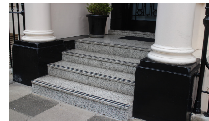
Fig 49. Small negative changes and the use of low quality and inappropriate materials, such as marbled granite in the above example, leads to the erosion on the area's character.
