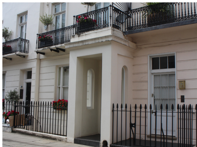
Fig 47. Infilled porticos have a negative impact as they are not sympathetic to the historic character of the area.
