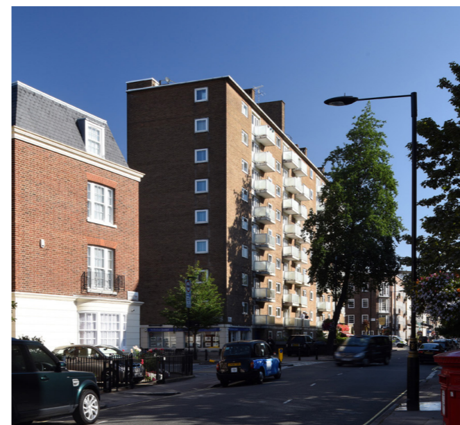
Fig 71. Kilmuir House breaks the order of the local context in favour of a high-rise modernist block. The rhythm of the terraces of South Eaton Place and Eaton Terrace is broken in favour of open space dominated by surface parking at the rear. This building is an example of insensitive urban planning during the post-war era.
