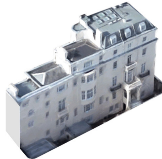
Fig 38. Street Elevations The street elevations on Eaton Place are ordered and the street design of individual buildings is developed in reference to its neighbours.
