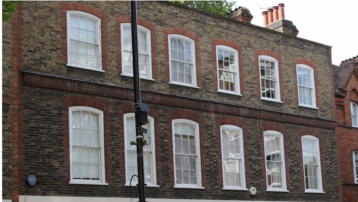
Fig 63. Several buildings along Ebury Street, near Orange Square, have very shallow window reveals (shown above). This is because these buildings were built in the early to mid-18th Century, before stricter fire regulations enforced deeper reveals and hence are a historic anomaly and not typical of the majority of Belgravia's buildings.
