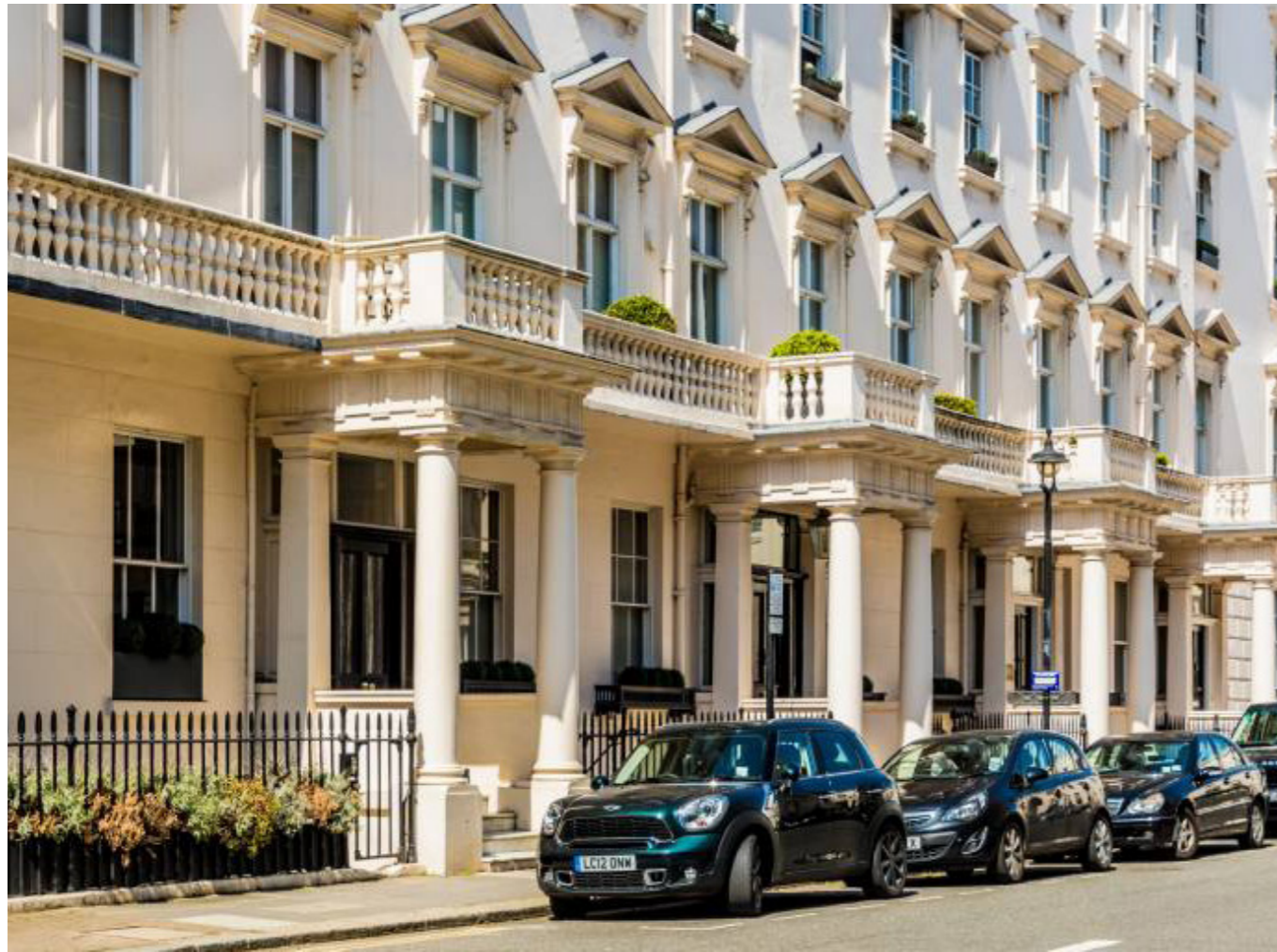
Fig 46. Entrance portico on Eaton Square. The portico performs a number of interrelated functions clearly denoting the position of the entrance, spanning over the ground floor and accommodating the step up to the raised ground floor. At first floor level the top of the portico provides external terrace space.
