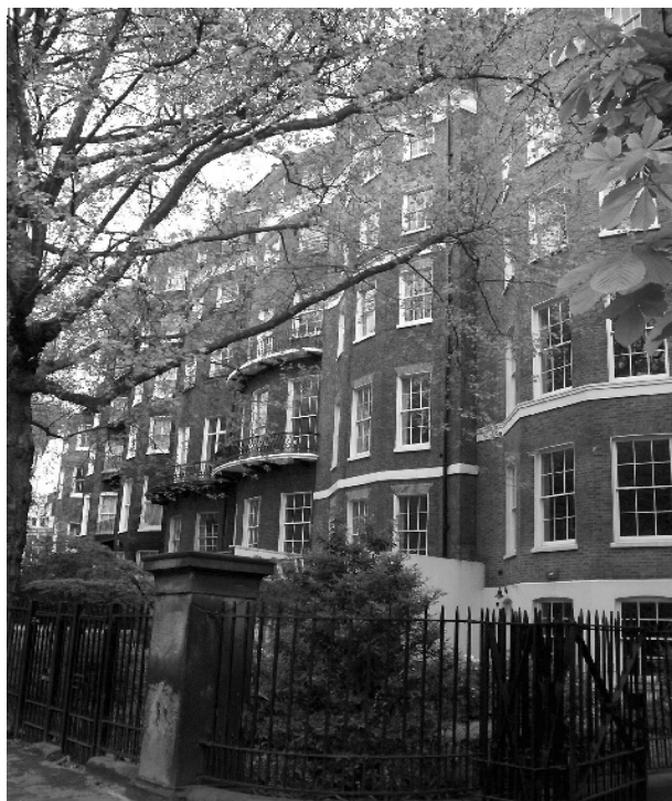
Figure 62: Bowed backs of nos. 22 - 36 Old Queen Street
