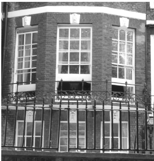
Figure 64: Canted back to no. 30 Queen Anne's Gate
