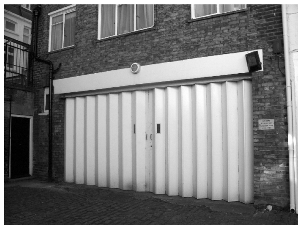
Figure 109: Steel doors in Buckingham Mews
