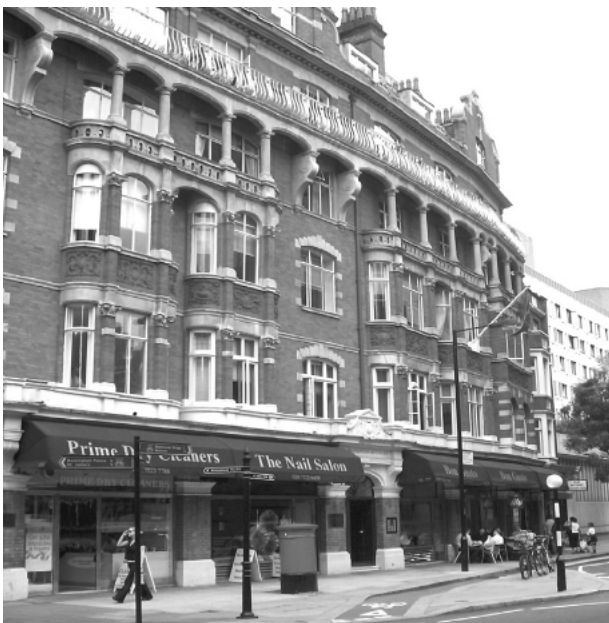
Figure 71: Nos. 75 - 81 Buckingham Gate
