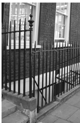
Figure 76: Original railings along Buckingham Gate
