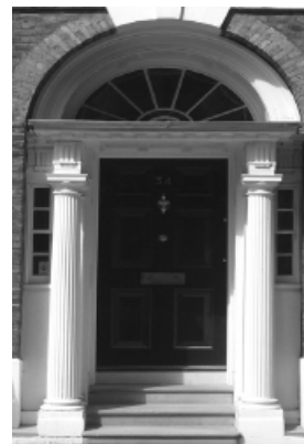
Figure 59: Recessed doorcase with fluted columns at no. 32 Old Queen Street
