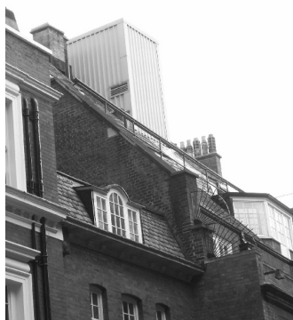
Figure 105: 16 Old Queen Street
