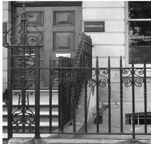
Figure 82: Late 19th century railings using wrought iron at 21 Buckingham Gate
