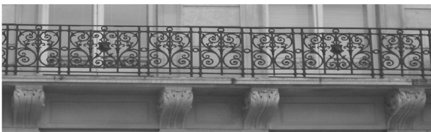
Figure 81: Victorian balcony to the Buckingham Palace Hotel
