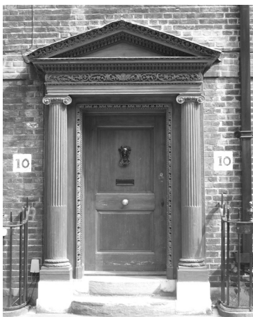
Figure 19: Reused 18th century doorcase at 10 Catherine Place
