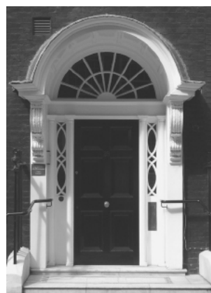
Figure 58: Doorcase with panelling in the arched recess and transom light detail at no. 28 Old Queen Street
