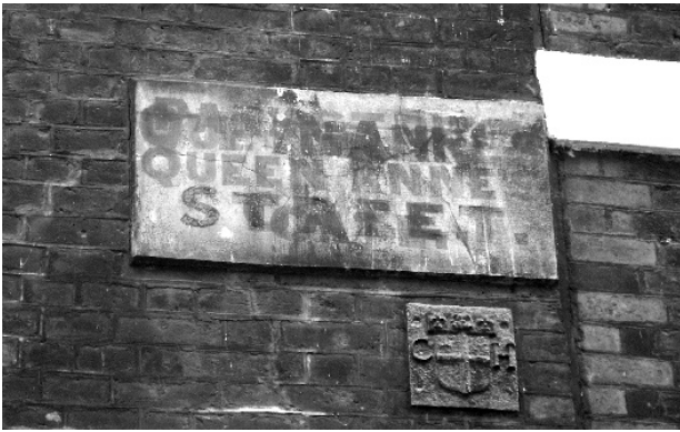
Figure 94: Historic Street Sign for Queen Anne Street
