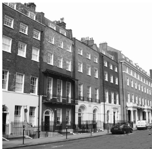
Figure 55: Nos. 14 - 22 Queen Anne's Gate
