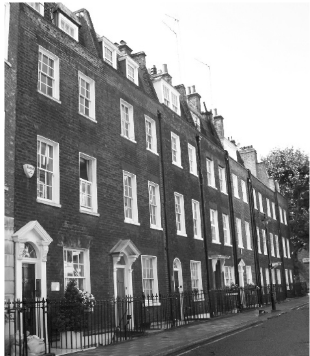
Figure 22: Simple two bay late Georgian terraces at 30-42 Catherine Place
