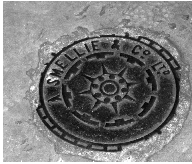
Figure 100: Coal Hole Cover to Queen Anne's Gate
