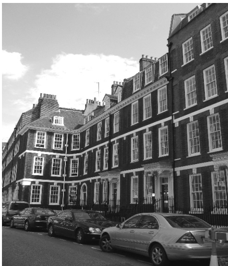
Figure 46: Nos. 15- 19 Queen Anne's Gate
