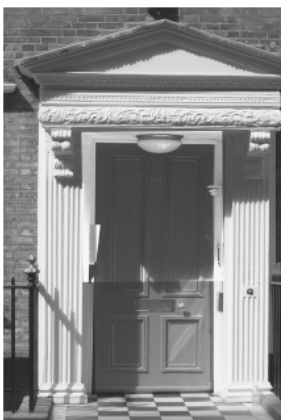
Figure 57: Pedimented doorcase with fluted pilasters and consoles at no. 24 Old Queen Street
