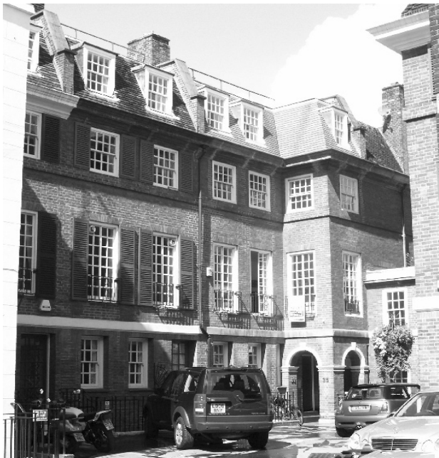
Figure 18: 29-37 Catherine Place in a simplified neo-Georgian/ neo-Queen Anne style, with high pitched clay tiled mansard and overhanging eaves cornice
