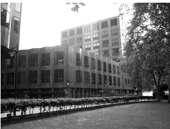
Figure 17: Rear of 50 Victoria Street, viewed from Christchurch Gardens.
