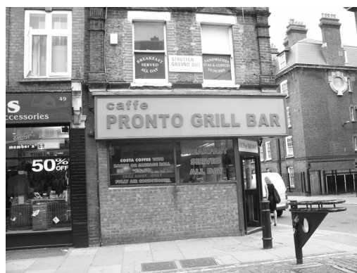
Figure 75: 51 Strutton Ground. This shopfront relates poorly to the building in which it is set. The very high stallriser has been built in brick which does match the brick to the upper floors and the large plastic fascia
