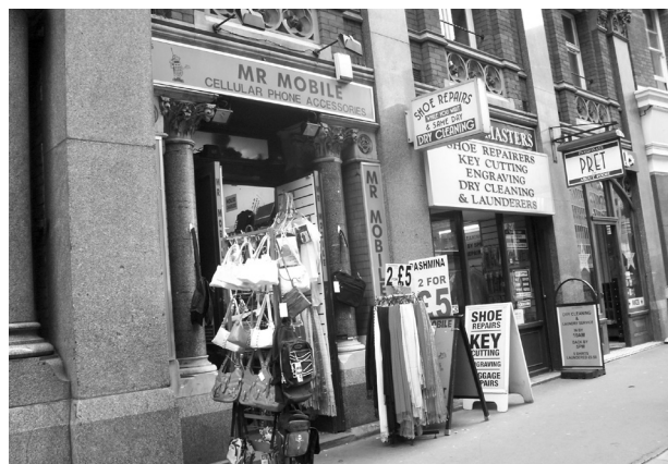
Figure 74: The range of signage at 75 and 75a Victoria Street is out of character with the host building, and causes both visual and physical clutter
