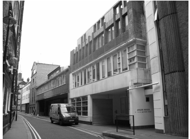
Figure 26: St Matthew Street
