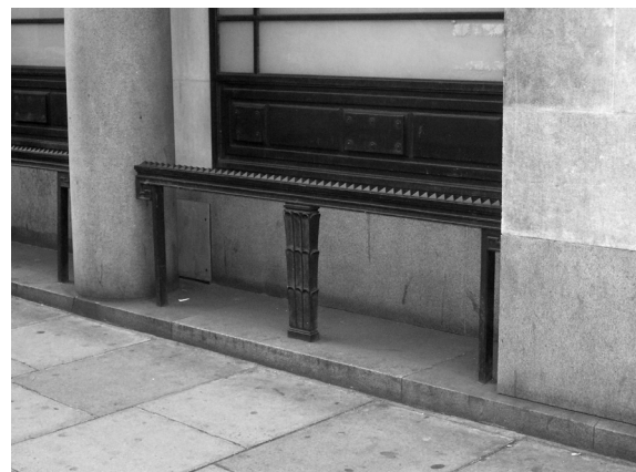
Figure 54: Bronze rails to St James Park Underground
