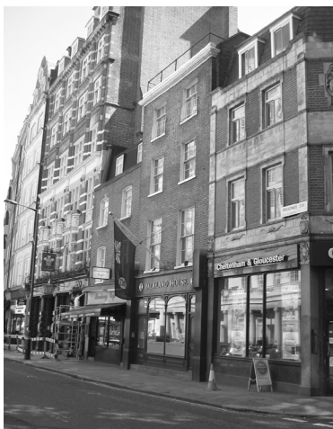
Figure 38: Group of Unlisted Buildings of merit including 12-16 Broadway and the Feathers Public House
