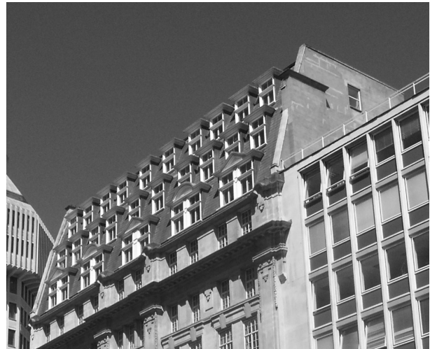
Figure 41: Many buildings in the conservation area already have mansard or other roof extensions
