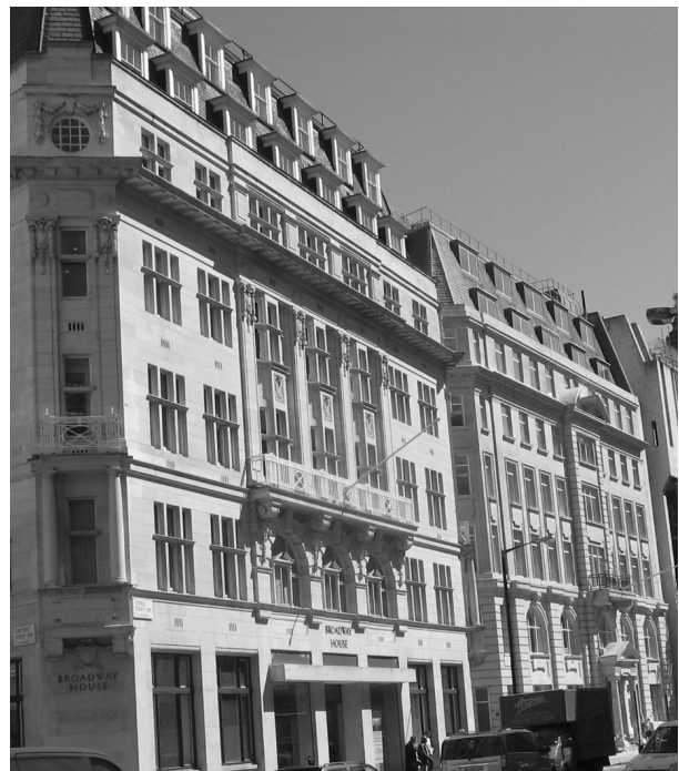
Figure 35: Broadway House, Tothill Street
