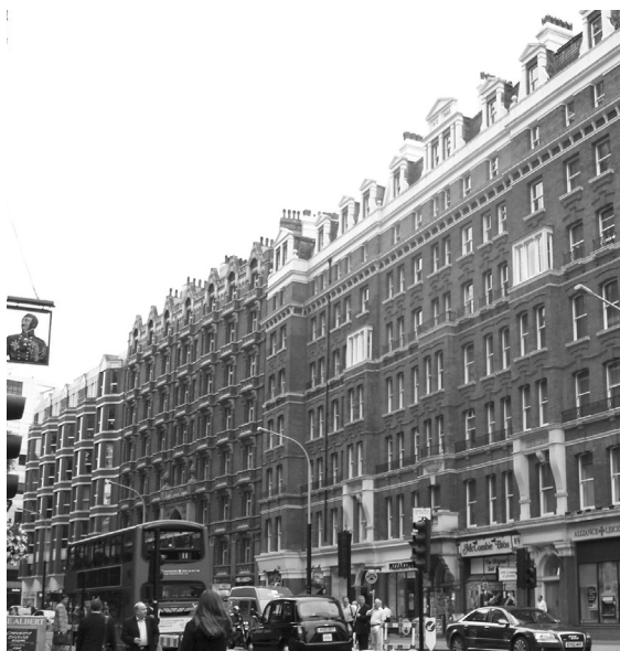
Figure 13: South Victoria Street, with Artillery Mansion at the centre and nos. 77-93 to the right in the foreground.
