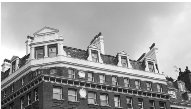
Figure 40: Typical mansion block roof treatment, with mansard roof with tall chimneys and dormers.
