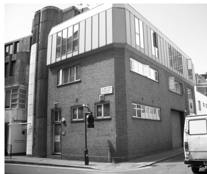
Figure 85 -6: 2-4 Old Pye Street
