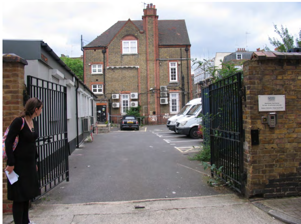
Looking east from Stalbridge Street, through the site's car park towards 29 Cosway Street, with the temporary portacabin on the left
