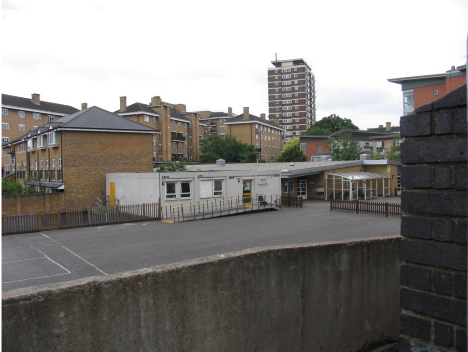
Looking south through the gate in the Luton Street wall, towards the vacant white portacabin, the residential terrace on Capland Street to the left, and the single storey yellow brick nursery building to the right
