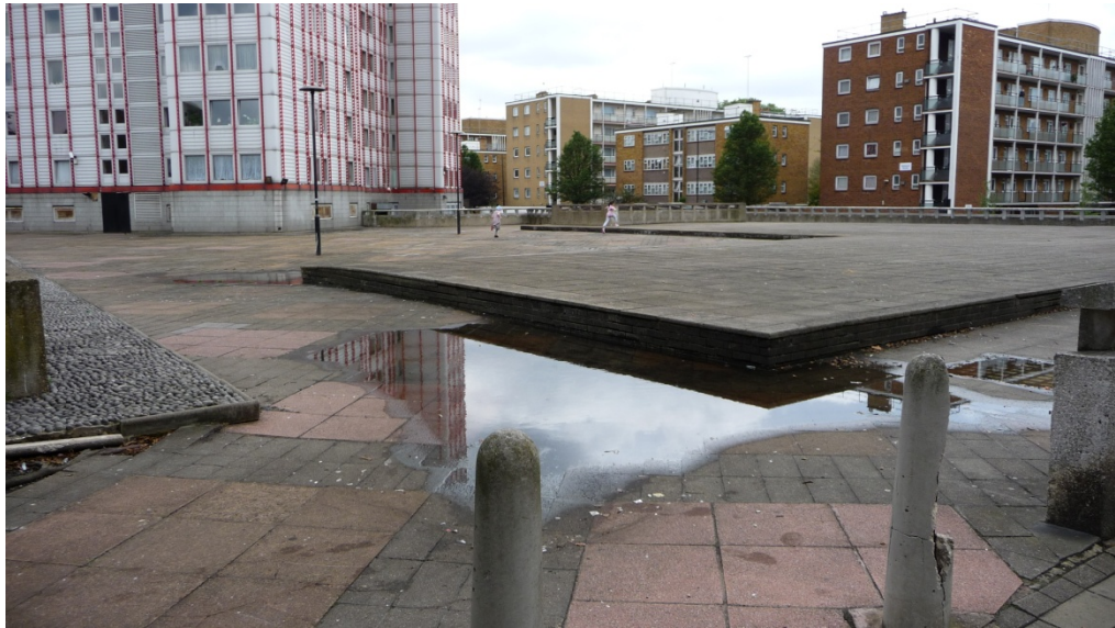
Looking from Crompton Street, south across the site, towards Hall Place
