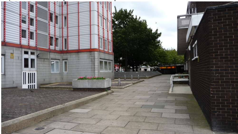
Looking east towards Edgware Road, with the brick podium containing trees ahead
