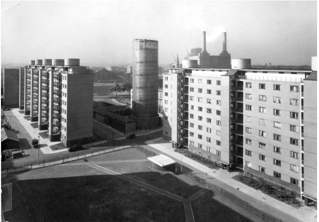
Figure 5: Churchill Gardens looking towards Battersea (RIBA library photograph collection)
