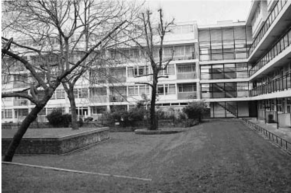
Figure 12: Continuous Blocks of Five storeys from the final phase
