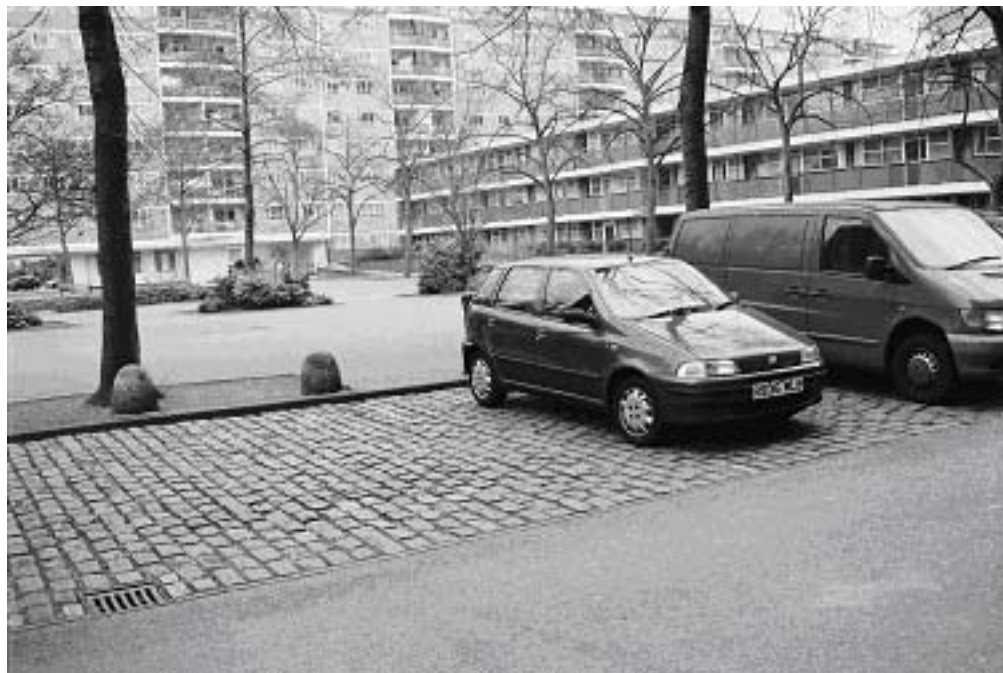
Figure 29: Granite setts mark out car-parking areas
