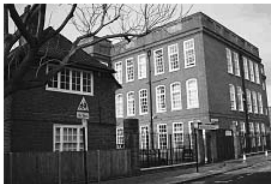
Figure 19: Churchill Gardens Primary School.
