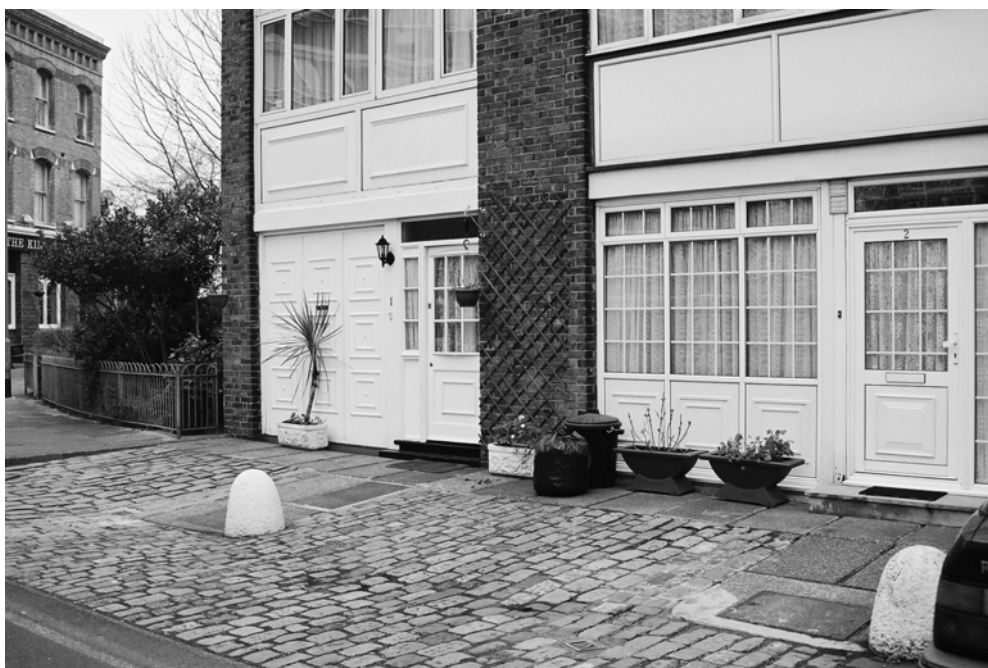
Figure 32: uPVC replacement doors and windows
