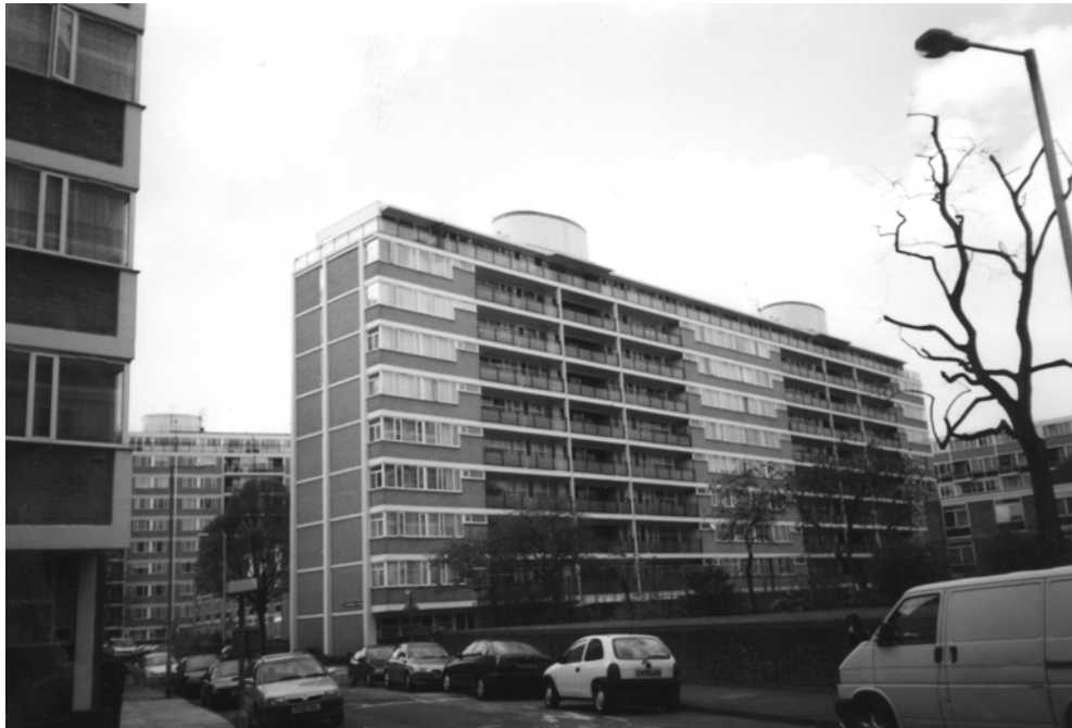
Figure 10: Later Blocks with gallery Access
