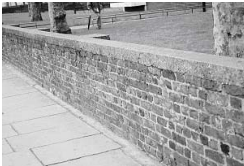
Figure 24: Brick Wall to Grosvenor Terrace
