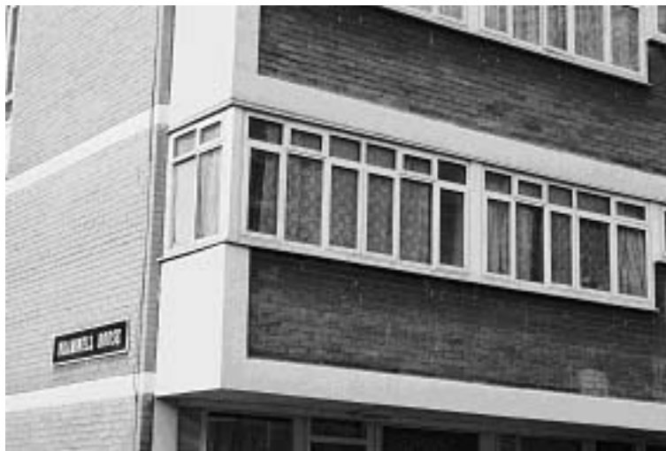
Figure 17: Early phases of replacement windows with toplights (Bramwell House)
