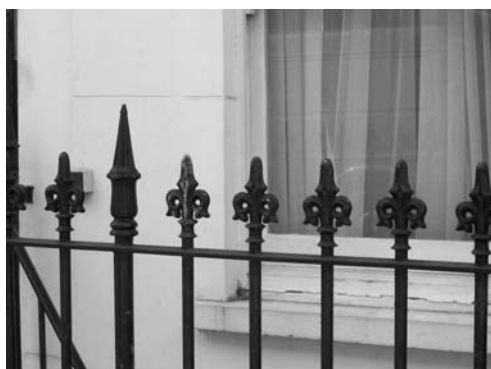
Figure 29: Replacement railings at No. 147
