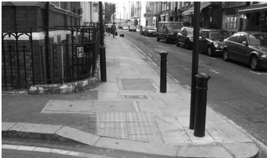
Figure 32: The street surface along Cleveland Street has been recently re-paved, but the surface treatment does not continue into Carburton Street.
