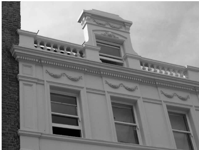
Figure 23: Distinctive roofline of No. 151 the 'George and Dragon.'
