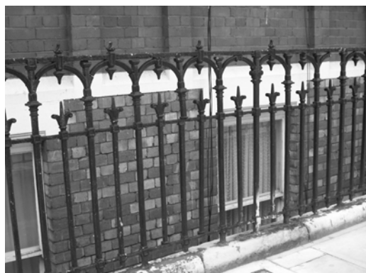
Figure 27: Railings outside the Victorian Mansion block, Nos. 127-133
