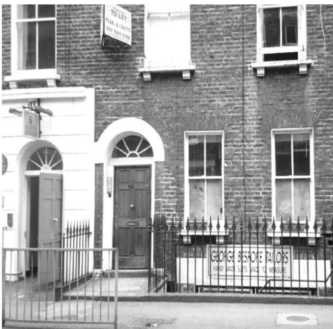
Figure 7: No 143, the only property with original ground floor treatment. Retaining two sashes and the lightwell, although with a modern shopfront to the basement.
