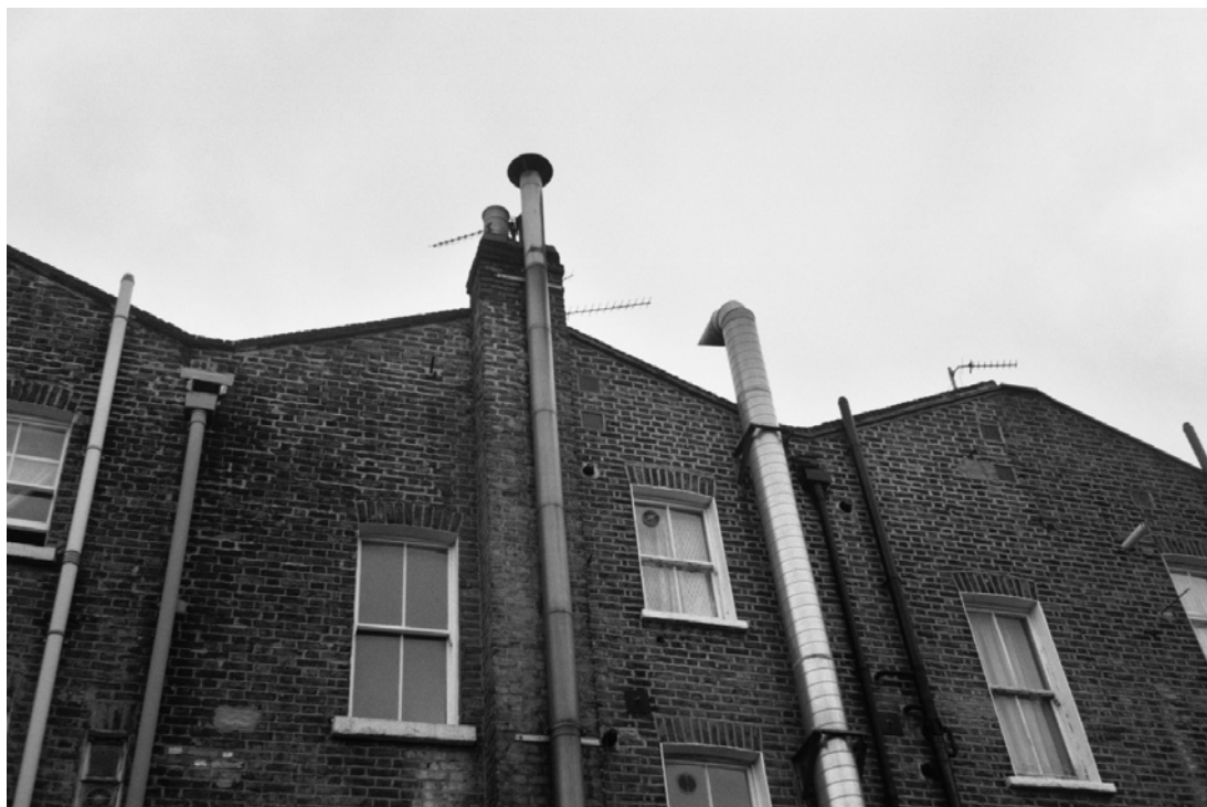
Figure 34: Flues to the rear of the terrace.
