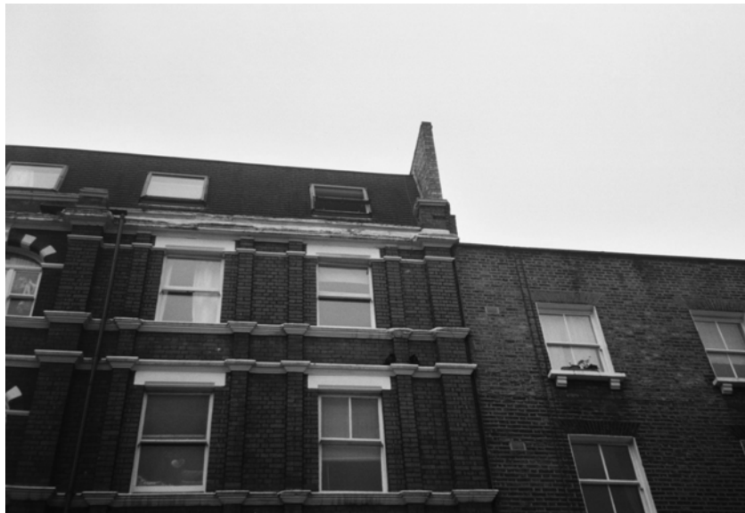
Figure 24 : The modern mansard roof is out of scale with the Georgian terrace it adjoins.
