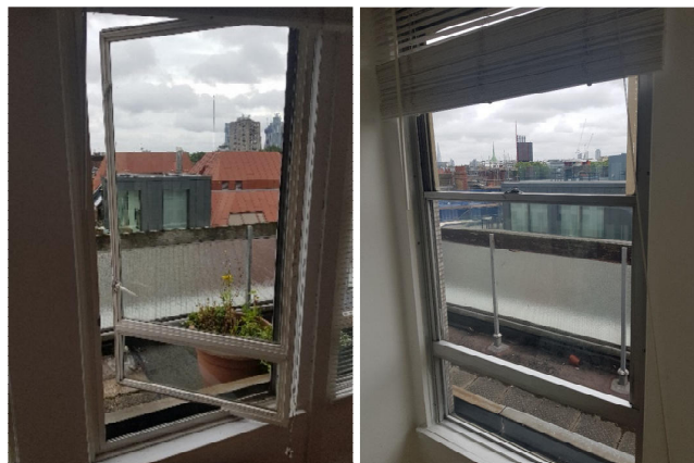
Photographs Windows internal 6 th floor Offset pivot and sash
