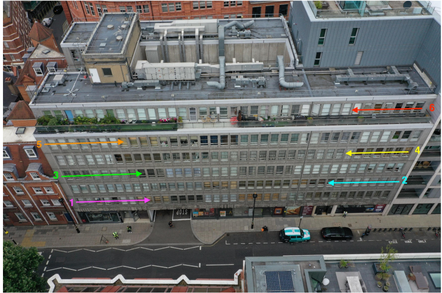
Photograph: East Elevation Rochester Row comprising 222No. windows
