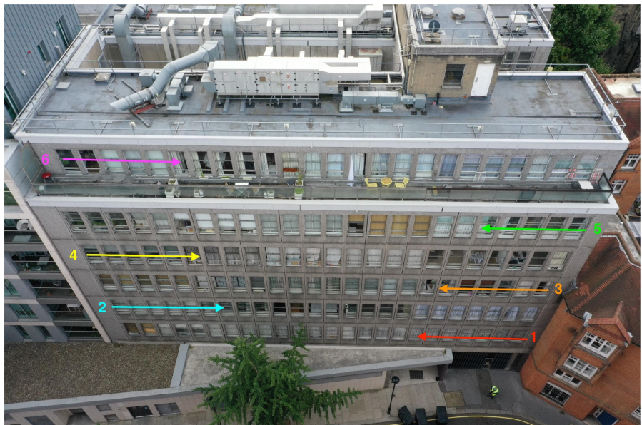
Photograph: West Elevation Greencoat Place comprising 144 windows (lightwells another 45 windows)
