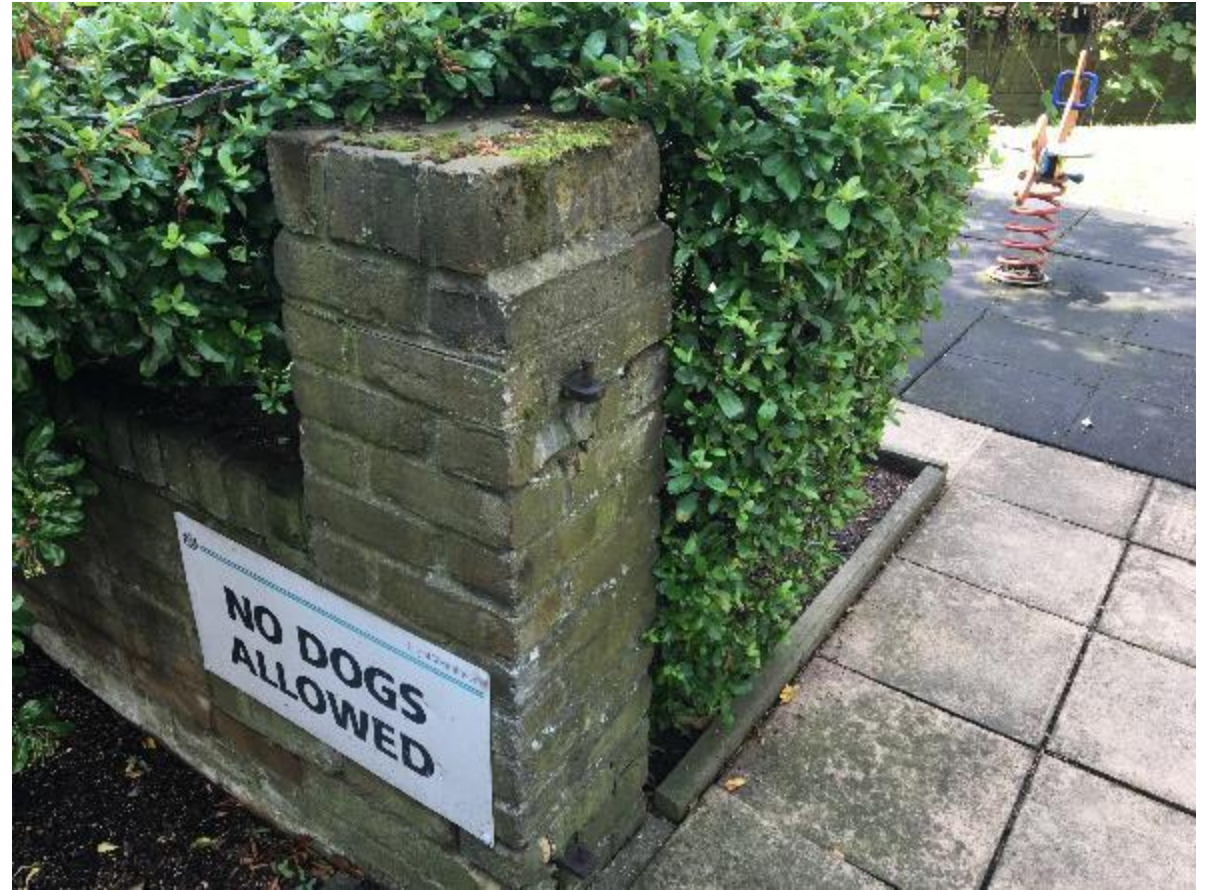
Photo 146. Gate missing from play area.
