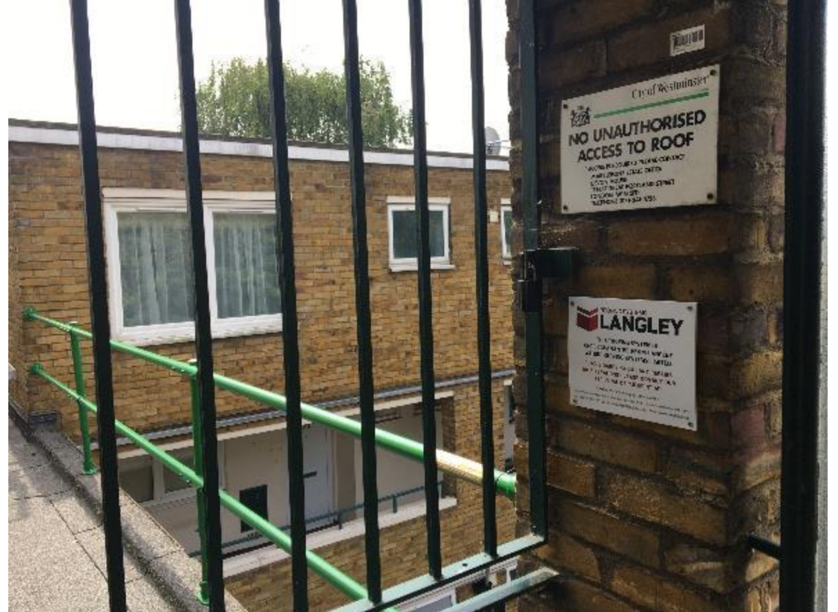
Photo 36. Evidence of roof covering replacement/overlay.
