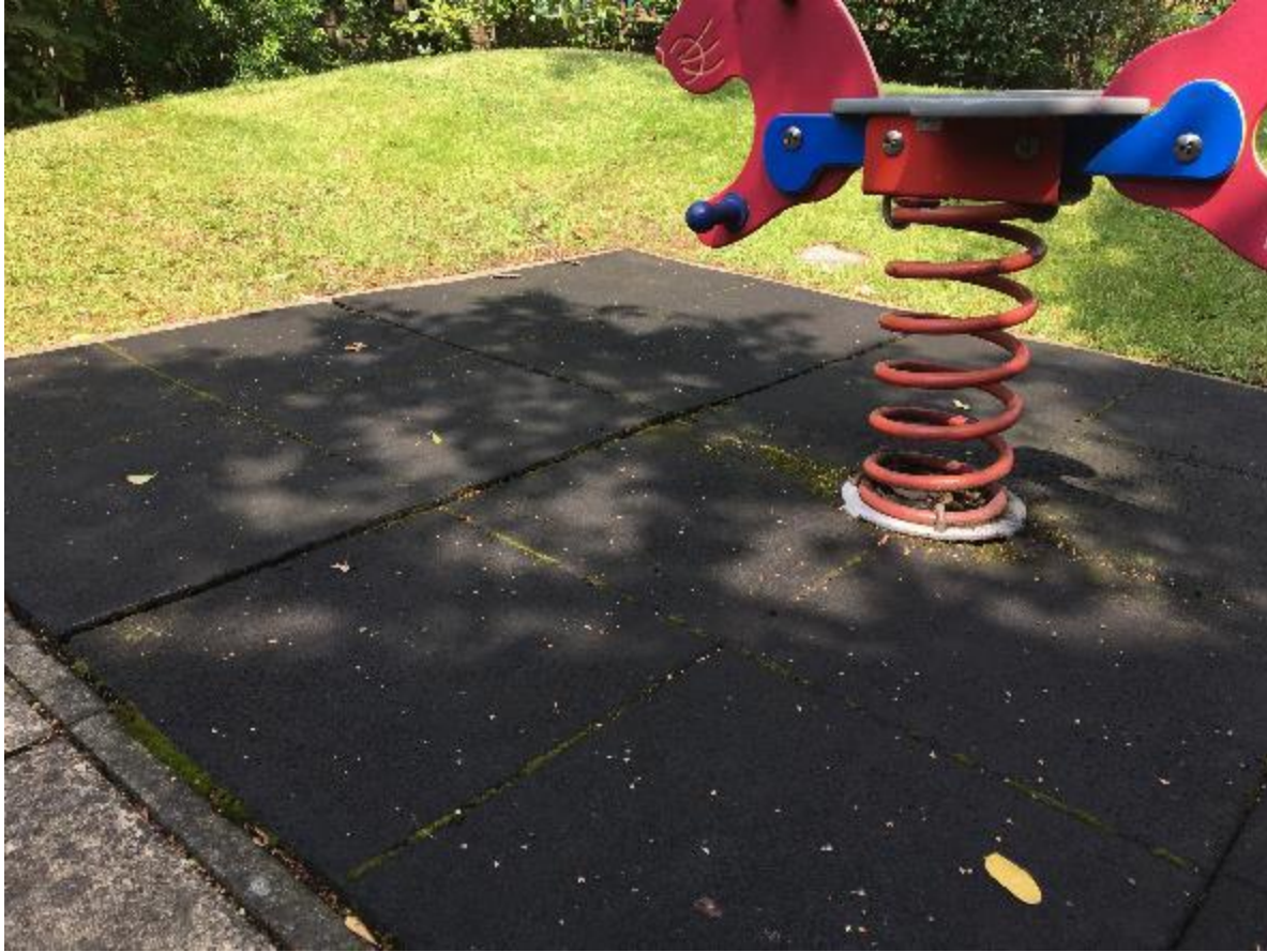
Photo 147. Edges of rubber matting lifting.
