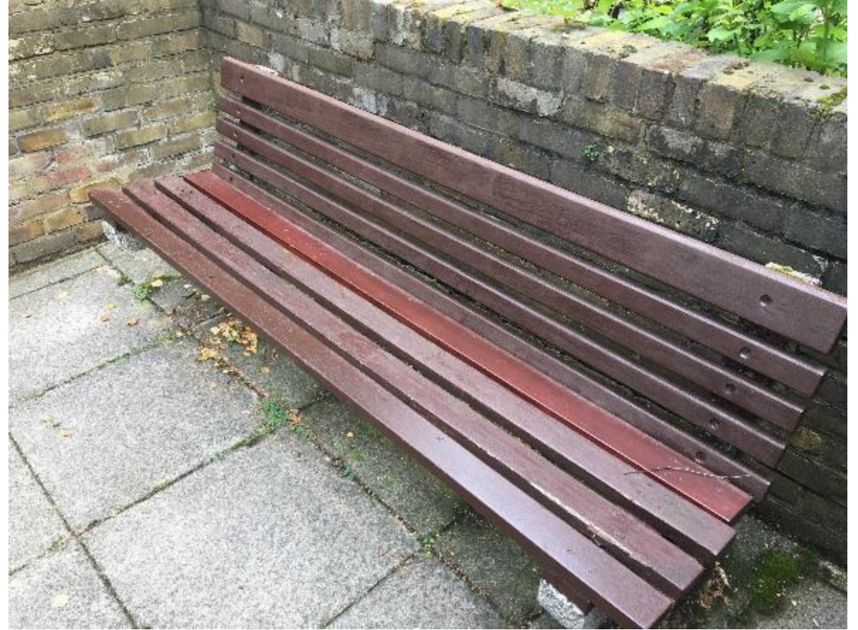
Photo 148. Decorations to bench starting to fail.
