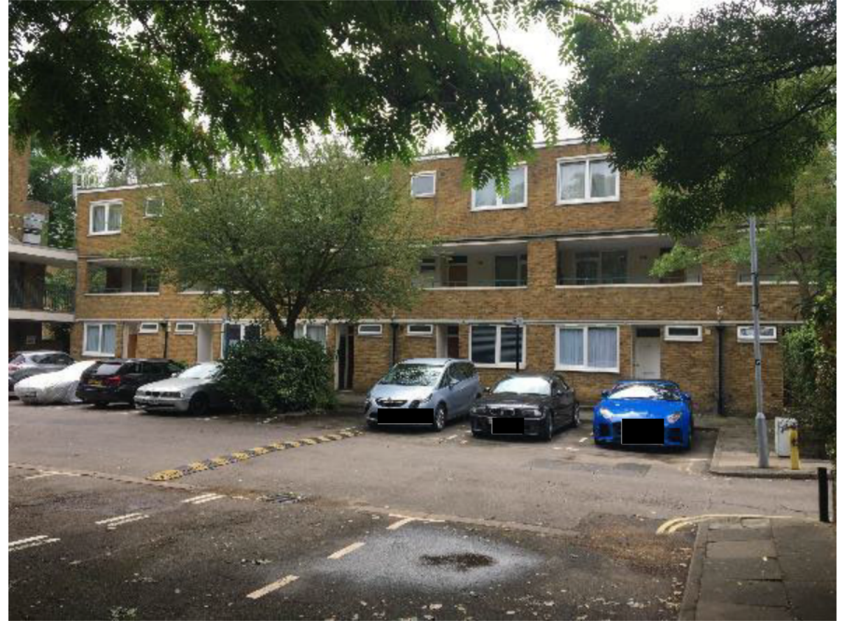
Photo 152. Carpark in front of Mordern Hse where the tarmac is starting to break up particularly near the entrance.
