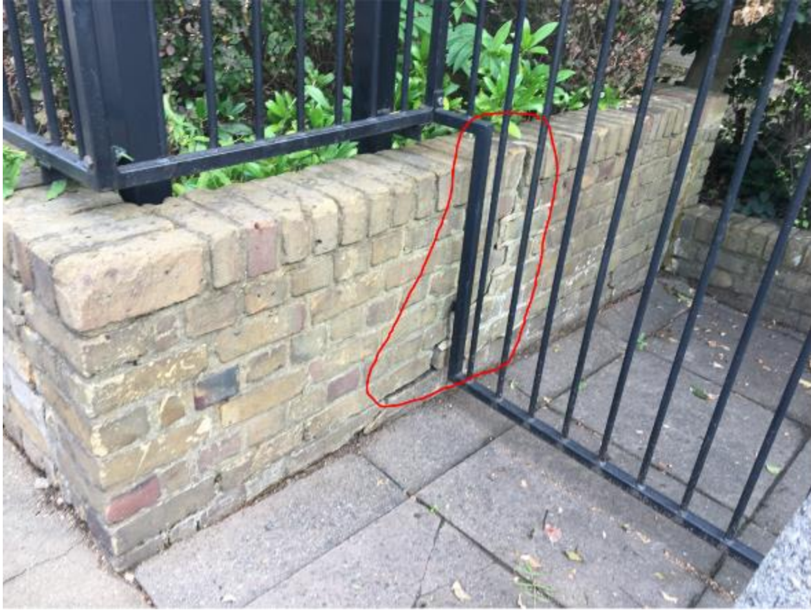
Photo 159. Showing return of same wall.
