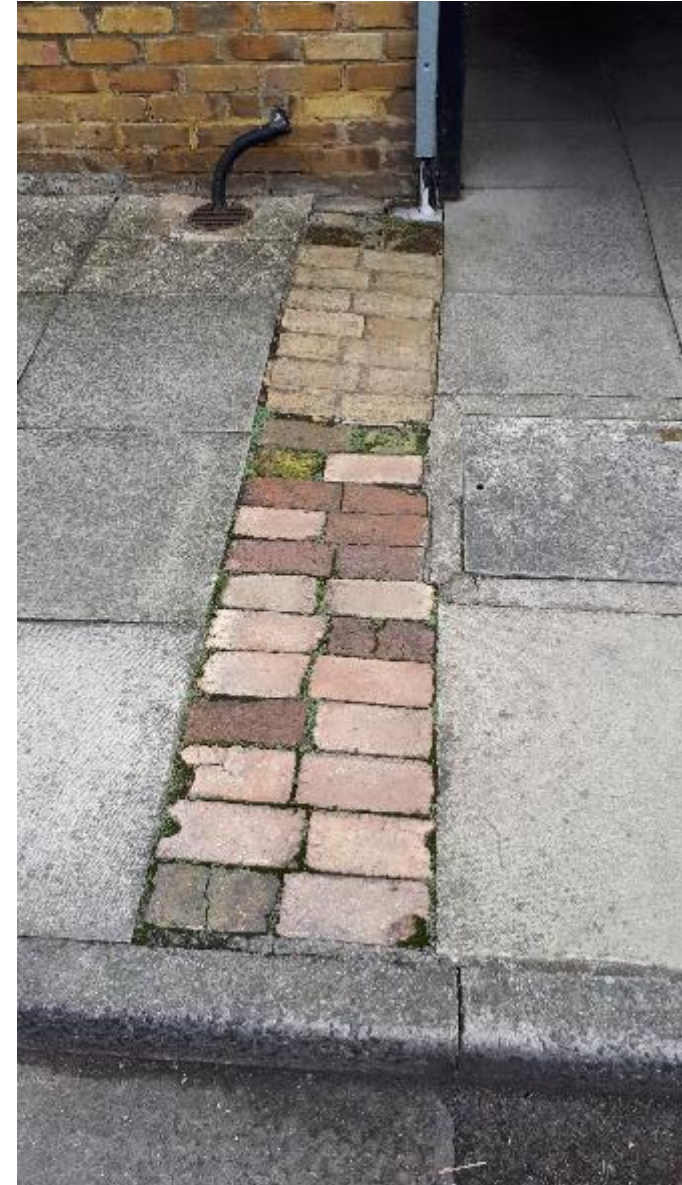
Photo 144. Interesting detail, bricks more susceptible to wear than pavers
