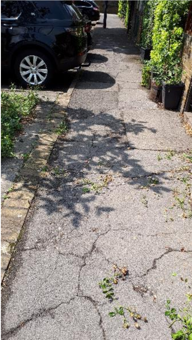
Photo 137. As previous photo.
