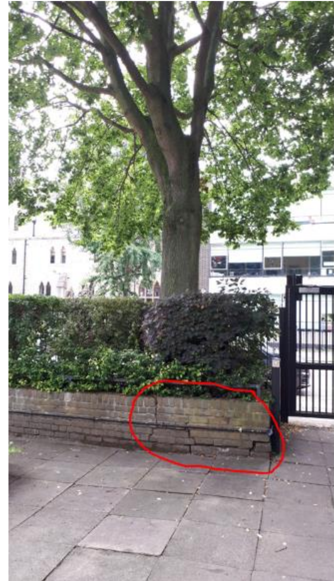
Photo 126. As elsewhere across the Estate, there is little else that can be done other than to keep repointing and re-bedding bricks as well as lop trees, those to public footpaths are assumed to have Preservation Orders.
