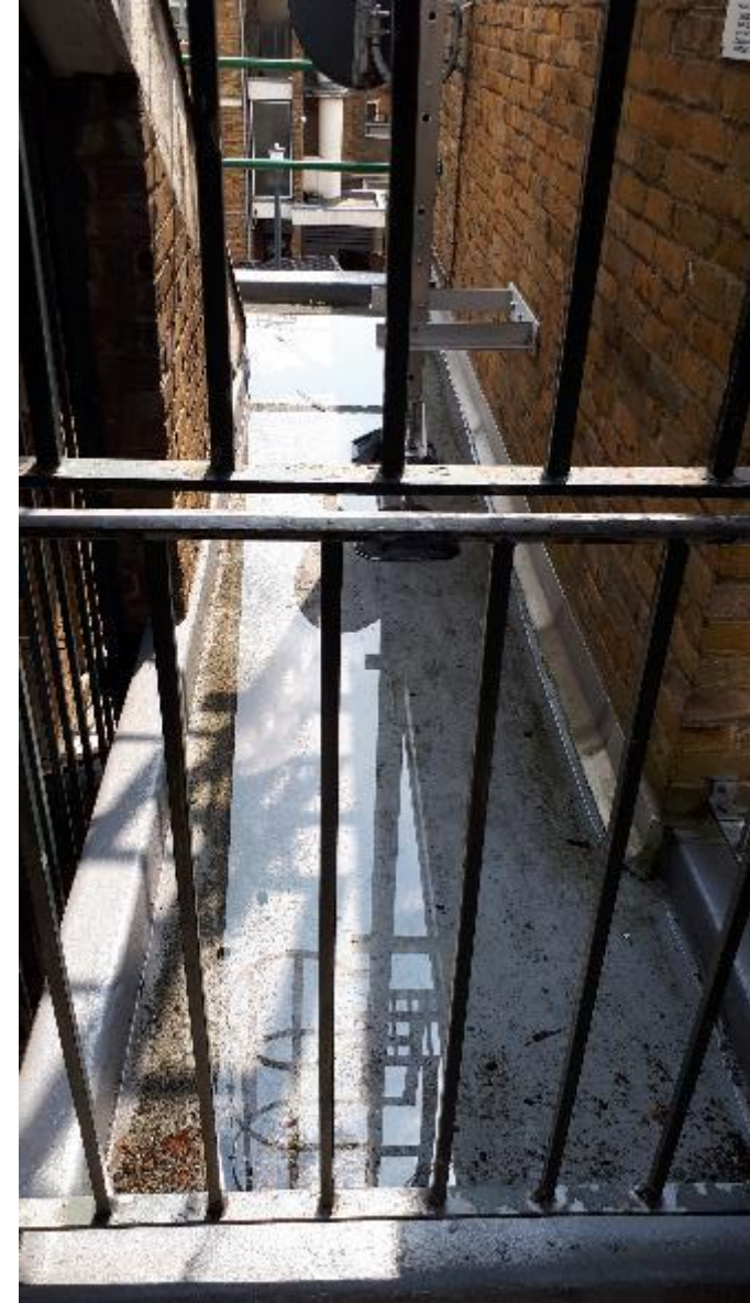
Photo 62. Flat section of stairwell roof.
