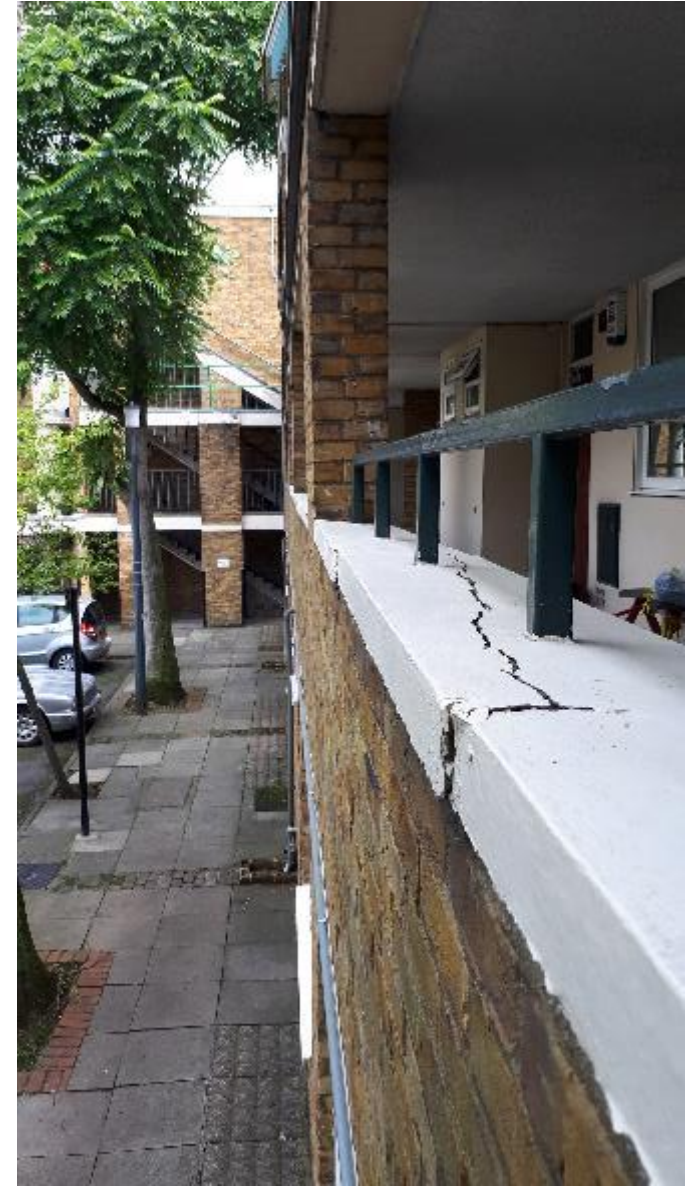
Photo 100. As previous photo.
