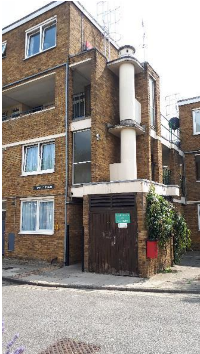
Photo 89. Farnham Hse communal stairs and bin store.
