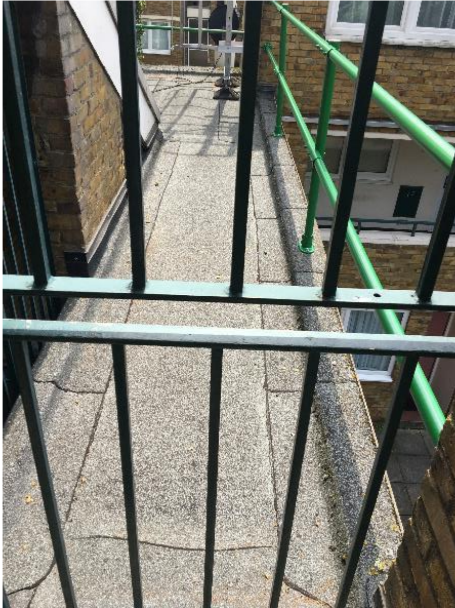
Photo 37. Showing replacement/overlayed felt system.
