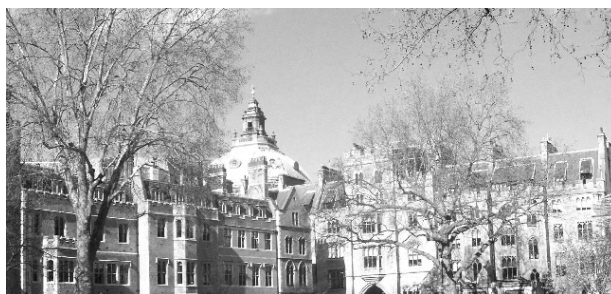
Figure 77: Roof profile of the north-west corner of Dean's Yard with the Methodist Central Hall in the background
