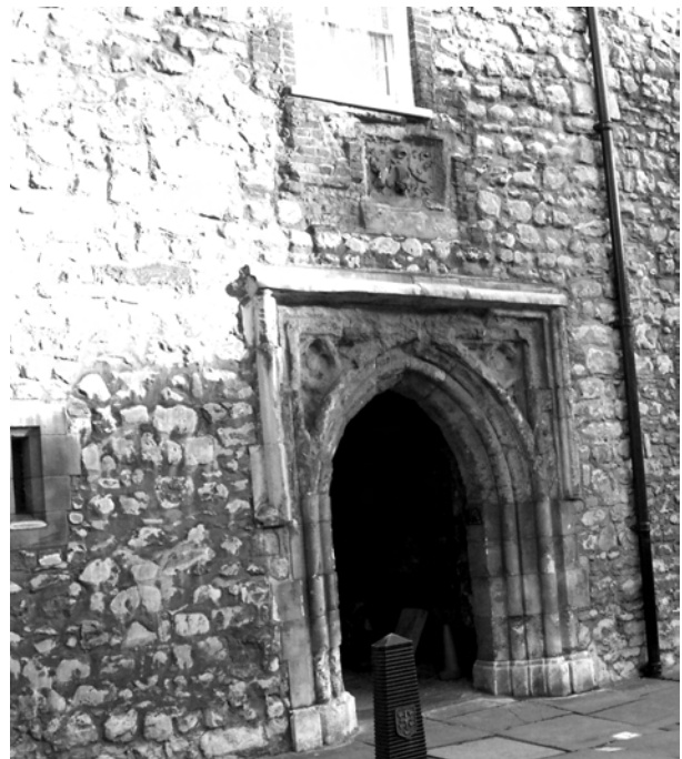
Figure 56: 16th century entrance to the Blackstone Tower
