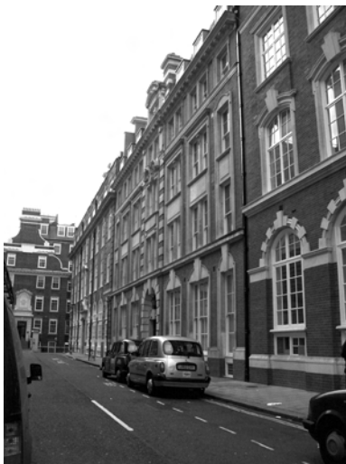
Figure 38: Edwardian buildings on Matthew Parker Street
