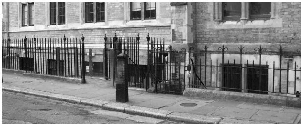
Figure 97: Elegant railings, No. 3 Dean's Yard
