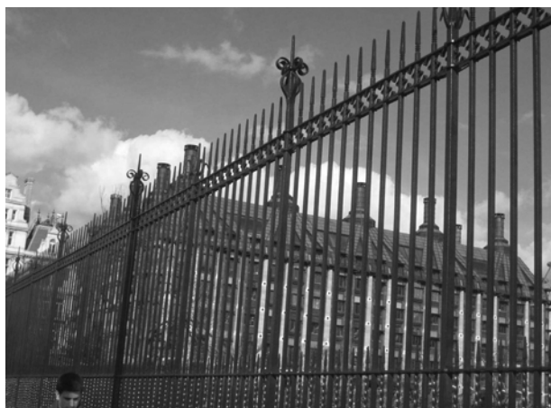
Figures 84-85: ( Above ) Railings to Cromwell Green Visitor Entrance (2007) by Architects Design Partnership. ( Below ) Houses of Parliament gates and railings (c.1869). Portland stone and cast iron. Gate piers with gablet-spire caps.
