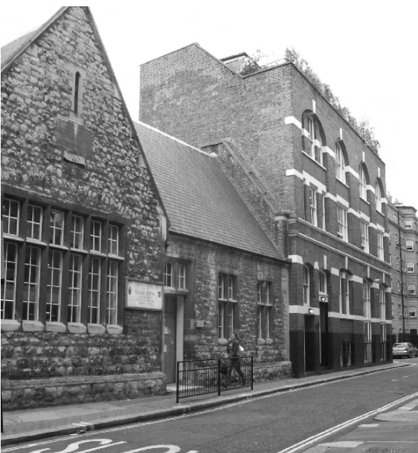
Figure 75: St Matthew's and Old Pye House's eastern facades on St Ann's Street
