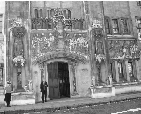
Figure 31: Middlesex Guildhall porch detailing
