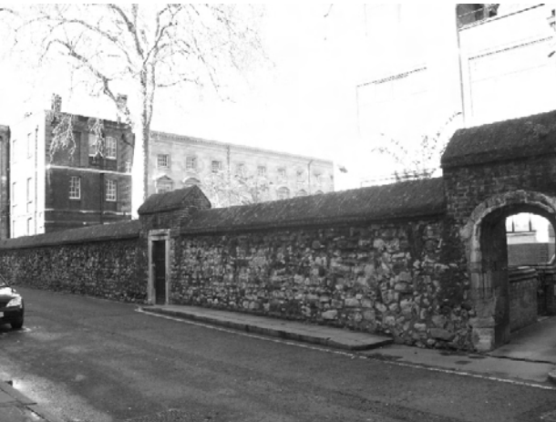
Figure 93: Medieval stone wall north of Great College Street marking southern boundary of Thorney Island and the Abbey Precinct with cast-iron railings between these. They are listed Grade II. Fronting the Abbey are more decorative Gothic railings. The central gate is painted in red, gold and black, with a lantern to either side (Figure 91). These date from 1882, possibly by W. D. Caroe. The same detail can be found to the railings to the rear of the Abbey.
