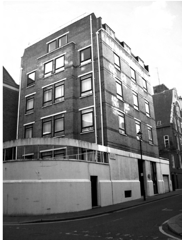
Figure 139: No. 2 Little Smith Street
