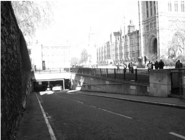
Figure 138: Abingdon Street car park entrance
