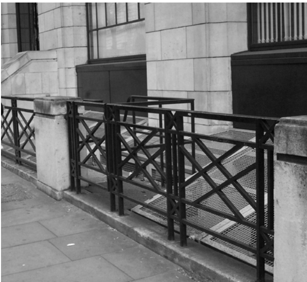
Figure 145: Modern replacement railings and grilles blocking basement lightwell to 10 Great George Street
