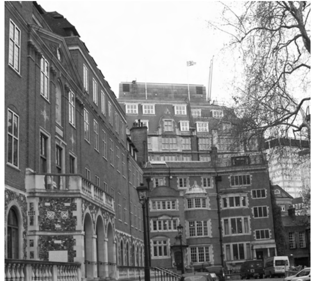
Figure 143: Looking from Dean's Yard, the roofs of 16 Great Smith Street forming the backdrop
