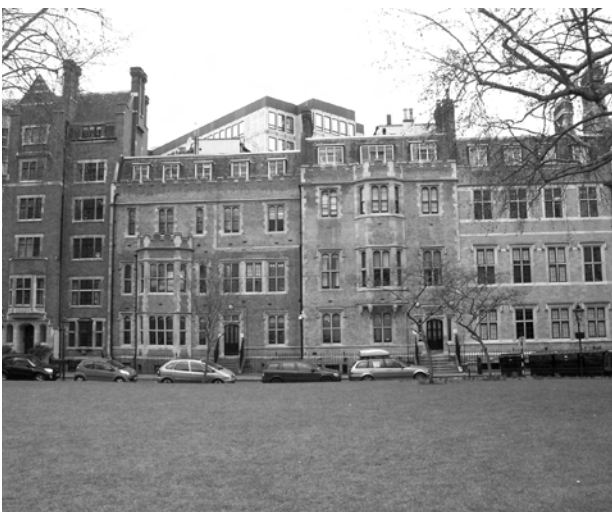
Figure 62: Former Queen Anne's Bounty Offices
