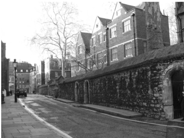
Figure 48: Stone wall defining southern boundary of Thorney Island
