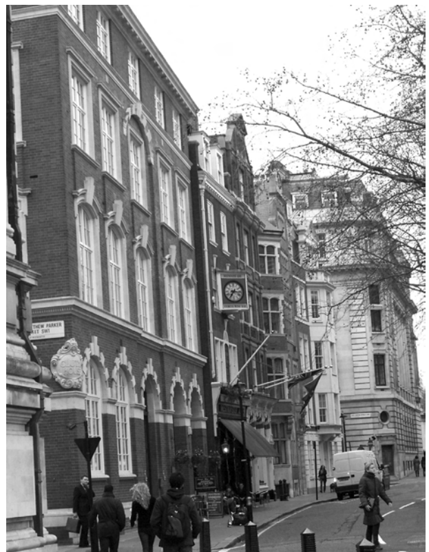
Figure 37: Nos. 8-10 Storey's Gate, with No. 10 (Clutha House) in the foreground and No. 9 (Westminster Arms) to the centre
