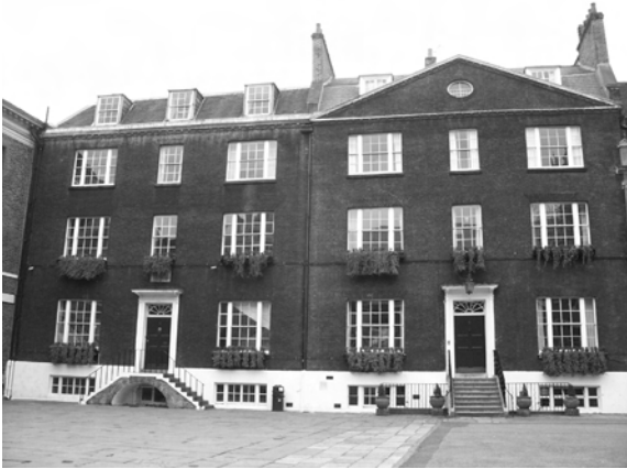
Figure 51: Nos. 2 and 3 Little Dean's Yard
