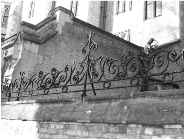
Figure 96: Wrought-iron railing panel, Dean's Yard
