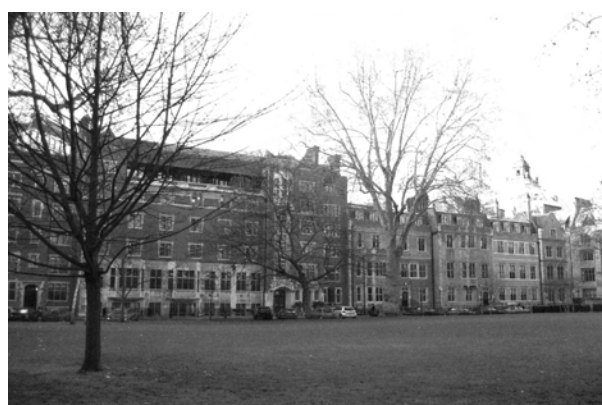
Figure 60: Western elevations to Dean's Yard
