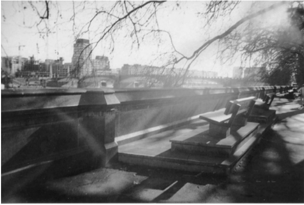
Figure 87: Embankment walls in Victoria Tower Gardens
