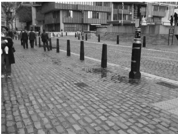
Figure 130: Granite setts of footways and carriageways of Storey's Gate
