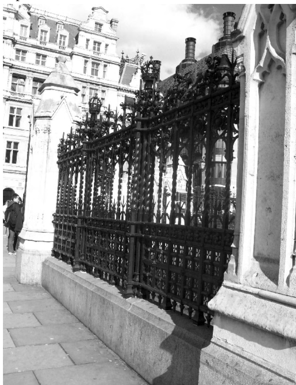
Figures 84-85: ( Above ) Railings to Cromwell Green Visitor Entrance (2007) by Architects Design Partnership. ( Below ) Houses of Parliament gates and railings (c.1869). Portland stone and cast iron. Gate piers with gablet-spire caps.
