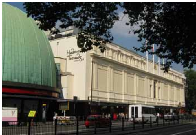
Figure 9: The front elevation of Madame Tussauds facing Marylebone Road.
