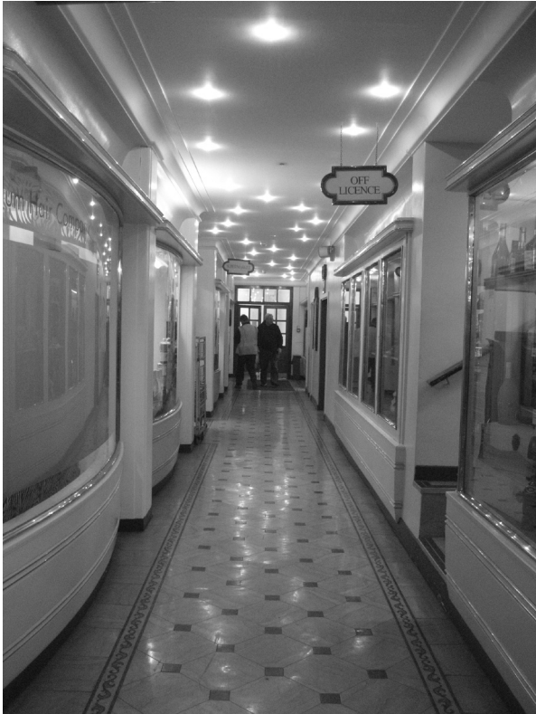
Figure 51: Shopfronts in Rodney House Shopping Arcade
