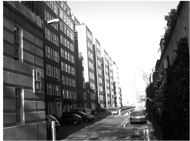
Figure 14: Eastern elevation of Dolphin Square
