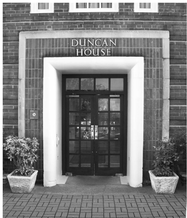
Figure 23: Entrance Porch, Duncan House
