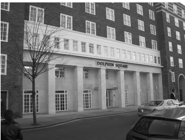
Figure 25: Chichester Street entrance
