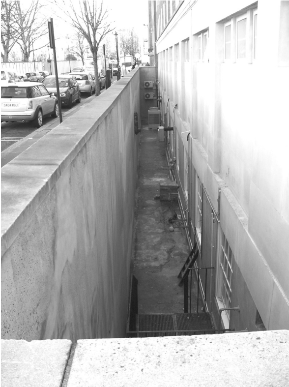
Figure 59: Lightwell off Chichester Street
