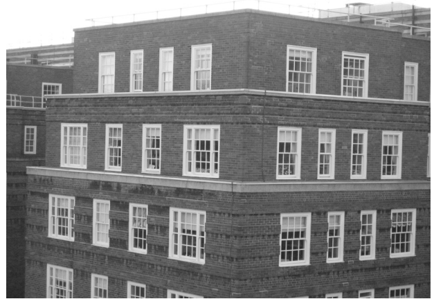
Figure 17: Stepped roof of internal projecting section
