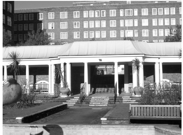
Figure 26: Rodney House's Pavilion frontage
