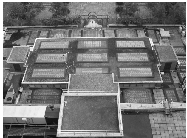
Figure 27: Roof of leisure centre located in Rodney House
