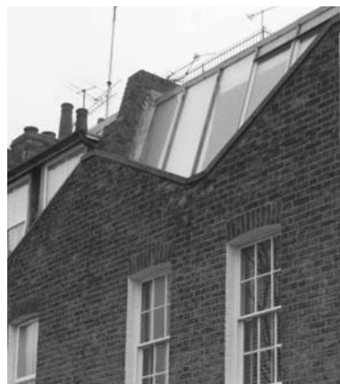
Figure 148: 96 Boston Place: example of roof extension which does not relate well to the historic roof form. There are many similar extensions within the conservation area
