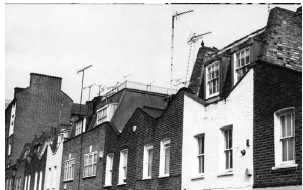
Figure 146: Poorly sited aerials and railings to roof of mews property
