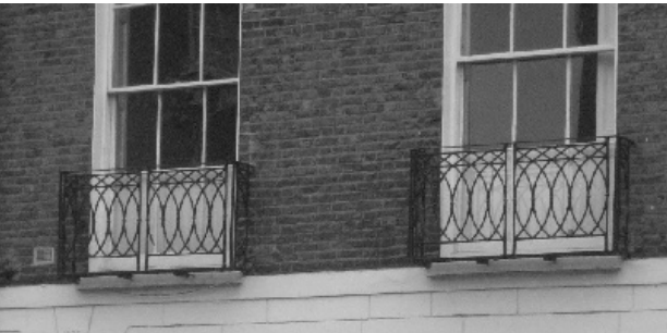
Figures 104-6: Examples of balcony detailing
