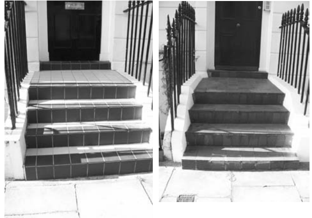
Figure 144 and 145: Examples of stone steps covered with modern tiles
