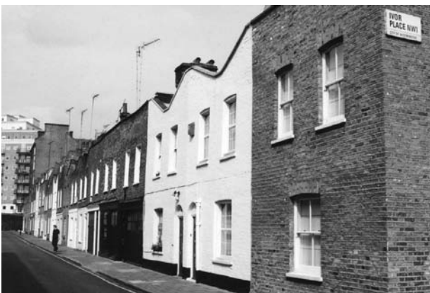
Figure 48: Nos. 64-100 Boston Place small scale 2-storey properties with original butterfly roof profile and sash windows
