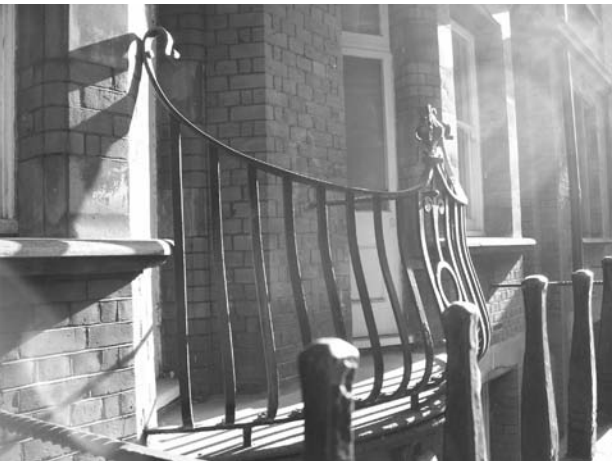
Figure 107: Wrought iron Art Nouveau balcony of Clarence Gate Mansion blocks
