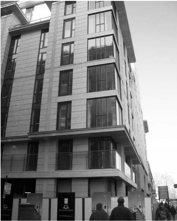
Figure 80: Abbey House development
