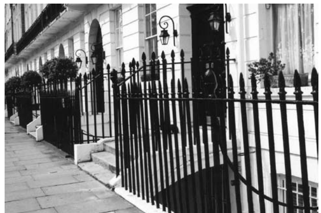
Figure 98: Spear-headed railings to Dorset Square properties
