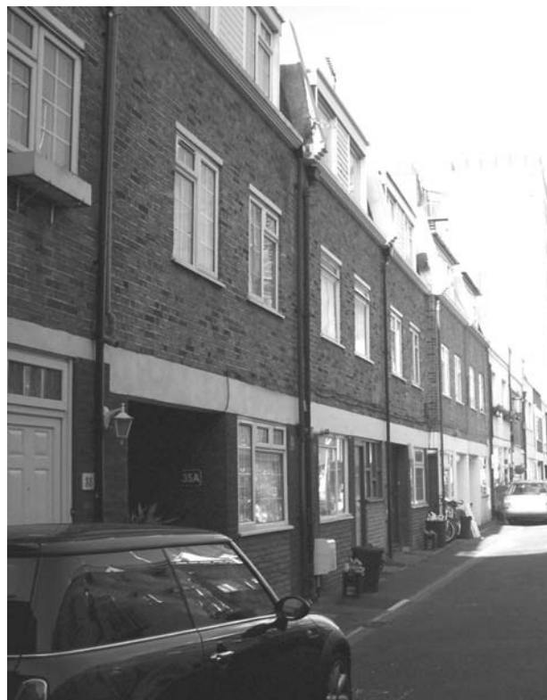
Figure 141: Replacement uPVC windows and doors in Huntsworth Mews
