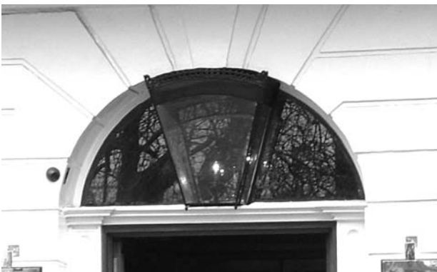
Figures 27-29: Different styles of decorative fanlights on Dorset Square, one incorporating a gas lamp holder
