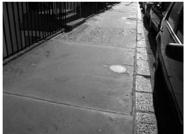
Figure 131: York Stone paving to Balcombe Street interspersed with original coal hole covers
