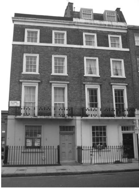
Figure 38: Nos. 62-64 Balcombe Street have undergone subsequent alteration
