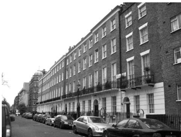
Figure 22 and 23: ( above ) Dorset Square western side; ( below ) northern side, with sheer storey extension disrupting the unity of the group
