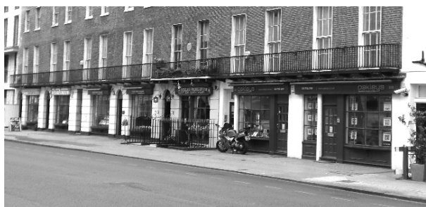
Figure 95: Shopfronts at 231-243 Baker Street
