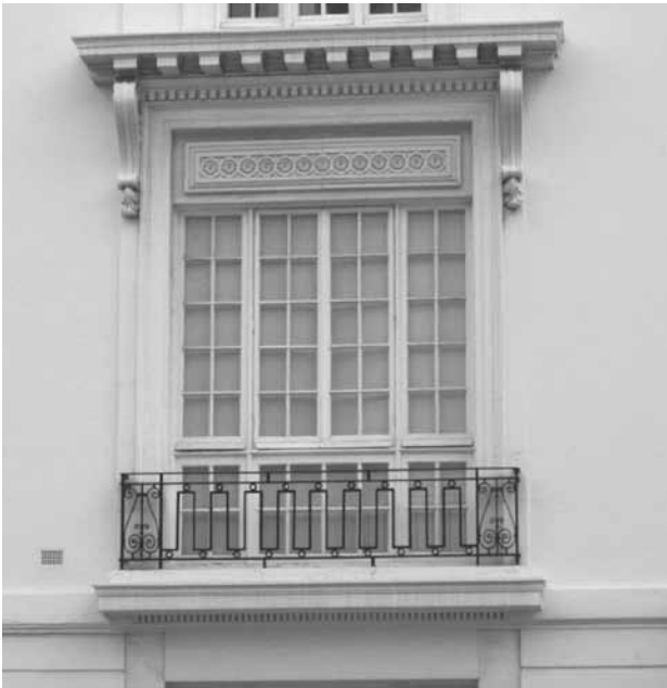
Figure 106: (above) unusual windows topped with frieze below lintel with dentils and supported on decorative consoles, Upper Belgrave Street.
