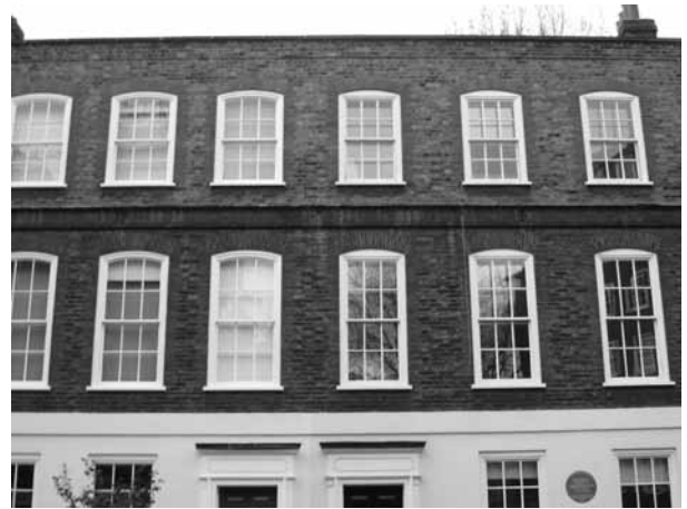
Figure 109: Flush sash windows to early Georgian terrace, Ebury Street
