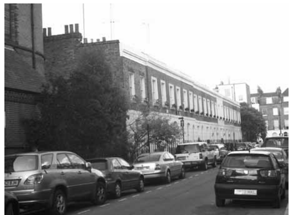
Figure 63: Small-scale terraces to Graham Terrace with a highly consistent character; most of the houses are 2 storeys above a semi-basement.
