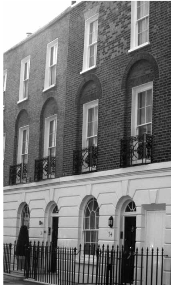
Figure 52: (above) First floor windows set in round headed blind reveals on Eaton Terrace.
