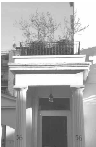
Figures 227 & 228: (top) Eaton Square portico with stucco in poor condition and replacement of original stone steps with tiling; (left) loss of original balustrade to portico.
