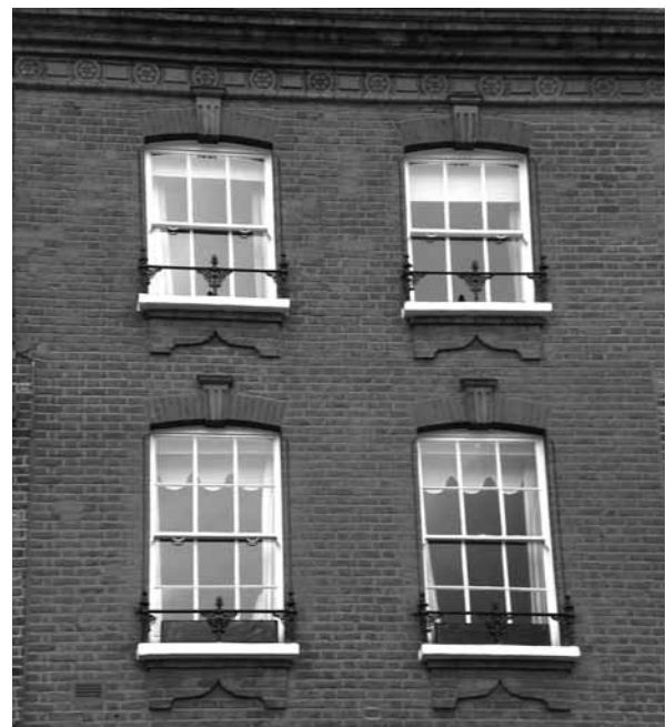
Figure 126: Typical Victorian house in red brick, with decorative brickwork to the eaves, brick arches with central keystone, brick aprons below windows and pot retainers.
