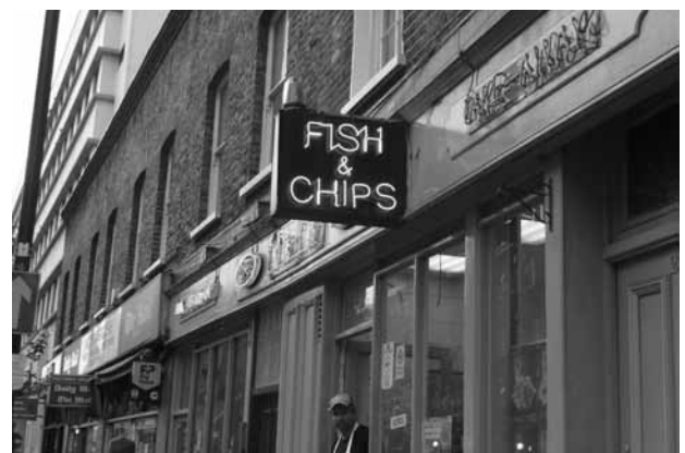
Figures 233 & 234: Poor quality shopfronts on Elizabeth Street including projecting boxes and illuminated signage.
