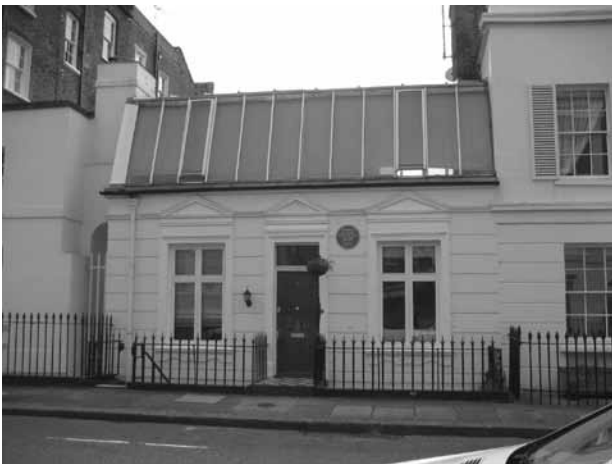
Figure 231: Roof alteration at No.1A Caroline Terrace.
