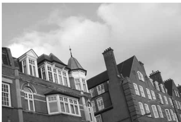
Figure 130: Late Victorian roofscape
