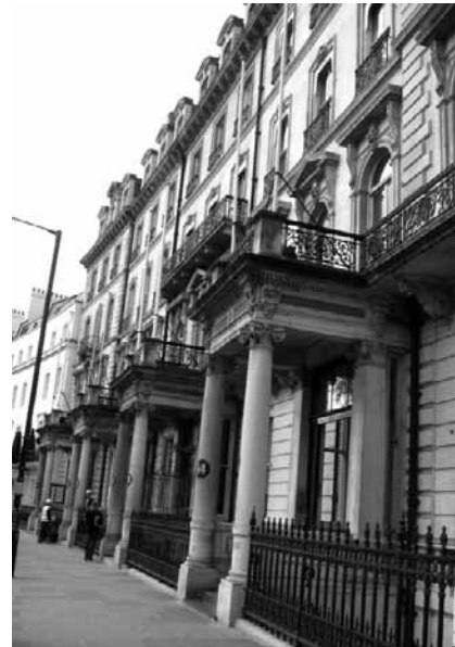
Figure 85: (left) Victorian townhouses on Grosvenor Crescent.
