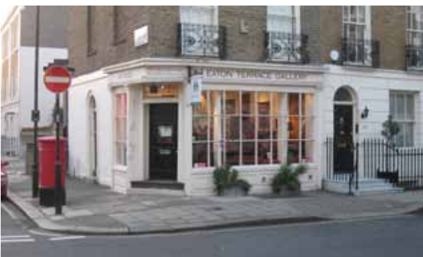
No. 40 Eaton Terrace
