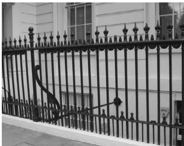
Figure 144: Belgrave Square has a distinctive pattern of railings with spearhead finials, semi-circular 'swag' ornamentation below the rail and dog rail to base.
