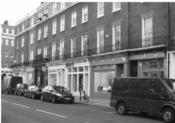
Figure 140: Small shopfronts on Elizabeth Street
