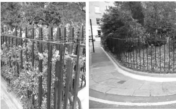
(Figure 156). Many of the small shops are also set back behind basement lightwells fronted by a variety of attractive railings designs.
