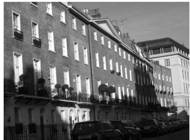
Figure 57: (above) Late Georgian terraces on Wilton Street.
