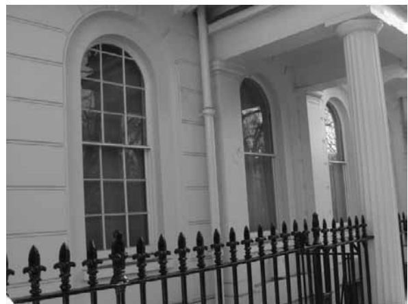
Figure 217-218: Loss of original glazing patterns to windows on Eaton Square and Eaton Place.
