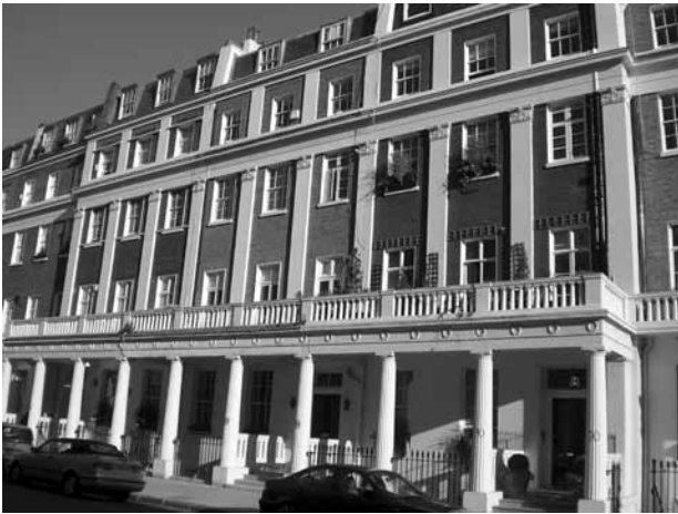
Figure 23: Giant Corinthian pilasters used to define the centre of the terrace on Eaton Place. Colonnade to entrance with fluted Doric columns and balustraded balcony above.
