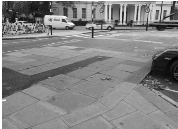
Figure 245: ( top ) patching of paving on Belgrave Square; Figure 246 ( below ) asphalt surfacing to pavements on Eaton Square is not in keeping with the character of the area and Figure 247: below, loss of setts within the mews significantly alters the character.
