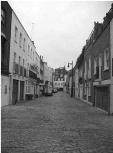
Figure 198: Historic Street Surfacing in mews.
