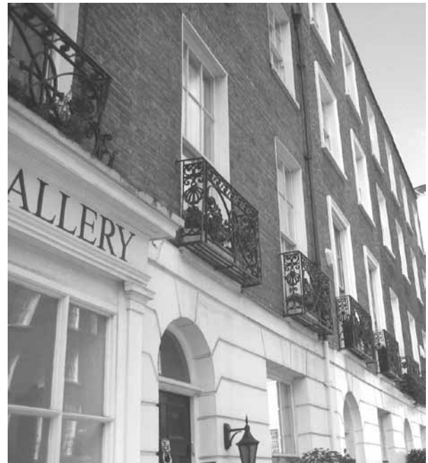
Figure 161: ( above ) Balconettes to Eaton Terrace first floor.
