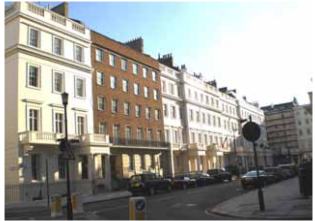
Figure 98: Red brick 1950s infill at no. 86 Eaton Place contrasts with the stucco terraces
