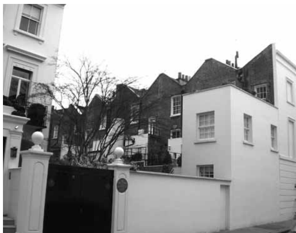
Figure 131: Pattern of butterfly roofs visible at the rear of South Eaton Place from Gerald Street
