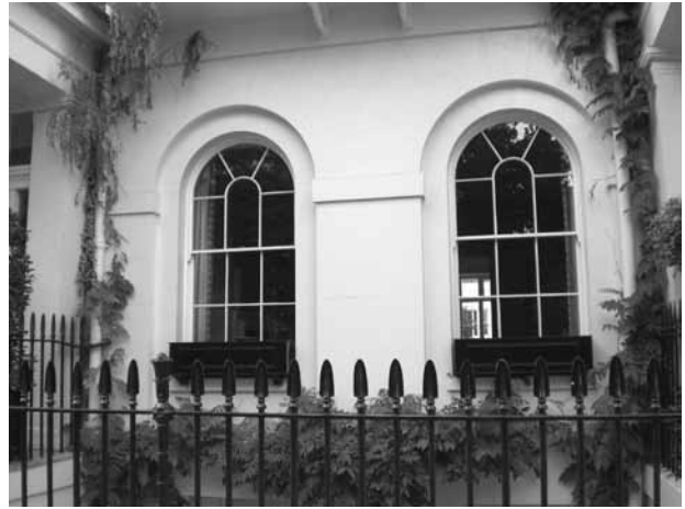
Figure 103: ( above ), Arched sash windows are common on the ground floor of Belgravia terraced houses. Figure 104: ( below ), Sash window with side lights on Chester Square
