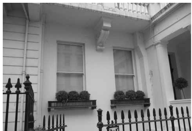
Figure 217-218: Loss of original glazing patterns to windows on Eaton Square and Eaton Place.
