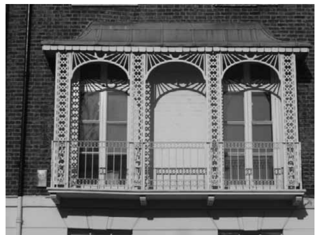
Figure 162: ( above ) Cast iron balcony to Eaton Terrace.
