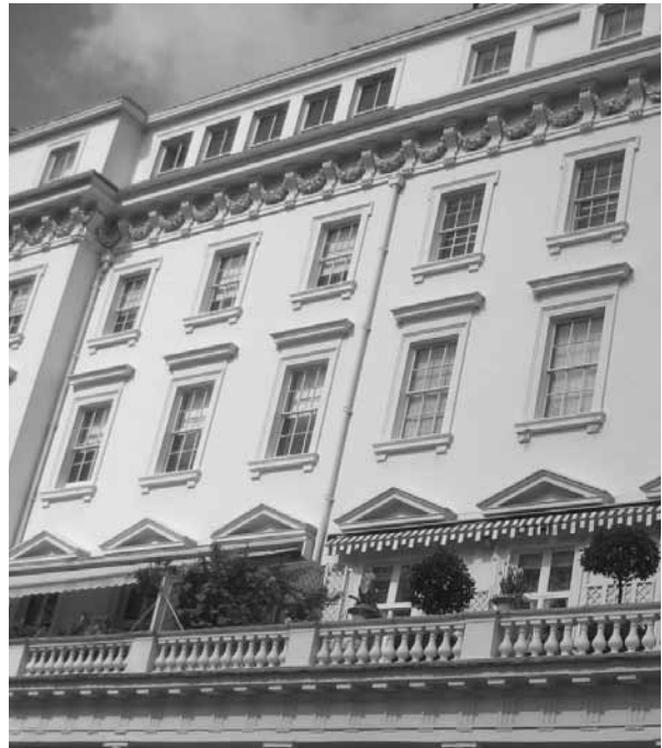
Figure 32: Italianate detail to Eaton Square (c.1850), including bottle balustraded balcony, pedimented windows to first floor and elaborate moulded cornice below the attic storey decorated with dentils and swags.
