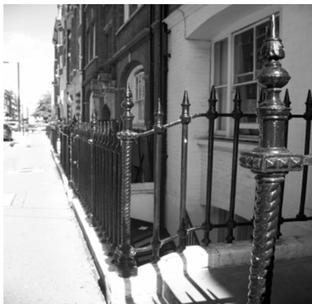
Figure 77: Heavily moulded cast iron railings at No. 114 Great Titchfield Street
