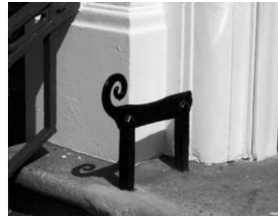
Figure 85: Wrought iron boot scraper
