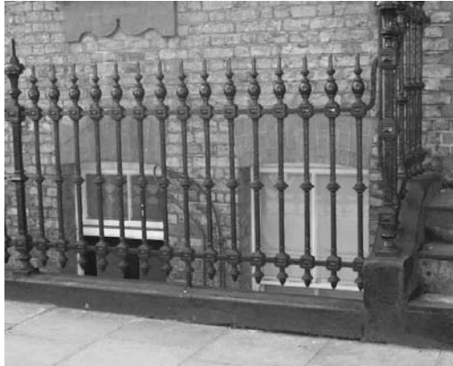
Figure 79: Heavy cast iron railings along Gosfield Street
