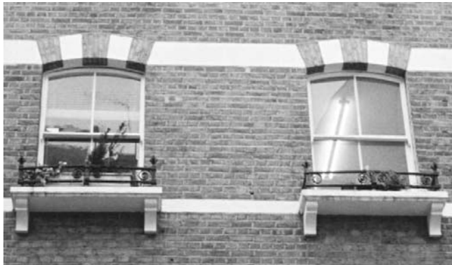
Figure 84: Decorative cast iron pot retainers along Wells Street
