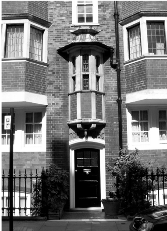
Figure 27: Entrance to the Tower House, Candover Street. The simple arched timber door has glazed panels and an oriel window above
