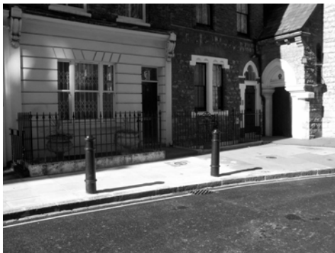
Figure 91: Cast iron ‘Cannon’ style Bollards on Ogle Street, produced to an early 19 th century pattern
