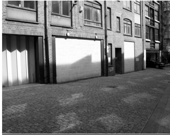
Figure 109: Bourlet Close – Doors blocked with breeze blocks
