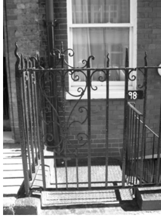
Figure 74: 98 Great Titchfield Street
