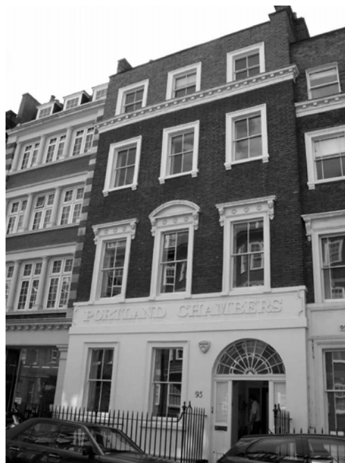
Figure 17: 93 Great Titchfield Street
