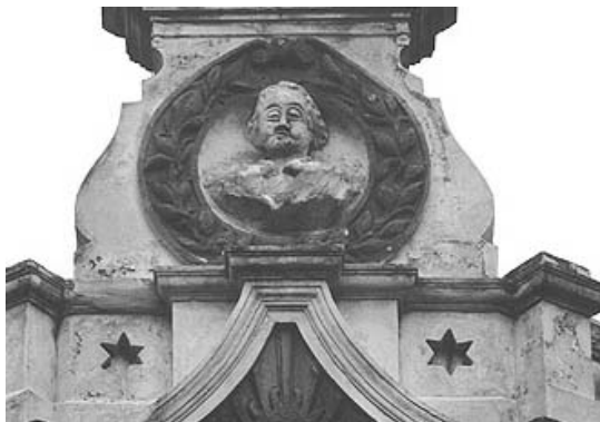
Figure 69: Former Earl Russell Public House, 24 Mortimer Street
