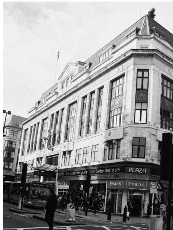
Figure 38: The Plaza, formerly Bourne and Hollingsworth
