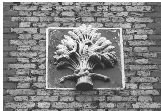
Figure 70: Former Wheatsheaf Public House, 71 Great Titchfield Street
