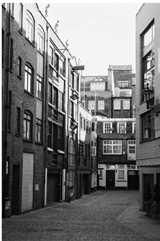
Figure 30: Bourtlet Close. Converted 19 th century warehouse buildings which although converted have retained original loading bays and hoists
