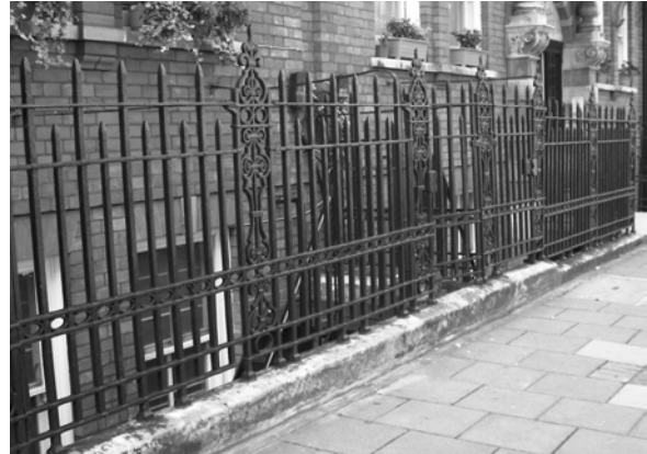
Figure 80: Elaborate cast iron railings outside Selworthy House, Great Titchfield Street
