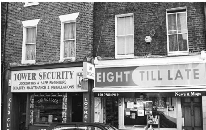
Figure 107: Oversized signage of poor quality design and materials on New Cavendish Street
