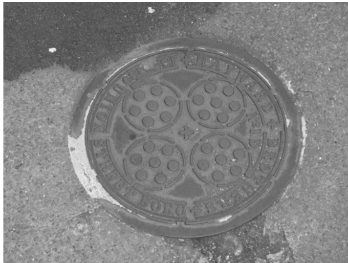
Figure 101: Coal Hole Cover
