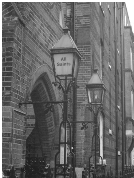
Figure 87: Listed lampstandards and railings, Margaret Street
