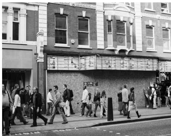
Figure 105: Vacant premises with stripped fascia and boarded front
