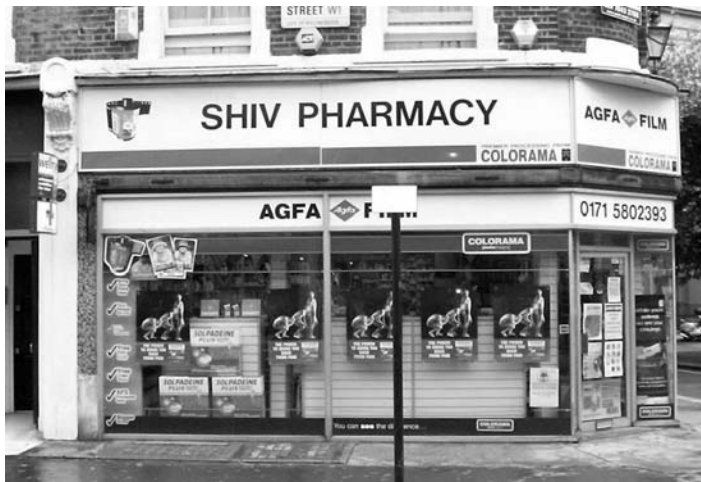
Figure 106: 70 Great Titchfield Street, a glass and metal front and large plastic fascia board have been unsympathetically inserted into the original surround
