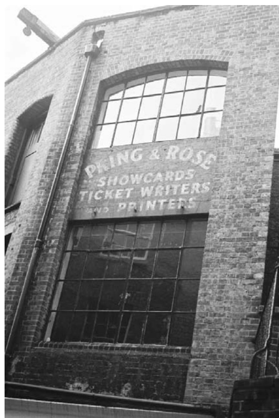
Figure 31: Warehouse, St Margaret's Passage. Steel Critall windows in large arched openings, characteristic of warehouse architecture
