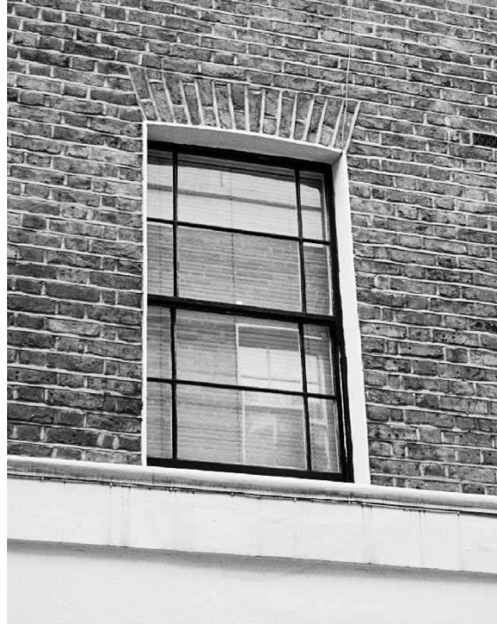
Figure 15: Window: Middleton Buildings
