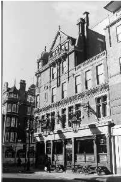
Figure 89: Great Titchfield Street
