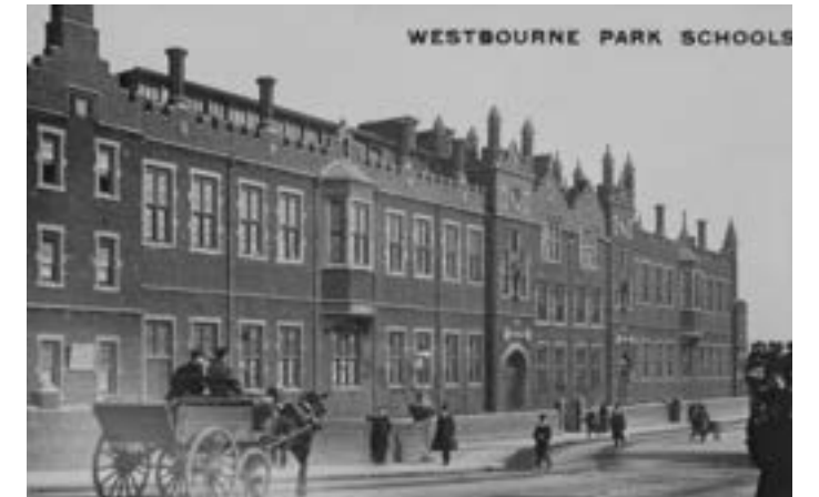
Figure 3.4 Westbourne Park School, built in 1861, occupied the Site before it was demolished Source: Layers of London
