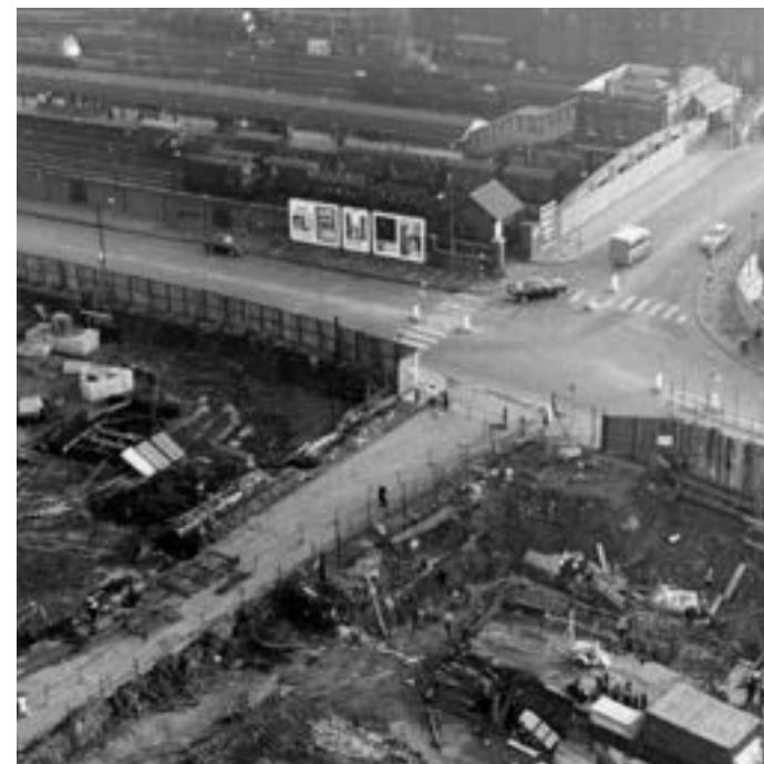
Figure 5.3 Construction of the Westway adjacent to the Site
