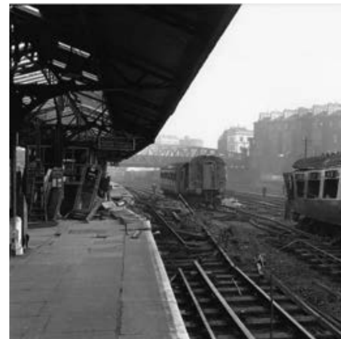
Figure 5.4 WW2 bomb damage at Royal Oak Station
