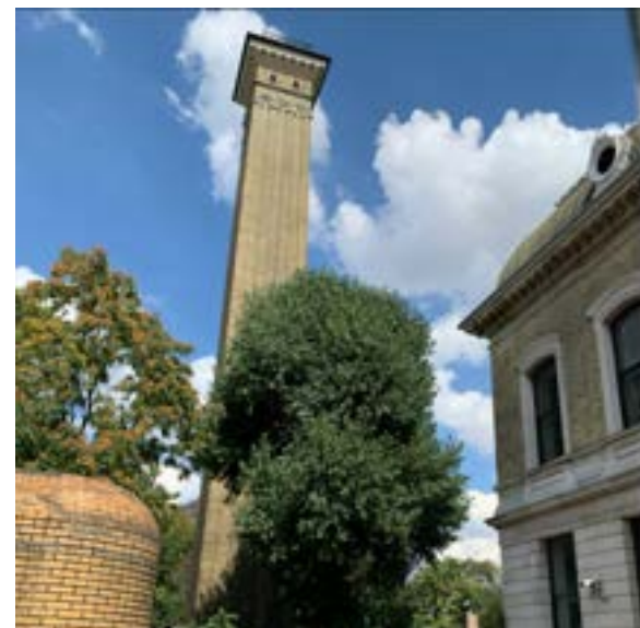
Figure 4.32 Site photograph showing the Water Pumping Tower and the listed building
