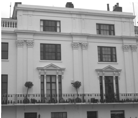
Figure 22: 5 & 6 Victoria Square. First floor windows to the centre blocks and each end of the terraces are of tripartite design. The French windows are capped by a triangular pediment supported on consoles with moulded female heads.
