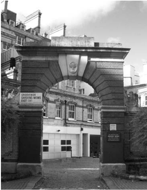
Figure 20: The grand brick and stone arched entrance to Grosvenor Gardens Mews East
