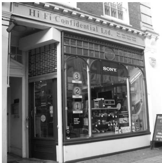
Figure 46: No. 32 Buckingham Palace Road This shopfront is typical of the group. The display window is subdivided by delicate curved glazing bars and there is multi-pane glazing to the transom light. The doorway is recessed and the fascia set below a projecting dentil cornice. A roller shutter box forms an intrusive addition above the door.
