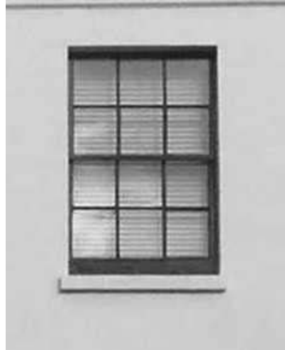
Figure 28: Standard 6-over-6 sash
