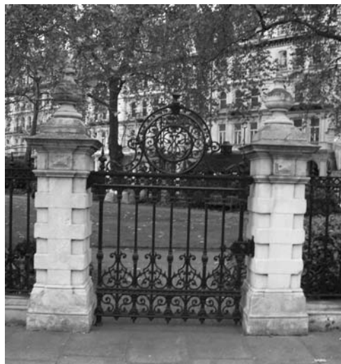
Figure 54: Gate Piers and Gates: Grosvenor Gardens North
