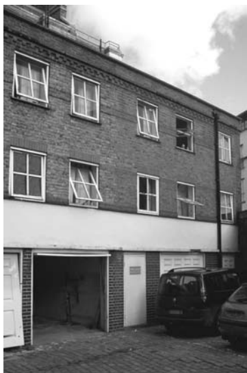
Figure 71: Nos. 13a & 15a Grosvenor Gardens Mews East – poor quality replacement to original architecture, especially ground floor treatment.
