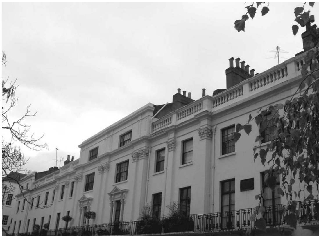
Figure 37: The Roofscape to the Eastern side of Victoria Square
