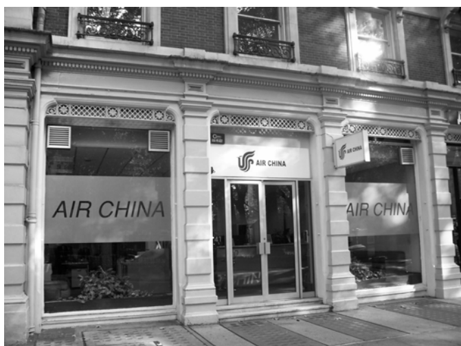
Figure 44: Although a new frame has been inserted, 41 Grosvenor Gardens is set within its original surround and retains its arches and decorative grilles.
