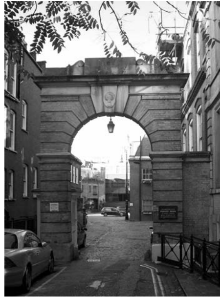
Figure 21: The other large archway to Grosvenor Gardens Mews North, with the Grosvenor Family emblem in the central key-stone
