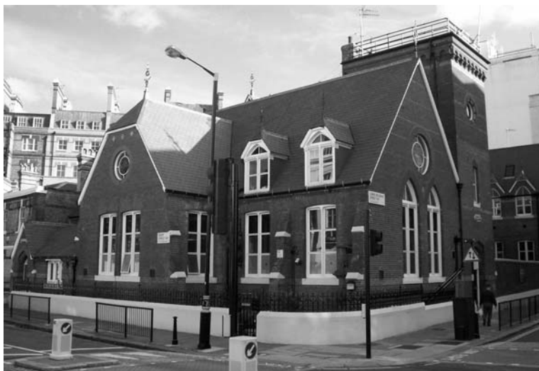
Figure 33: St. Peter's School, Ebury Street
