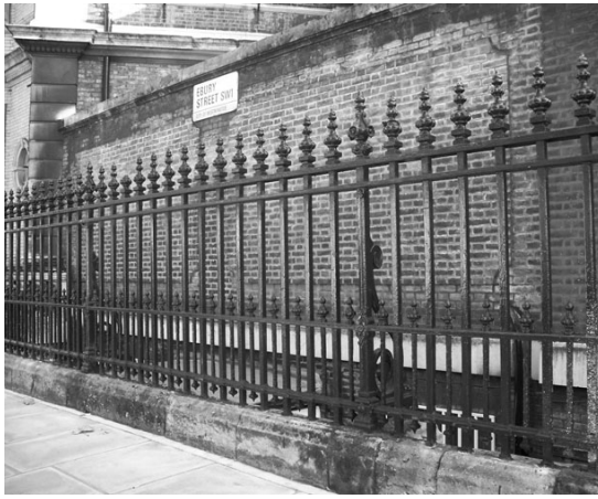
Figure 58: Robust Victorian railings on Ebury Street
