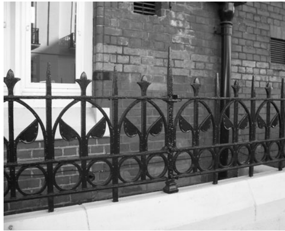
Figure 59: Railings to St Peters School on Ebury street
