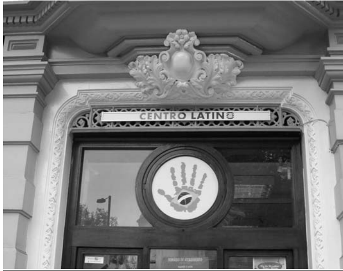
Figure 45: Detail of decorative mouldings to the arch and cartouche at 37 Grosvenor Gardens.
