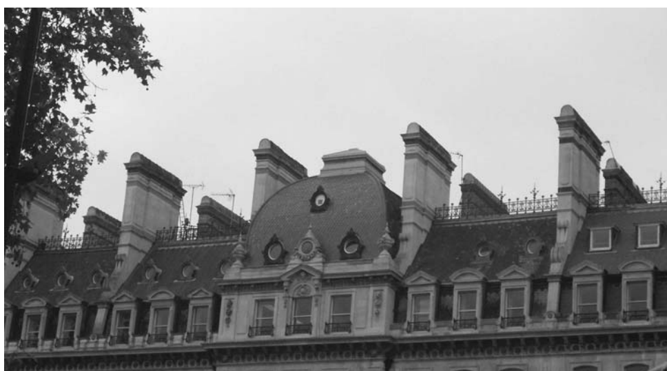
Figure 35: Roofscape. 36-50 Grosvenor Gardens
