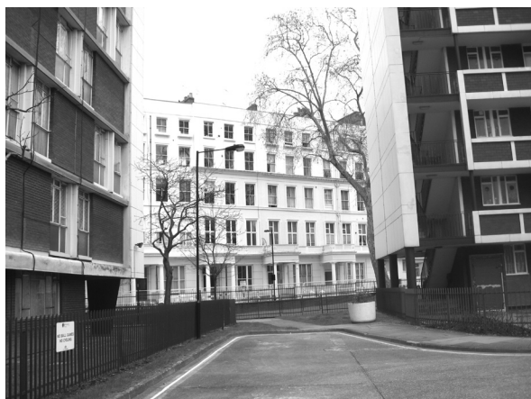
Figure 41: Glimpse of Victorian housing surrounding the estate, framed by the postwar blocks
