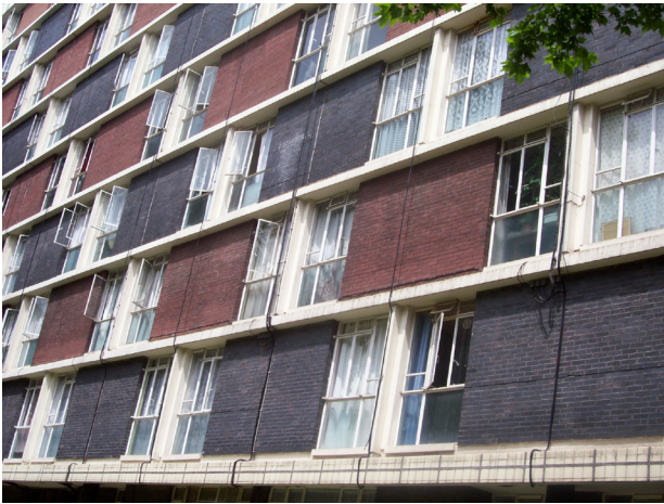
Figure 22: Checker board pattern of windows and red and grey brick panels on 10-storey block reverse elevation
