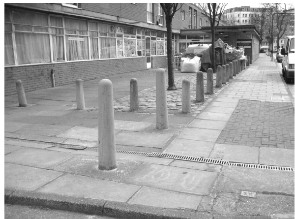
Figure 50: Concrete bollards and hard landscaping to the front of Pickering House
