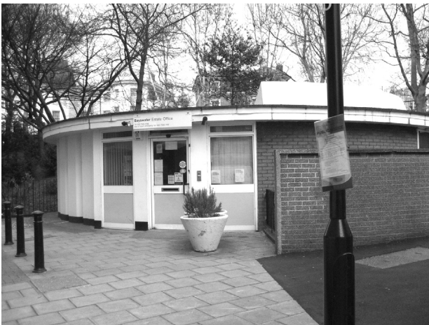
Figure 36: Original Laundry block
