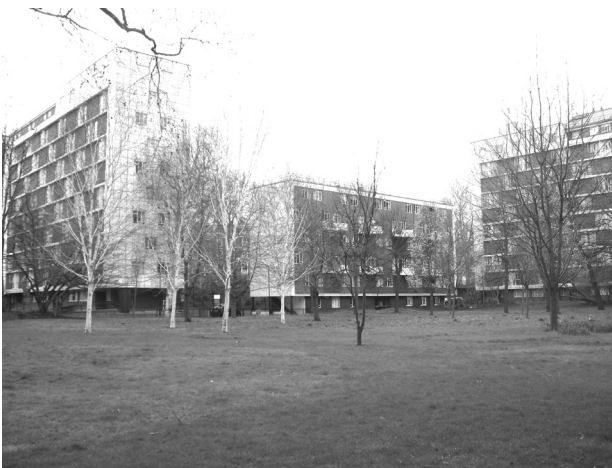
Figure 15: The arrangement of different types of blocks maximises the sense of open space within the estate
