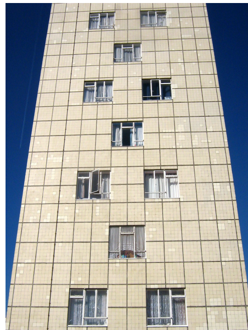
Figure 21: Gable end of 10-storey block
