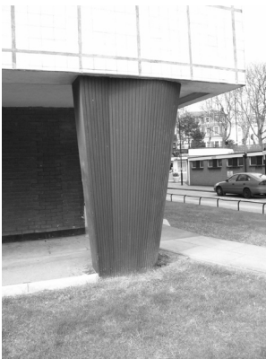
Figure 23: Fluted concrete columns
