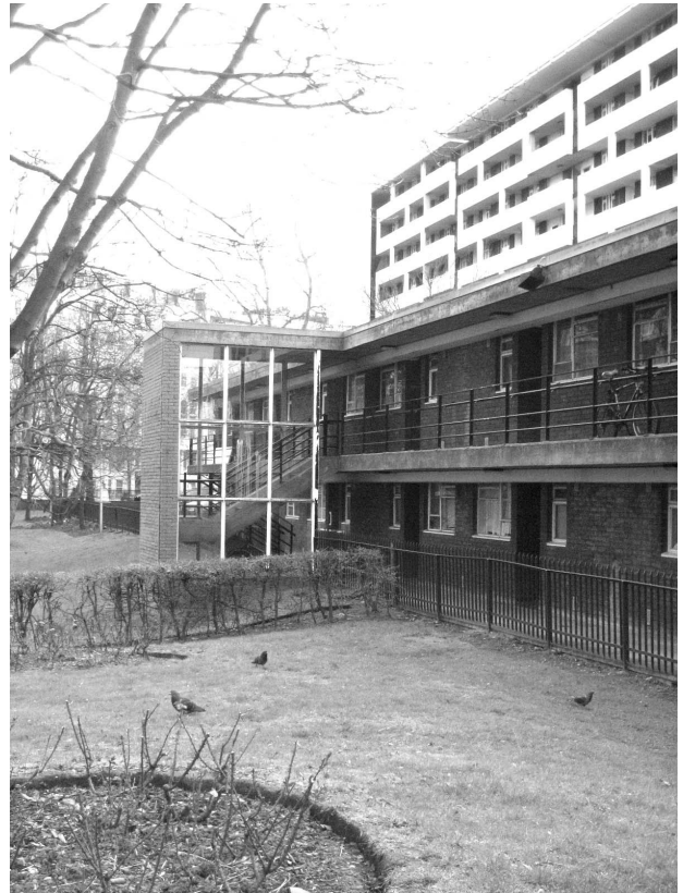
Figure 32: Glazed stairway to rear of Pickering House
