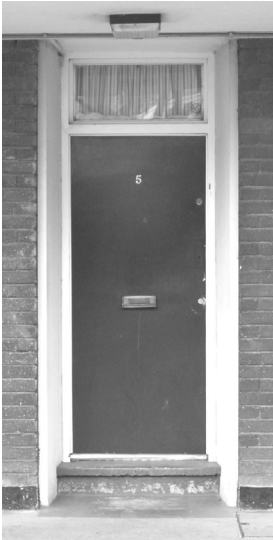
Figure 31: Original flush timber door with small aperture letterbox
