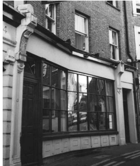
Figure 41: Canted wooden shopfront at No. 1 Hanway Place
