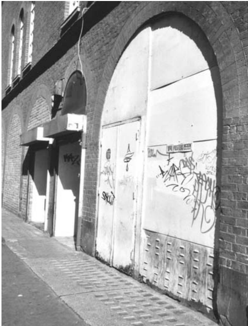
Figure 44: Projecting shutter casements and boarded up entrances have a deadening effect and are ideal for graffiti
