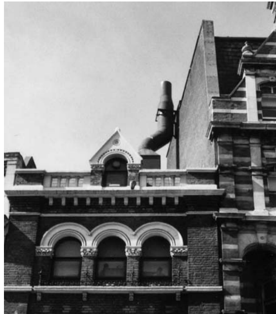
Figure 43: Little effort has been made to minimise the impact this ventilation flue has on the buildings it is attached to or on the local street scene
