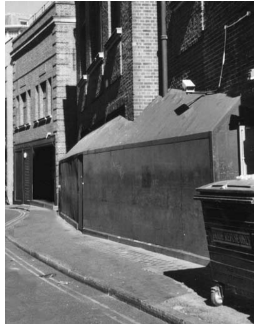
Figure 45: The large metal casing at the rear of Virgin Megastore is damaging the character of Hanway Street
