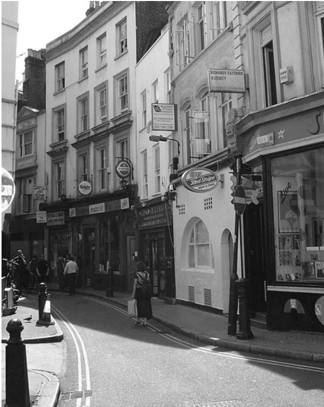
Figure 21: Hanway Street's west side, with narrow frontages, canted to follow the street pattern
