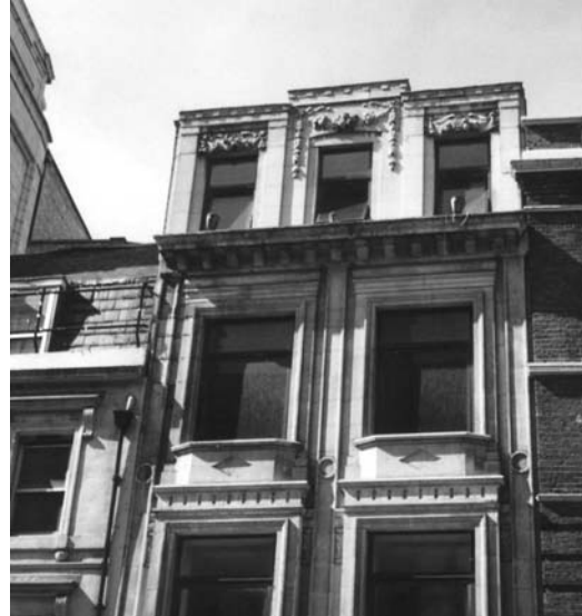
Figure 24: No. 10 Oxford Street
