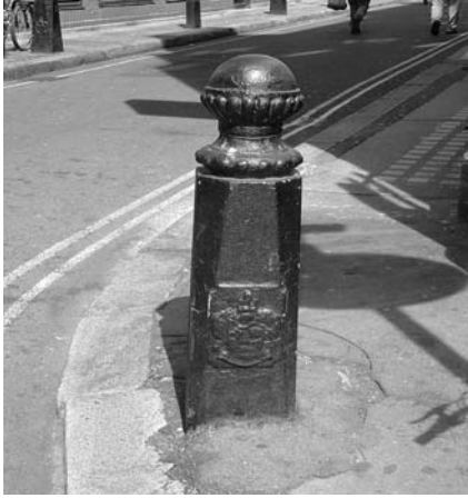
Figure 35: The historic St Marylebone bollard today, the numerous layers of paint have obscured the coat of arms
