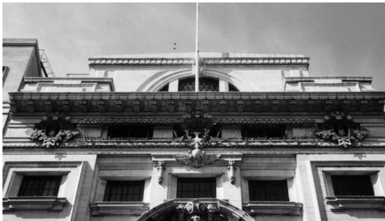
Figure 25: No.14-16 Oxford Street
