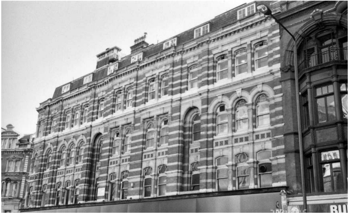
Figure 28: No. 4 Oxford Street, the vast building with its horizontal emphasis and polychrome brickwork makes it a prominent feature at one of London's busiest junctions
