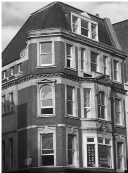
Figure 16: No. 48 Oxford Street
