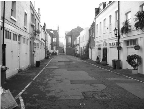
Figure 140: Devonshire Mews South. The loss of setts from the Mews areas detracts from their intimate character
