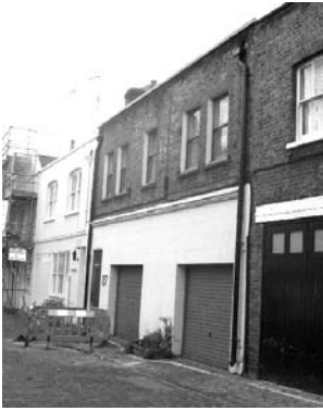
Figure 135: 27 Weymouth mews has blockwork to the ground floor with metal up and over garage doors
