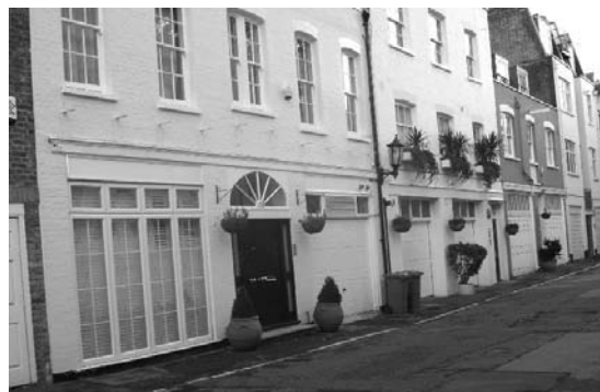
Figure 134: 103-105 Devonshire Mews. Ground floor openings have full height uPVC windows and metal up and over garage doors
