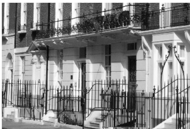
Figure 94: Original Georgian railings along Harley Street
