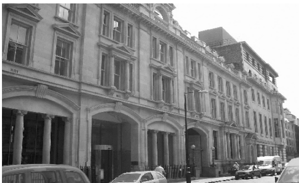
Figure 55: Kingsley House, Wimpole Street
