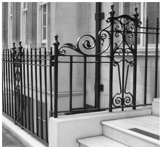
Figure 101: Edwardian 'Arts & Crafts' style railings in wrought iron with twisted leaves at 39 Queen Anne Street
