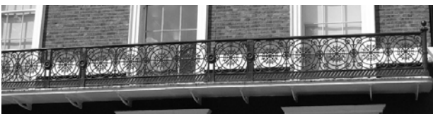
Figure 104: An elaborate 'spider's web' balcony of c. 1800 at 17 Cavendish Square
