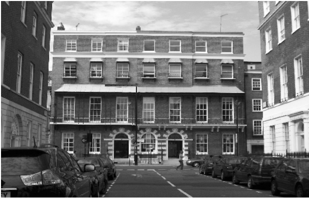
Figure 20: 61-63 New Cavendish Street
