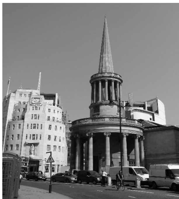
Figure 79: All Soul's Langham Place with Broadcasting House behind
