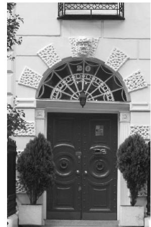
Figure 24: Coade stone door surround with central figurehead key stone. Surrounds of this type are found throughout the conservation area, particularly on Harley Street
