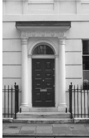
Figure 26: Eight panelled door in semi-circular arched opening. Stucco doorcase has engaged Corinthian columns supporting frieze with dentil cornice
