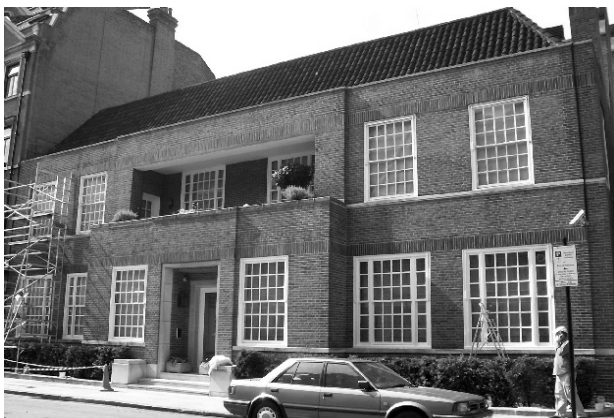
Figure 64: No. 22 Weymouth Street
