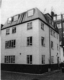
Figure 136: 11 Cross Keys Close unsympathetic replacement windows, smooth render and scale of this block does not relate well to adjoining buildings.
