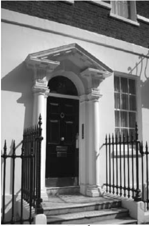
Figure 25: Eight panelled door in arched and slightly recessed opening. Doorcase with open pediment supported by Ionic pilasters
