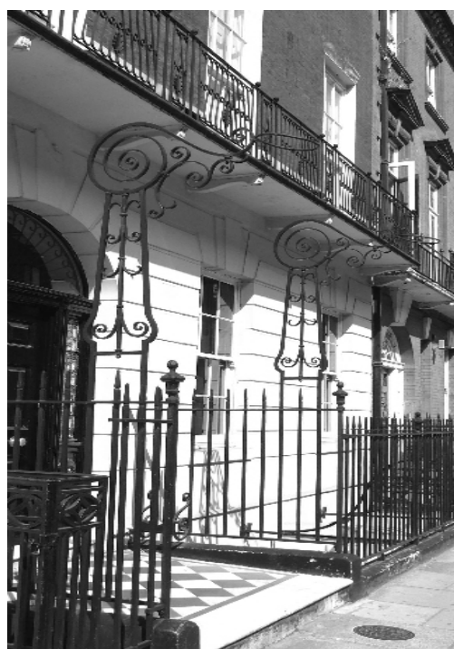
Figure 96: Cast iron lampholders at 21 Harley Street
