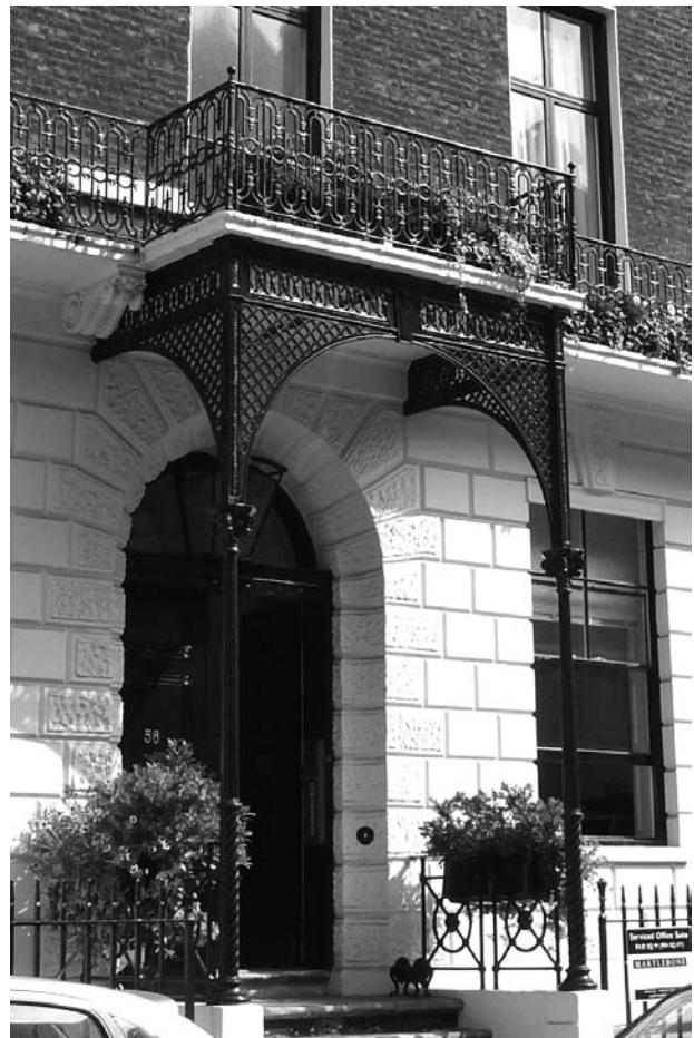
Figure 106: An early to mid 19th century cast iron porch and balcony added to a mid 18th century building
