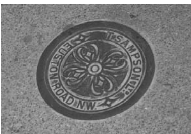
Figure 129: Coal Hole Cover
