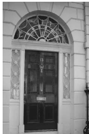
Figure 23: 13 Devonshire Place - a typical panelled door in Venetian timber door surround, with intricately detailed Adam style fanlight and side lights
