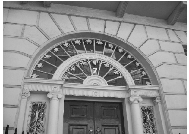
Figure 28: No. 7 Mansfield Street. An Adam fanlight with two rings, divided by timber architrave
