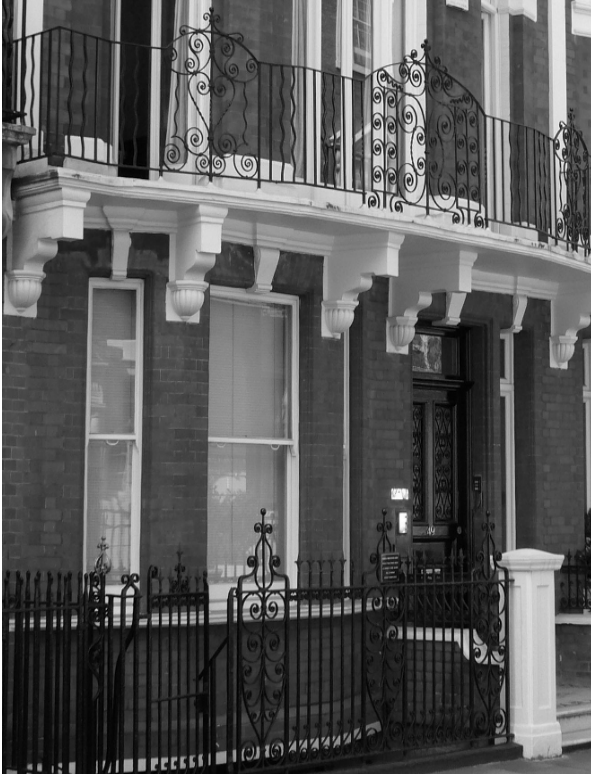
Figure 102: Elaborate railings and delicate first floor balcony at 49 Queen Anne Street
