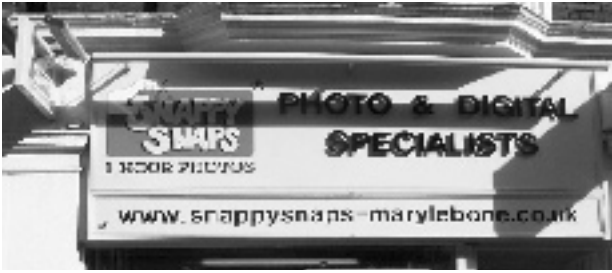
Figure 139: Oversize Signage, which does not relate to the shopfront frame, trough lighting and projecting signage
