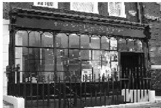
Figure 89: An attractive individual shopfront at no. 20 Welbeck Street. Set back behind railings with a multi-paned display window and slender pilasters supporting delicate console brackets.
