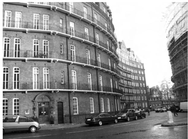
Figure 49: Rear blocks to Albert Hall Mansions
