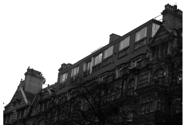
Figure 133: Roof extension to Park Mansions, Albert Gate
