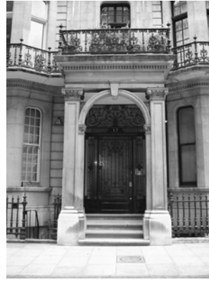
Figure 26: Porch detail, Ennismore Gardens
