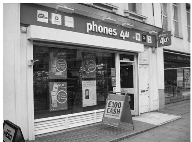
Figure 136: No.122 Brompton Road. Poorly detailed shopfront with projecting lights, internally lit box sign and shutter box creating visual clutter
