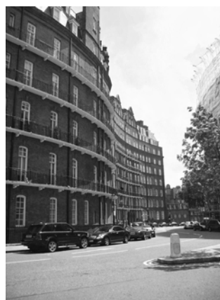
Figure 13: The curves and slope of the streets leading from Kensington Gore down past Albert Hall Mansions are an important part of the area's character
