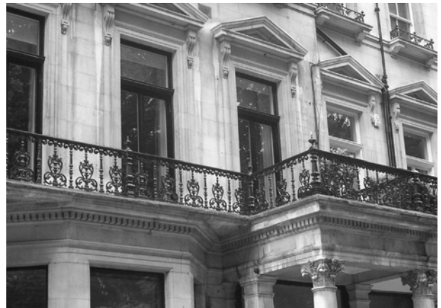
Figure 101: Decorative balcony detail to Ennismore Gardens, with matching pot retainers to upper floors
