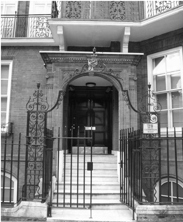
Figure 99: Delicate wrought iron railings to No. 29 Exhibition Road
