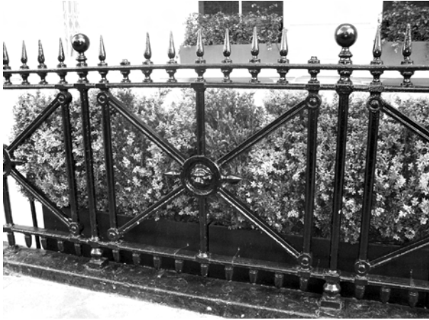
Figure 94: Railing detail in Rutland Gate
