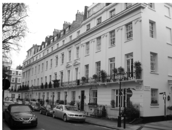
Figure 23: Montpelier Square, south side
