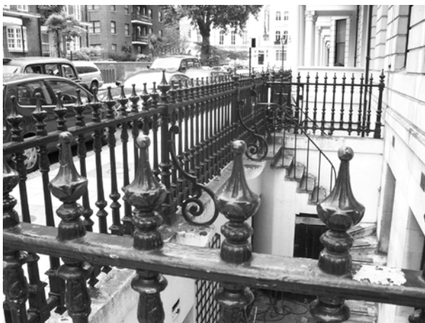
Figure 95: Railings at Prince's Gate
