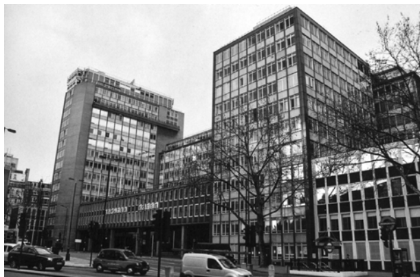
Figure 8: Bowater House prior to demolition
