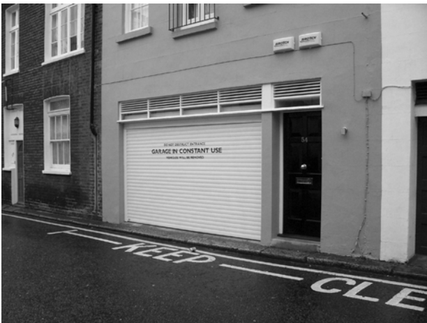
Figure 132: Garage door, Montpelier Walk
