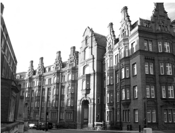
Figure 51: Queen Alexandra's House
