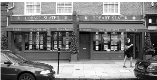
Figure 86: Nos. 6 & 8 Montpelier Street. Traditionally detailed shopfronts with stallriser, subdivided windows, pilasters and fascia
