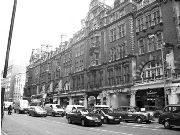
Figure 11: Mansion block on Knightsbridge, in the Albert Gate Conservation Area
