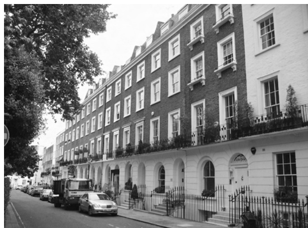
Figure 22: Montpelier Square, north side several different designs. Most window openings have stucco surrounds, some with pediments above. A simple moulded cornice runs the length of the terraces at parapet level, below recent roof extensions.
