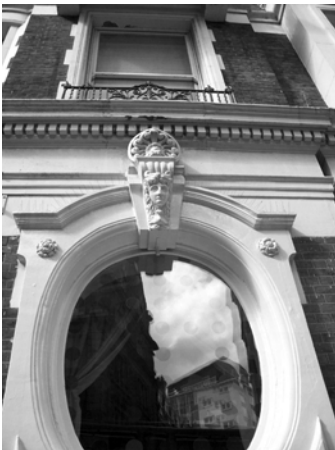
Figure 61: Window detail, Wellington Court
