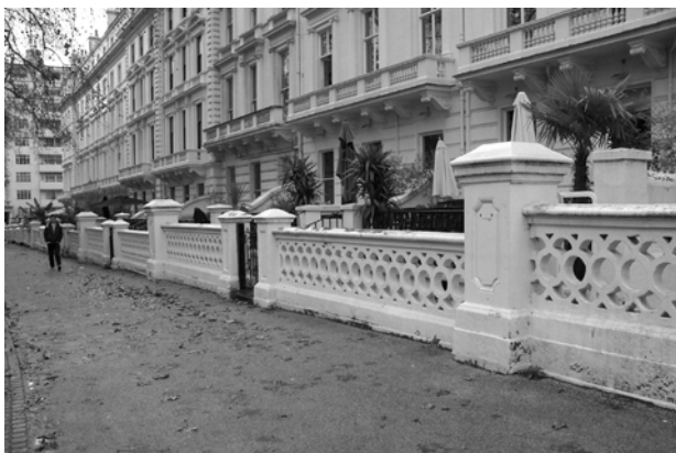
Figure 96: Stucco boundary wall at Prince's Gardens
