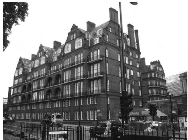
Figure 48: Albert Hall Mansions, front view
