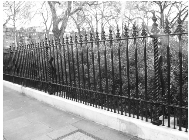
Figure 97: New replica railings to Prince's Gardens
