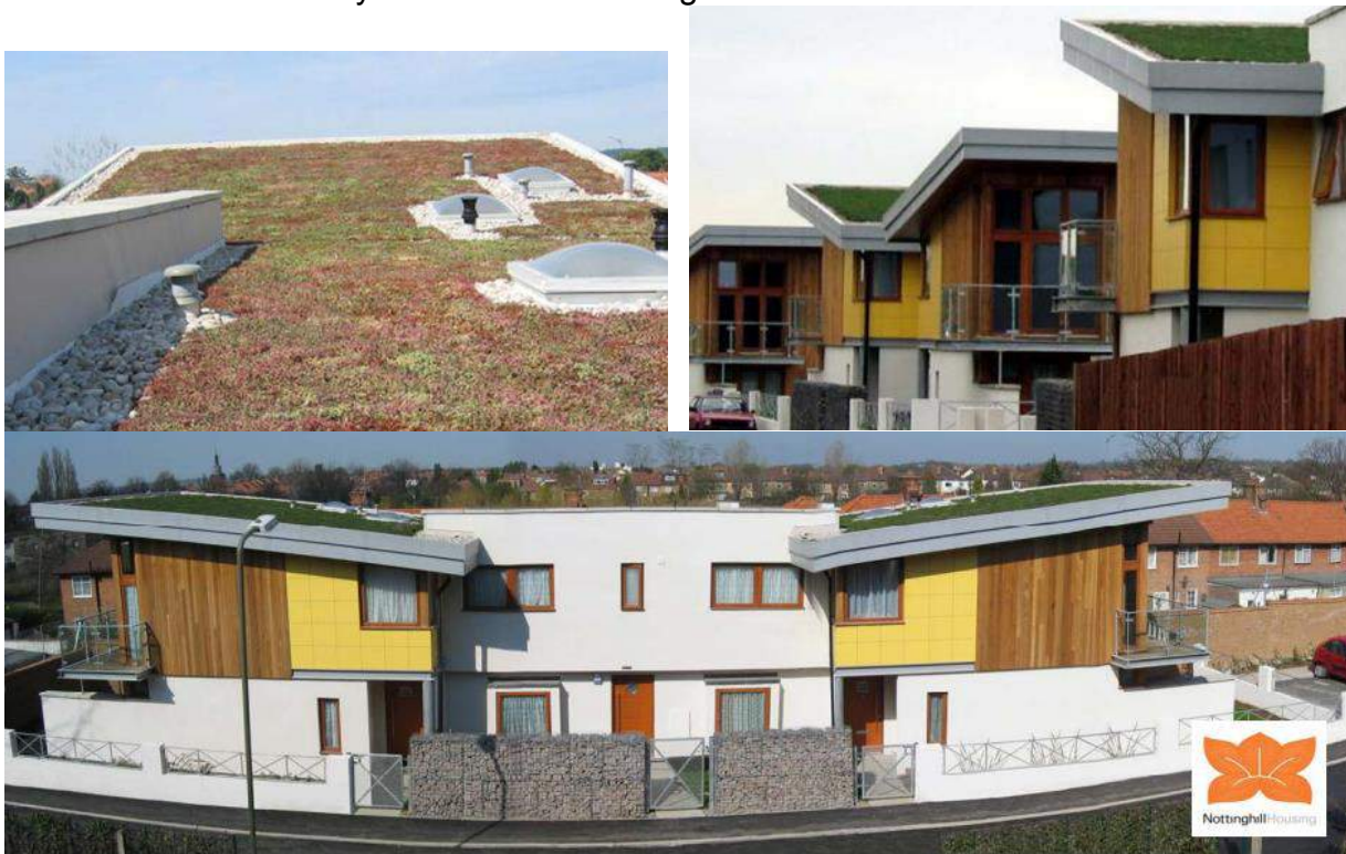
Figure 23, 24, 25: Photos of Gold Lane Social housing Project
