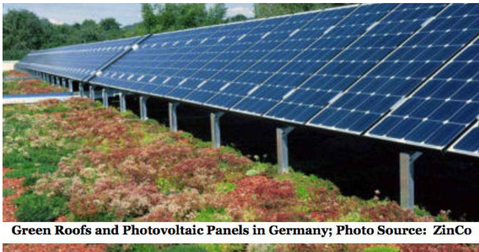
Figure 12. Co-existence of green roof and PV panels
