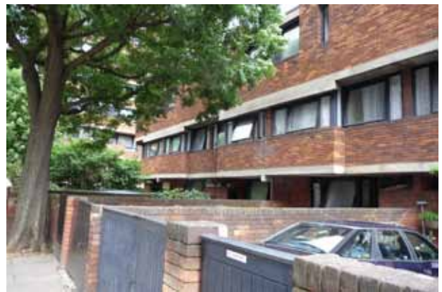
Figures 37-38: Above Charlwood Street elevation of Fairchild House with gates to front parking area and Below garden walls and gates to the rear that open out onto the communal garden.
