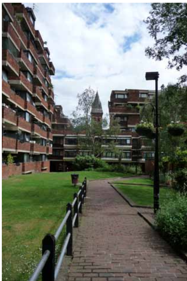
Figure 89: View 1 of the church visible behind Estate blocks; the skyline of which has been designed to better reveal the spire.
