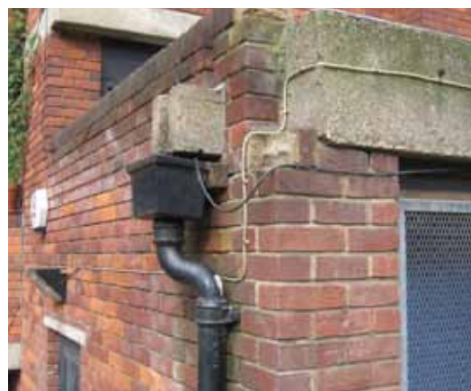
Figures 147-149: above damage to brickwork and below, pipework and wires below overflow chute
