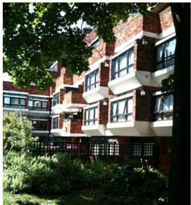
Figure 29: Typical Phase I block showing projecting bay windows of Charlwood House. This detail is only found in Phase I.
