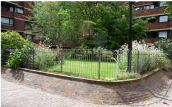
Figure 121-122: Above , brick paviours lining pedestrian walkways; Below , raised brick edging around garden areas, adjacent to Repton House
