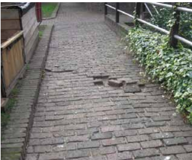
Tachbrook Street would also benefit from enhancement.
