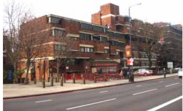
Figures 32 & 33: Charlwood House, Above the Vauxhall Bridge Road elevation steps down in height towards the Church. Access galleries are in-filled with glazed panels. Below Garden elevation of Charlwood house.
