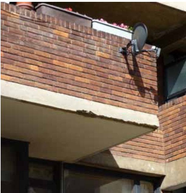
Figures 150-151: Areas of concrete decay in need of repair
