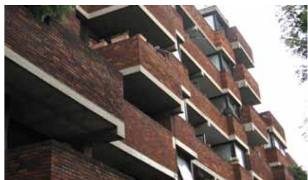
Figures 25 & 26: Above angled canted concrete bands and Below , Angular patterns of balconies creates highly articulated facades.
