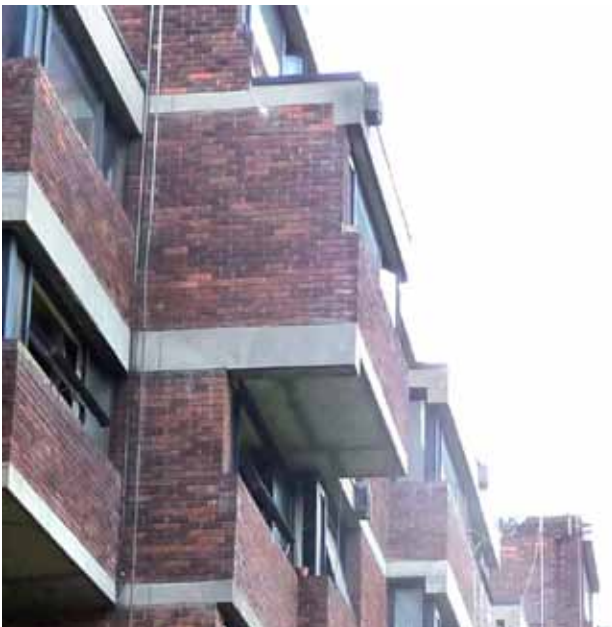
Figure 42 & 43: View of Forsyth House from the gardens and below , the overflow chutes are visible immediately above the windows.
