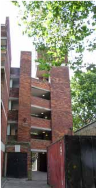
Figure 46: Staircase at the end of Parkinson House
