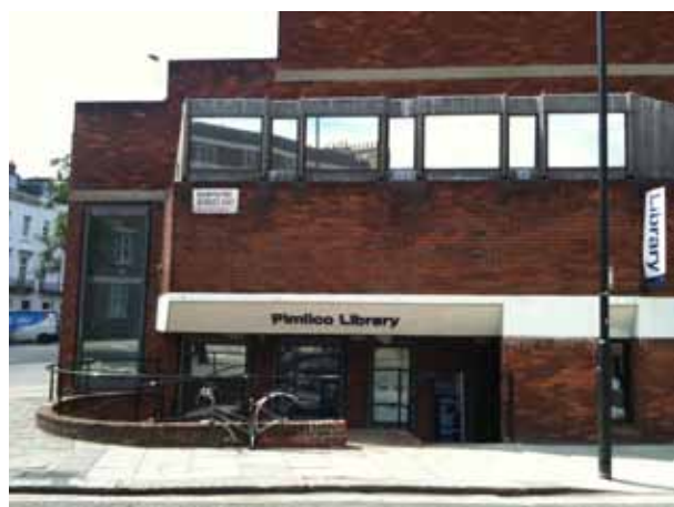
Figure 51: Former Pimlico Library, Rampayne Street
