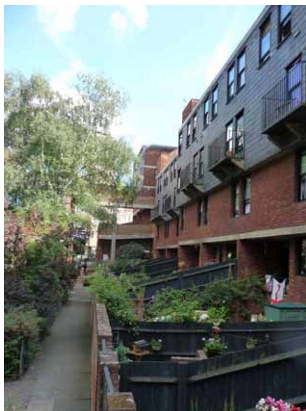
Figure 50: Phase three is characterised by smaller blocks with gardens (Rear of Stourhead House) play an important part in the arrangement of this later phase. These allowed front doors to be provided to access the upper flats and studios allowing for more space to be given up to small private gardens and courts which are a key characteristic of this phase.
