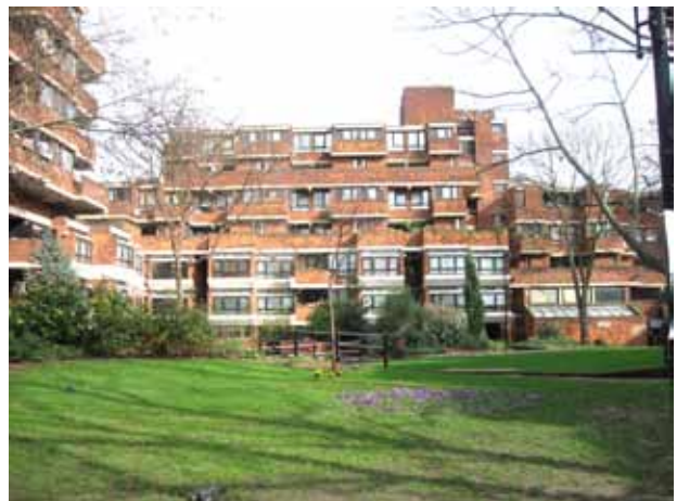
Figures 32 & 33: Charlwood House, Above the Vauxhall Bridge Road elevation steps down in height towards the Church. Access galleries are in-filled with glazed panels. Below Garden elevation of Charlwood house.
