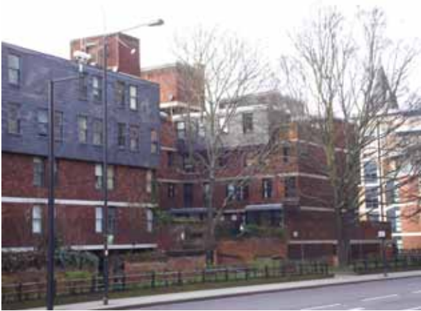
Figure 28: Later phases of development are lower in scale with less articulation to facades. A prominent feature adjacent to the bright red brickwork. Windows and doors are of dark stained timber as are the small access gates to the gardens of individual properties, which add to its domestic character.
