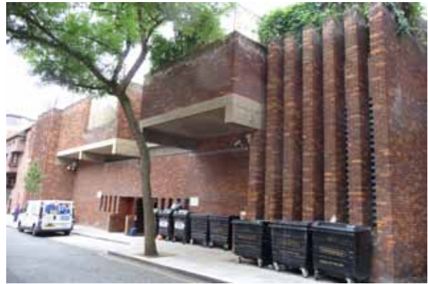
Figure 41: Electricity Transformer Station, Moreton Street elevation
