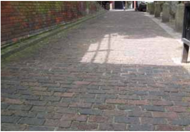
Figure 121-122: Above , brick paviours lining pedestrian walkways; Below , raised brick edging around garden areas, adjacent to Repton House
