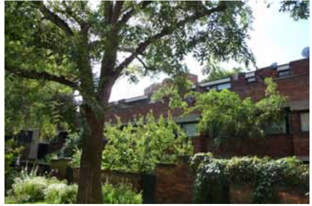
Figure 36: ( above ) Rear rooftop access walk of Fairchild House
