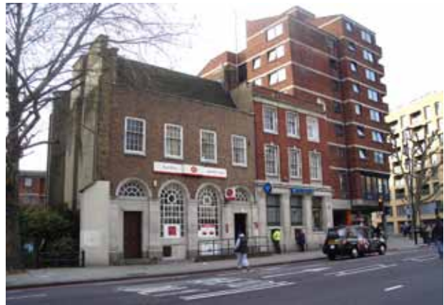
Figures 87: above , Barclays Bank and the Post Office on Vauxhall Bridge Road
