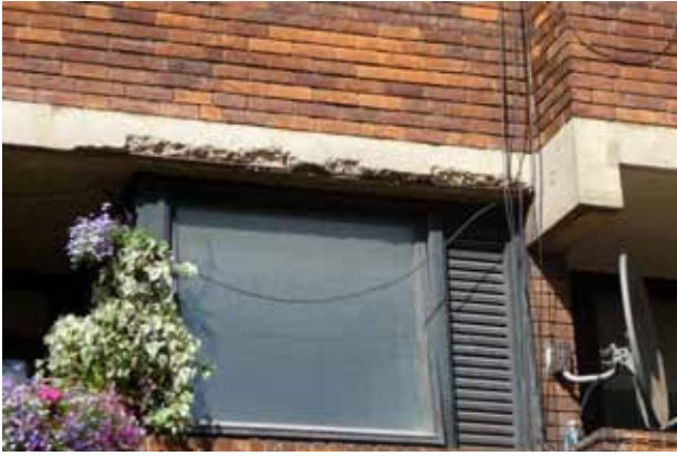
Figures 150-151: Areas of concrete decay in need of repair
