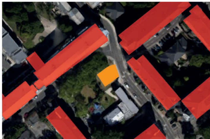
Figure 1: Yellow highlighted area showing potential site setup location in green area outside Greenside Community Centre
