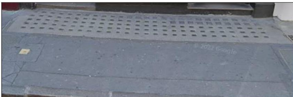
Mastic Asphalt around Basement
