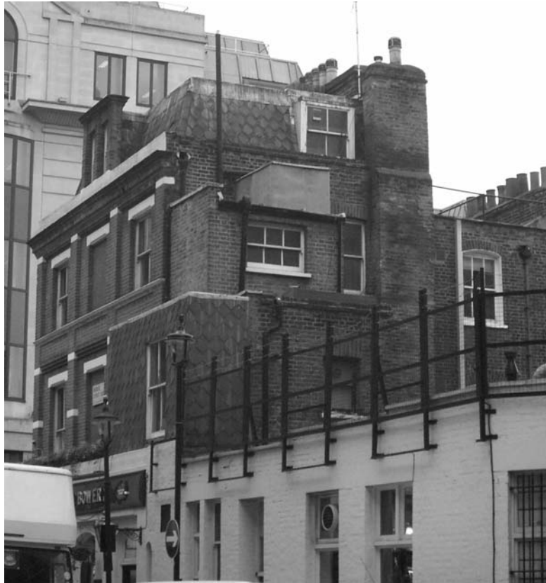
Figure 27: Rear elevation of the White Horse & Bower
