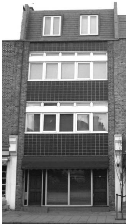
Figure 29: 108 Horseferry Road stands out within the Conservation Area
