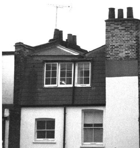
Figure 20: Butterfly roof at no. 116 Horseferry Road, visible from Medway Street
