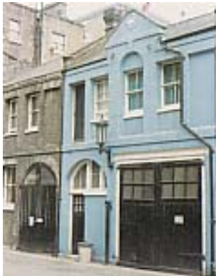
Kendall Place, W1: A mid/late 19th century mews building of 'quasi' classical appearance.
