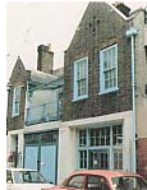
Devonshire Close, W1: Late 19th century example of a mews-house with double carriage space, and balcony on first floor.
