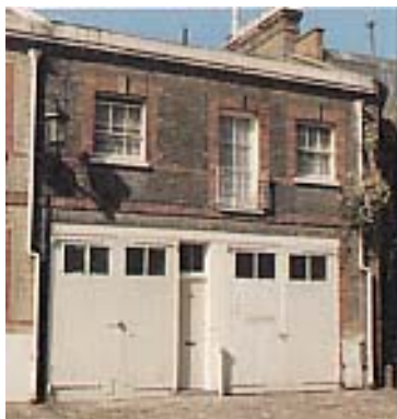
Grosvenor Gardens Mews, SW1: An example of a mews-house in the Grosvenor area. The good quality brick and red-brick bands, motifs and other decoration, are characteristic of the late 19th century when mews buildings were developed as independent houses.
