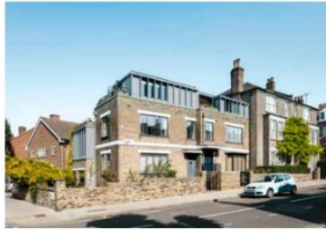
Figure 75: 32 Laurier Road - extra floor added to facilitate family living. Richard Keep Architects (photo credit: Ben Blossom).
