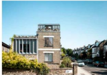
Figure 76: 32 Laurier Road - 2 roof terraces with planting make a positive contribution to the streetscape. Richard Keep Architects (photo credit: Ben Blossom).
