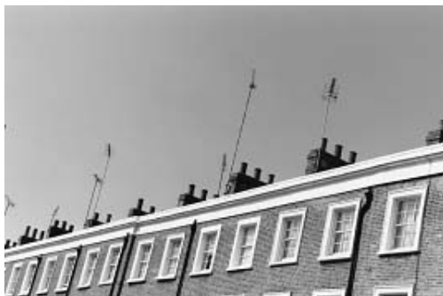
Figure 13a: Uninterrupted rooflines of Ponsonby Terrace
