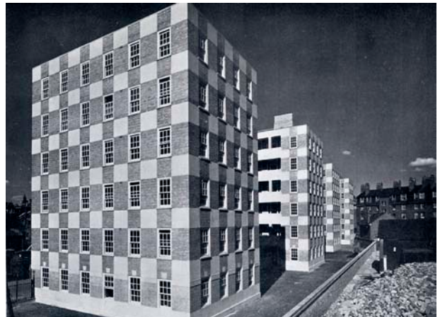
Figure 12: Historic image of the rear of Grosvenor Estate blocks, 1930
