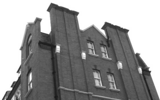
Figure 47: Gable end with tall chimneys to Probyn House
