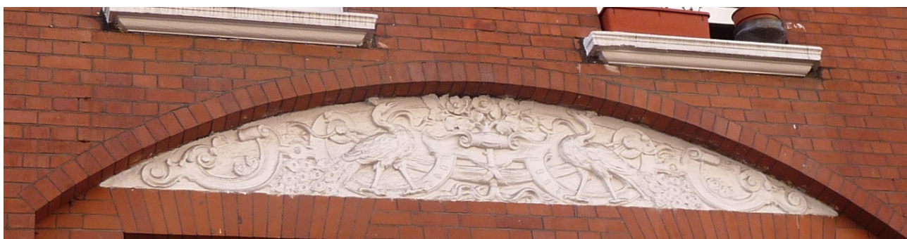
Figure 23: Decorative stucco panels to Regency Estate
