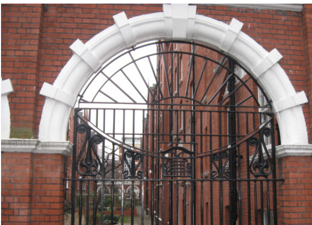
Figure 55: Modern welded steel infills above original railings
