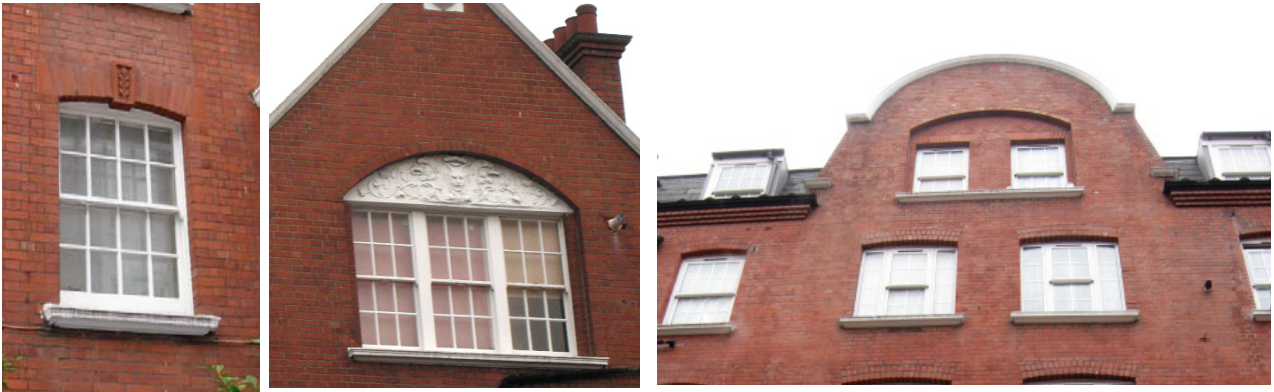
Figures 24-27: Original sash window detail; tripartite window below pointed gable; arched gable; and doorway with door hood ( below )
