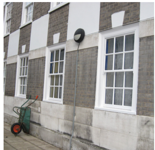
Figures 39-41: (left to right) Entrance door detail to gallery side, entrance to, and sash window detail to ground floor with keystone above.
