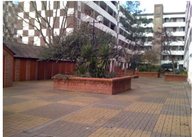
Figure 72: Unsympathetic late 20th century paving between Rogers House and Tothill House
