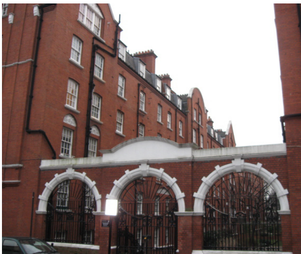
Figure 51: All of the blocks on the Regency Street estate, including associated screens are considered to be of merit.
