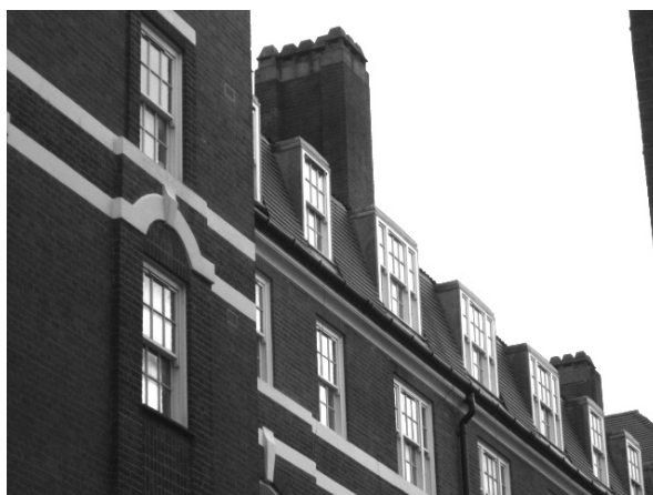
Figure 48: Mansard roof with dormers to Schomberg House
