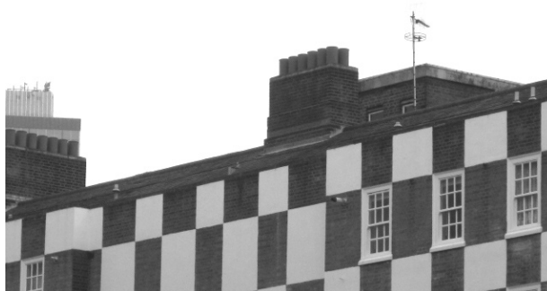
Figure 49: Roofscape to Grosvenor Estate
