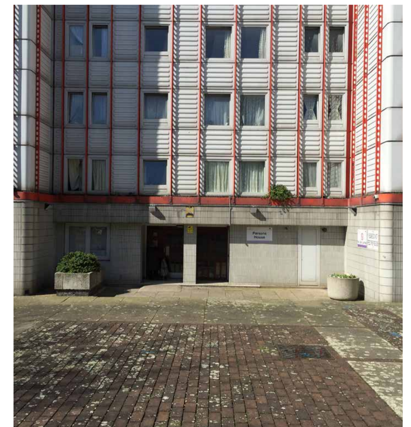
Existing entrance to Parsons House
