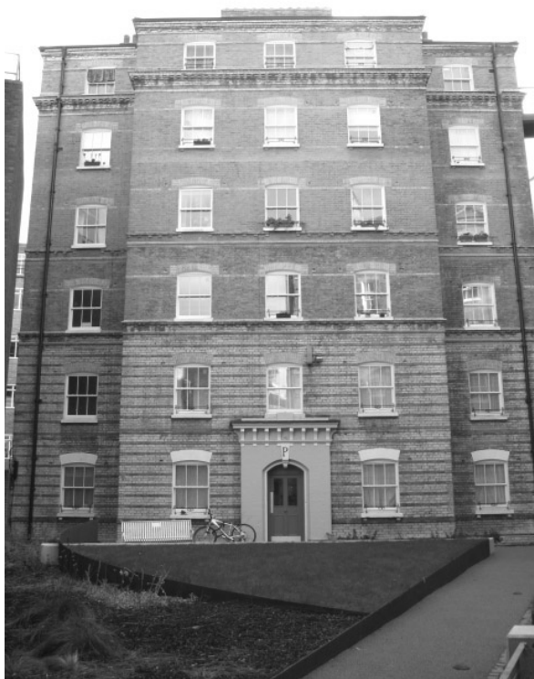
Figure 32: Block P, southern section of Abbey Orchard Estate
