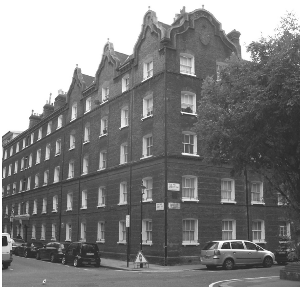
Figure 18: North-eastern corner (Blocks C&D) of Old Pye Street estate with original Dutch-style gables
