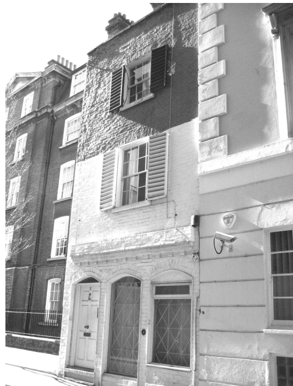
Figure 115: No 2 Chadwick Street
