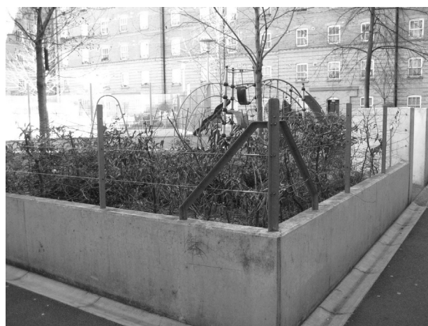
Figures 90 - 92: (top to bottom) Peabody Avenue Memorial Garden; Abbey Orchard Estate's metal retainer to plant beds; Abbey Orchard Estate's concrete planter with metal retainers
