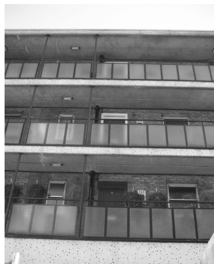
Figure 34: Access balcony on St Ann's Lane House, Abbey Orchard Estate
