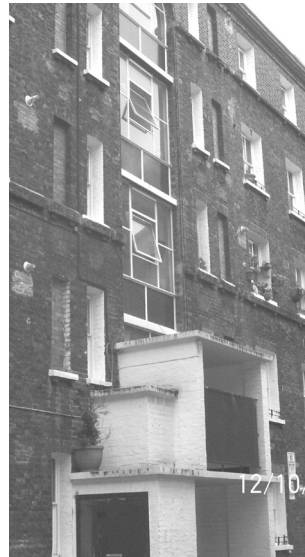
Figures 95 and 96: (left) Enclosed stairwell, and (below) lift shaft to Old Pye Street Estate
