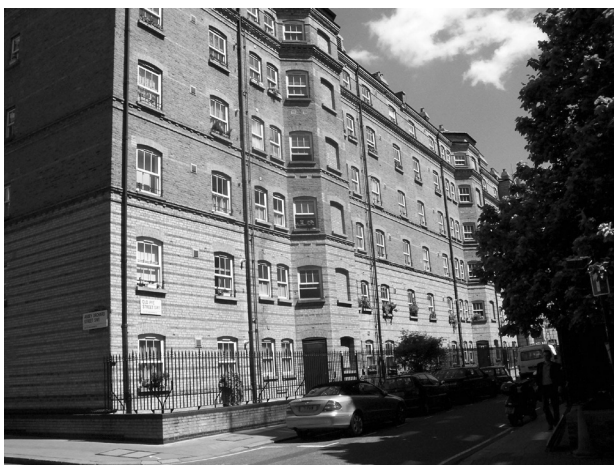
Figure 28: Southern facade of northern section of the Abbey Orchard Estate
