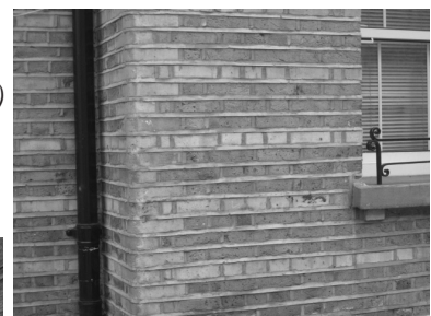
Figures 97-100: (below) Vacant Blocks Z & X respectively; (top right) poor repointing to western blocks of Peabody Avenue; and (bottom right) good quality pointing of Peabody Avenue's eastern blocks.
