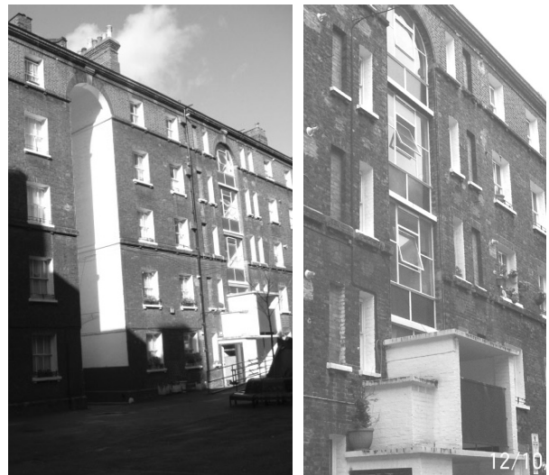
Figures 20-21: Arched opening to entrance, infilled doorways to original Block D, Old Pye Street Estate
