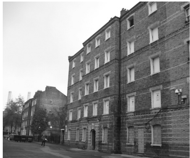
Figure 53: Block X, demolition of which has been granted consent
