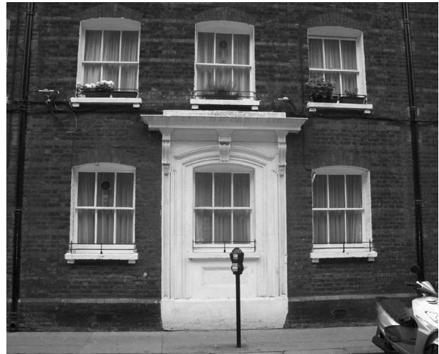
Figure 19: Central window on northern facade with white surround.
