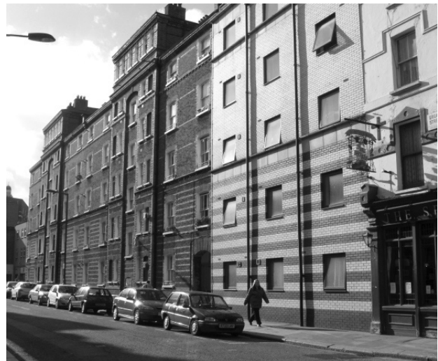
Figure 24: Great Peter Street elevation of Old Pye Street Estate
