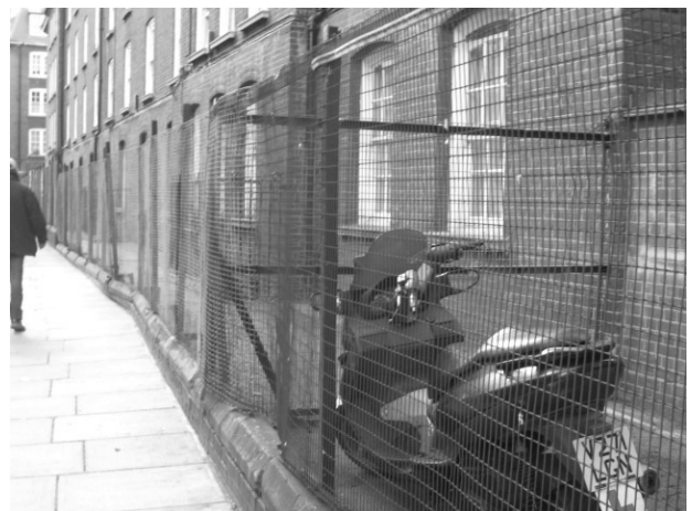
Figure 110: Poor quality metal fencing to the boundary of Horseferry Road Estate
