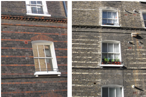
Figures 22-23: Brickwork to earlier blocks ( left ) and later blocks ( right )
