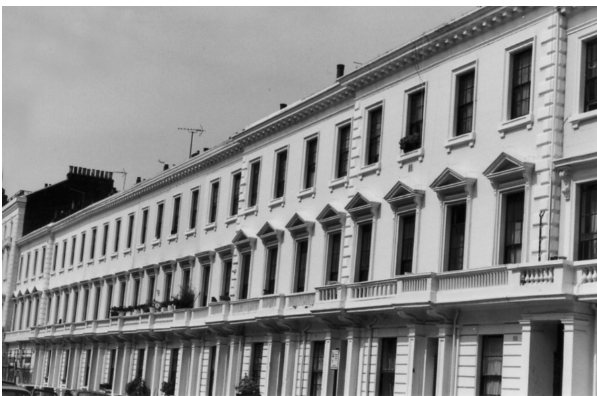
Figure 32: Pimlico terrace with a consistent roofline, uninterrupted by roof extensions
