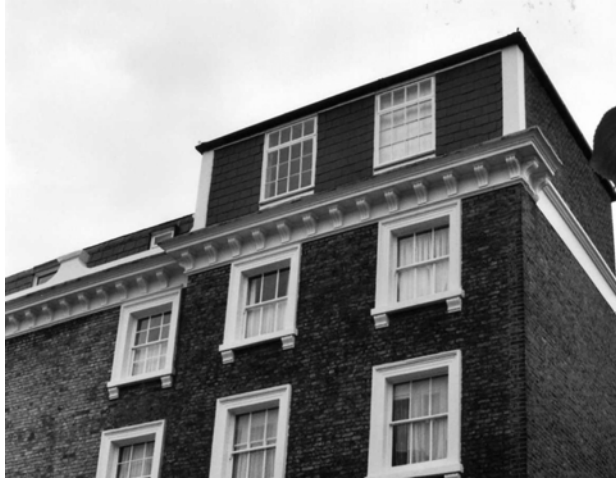
Figure 53. This sheer roof storey which is highly prominent and poorly detailed, with windows which do not match those in the existing building, and has been clad in slate to the street elevation.
