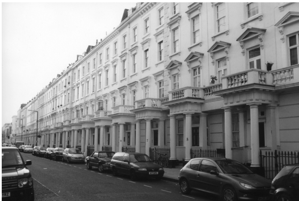
Figure 7: The grander Pimlico terraces are of 4-5 stories and show a full range of classical details; columned porticos, rusticated stucco to the ground floor, bottle balustrades, pedimented windows to the first floor, and dentil cornice to the parapet, behind which the roof structure is hidden.
