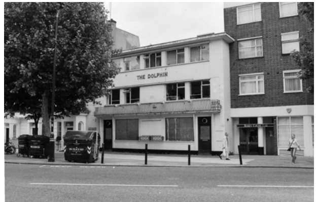
Figure 55: 114-118 Denbigh Street. This vacant public house, besides being an infill development of inappropriate design and scale, is vacant and in a poor state of repair.
