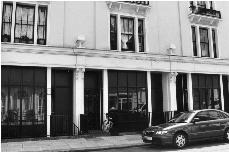
Figure 40: Shopfronts along Denbigh Place
