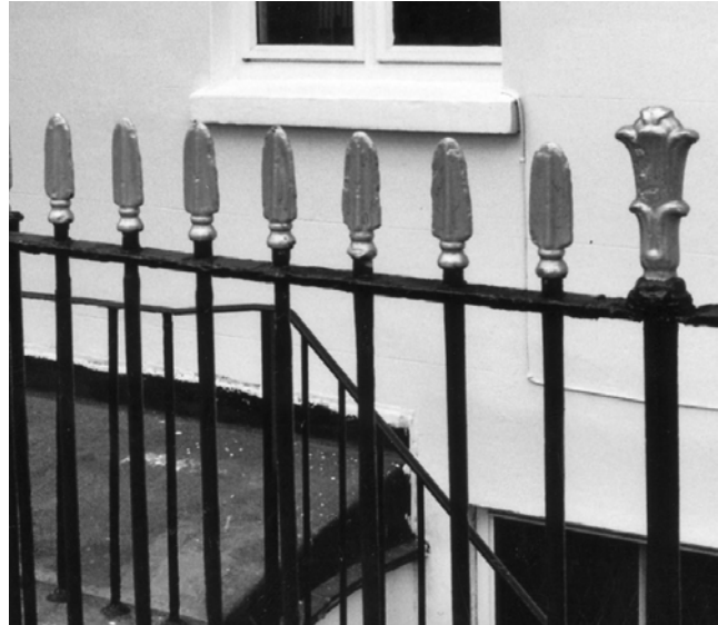
Figure 39: Typical spearhead finials. The use of metallic paint on finials is discouraged.
