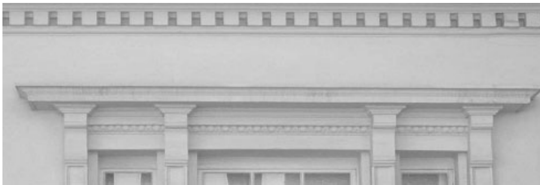
Figure 12: Stucco window surround
