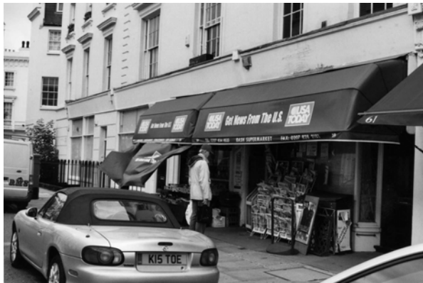
Figure 54: 59 Cambridge Street. This canopy is both crudely designed and manufactured in an inappropriate material for the shopfront.
