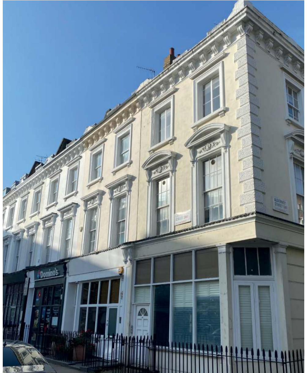
Sussex Street and Charwood Street – where shops are converted to residential without changing the shop front the loss of the shop/citylife can become very evident.
