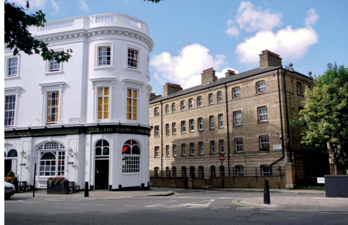
The junction of Sutherland Street and Turpentine Lane showing the Peabody Estate.
