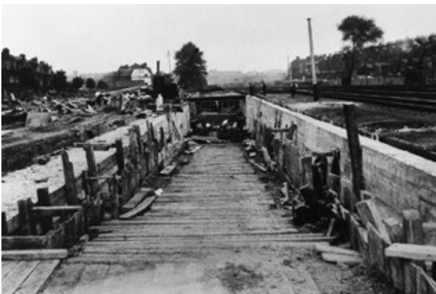
Bakerloo and Watford Junction extension, to include a station at Queen's Park, 1914
