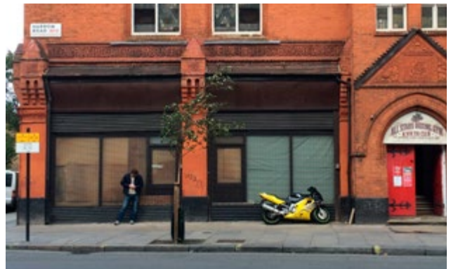
The vacant units on the ground floor of the Queen's Park Community Hall could be vibrant shop fronts to serve the local community as originally intended
