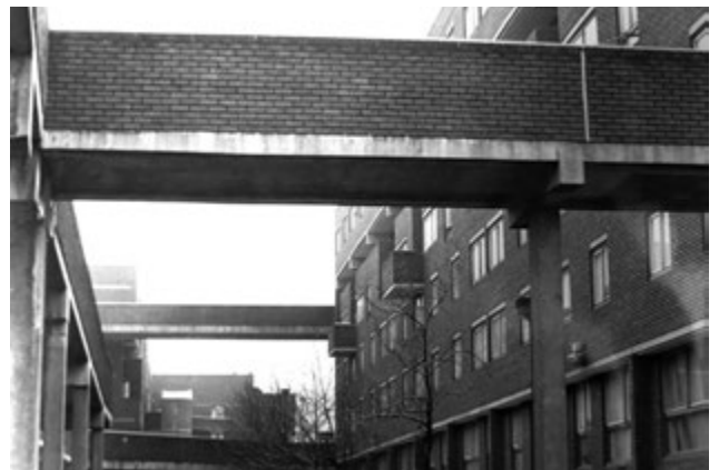
The original layout of the Mozart Estate with the now removed bridges between housing blocks, 1977
