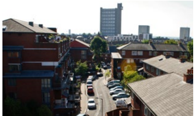
④ The Mozart Estate is made up of a variety of housing types with some housing blocks of up to seven storeys on Lancefield Street. Trelick Tower, in North Kensington is seen in the background Source: Flickr, Author: Nico Hogg
