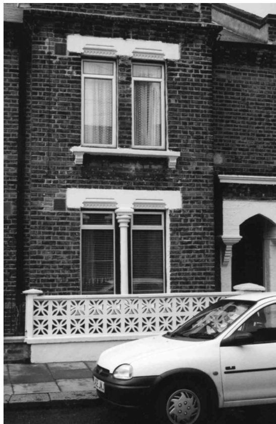
Figure 27: Small scale building alterations including replacement windows, painting and changes to boundary walls.
