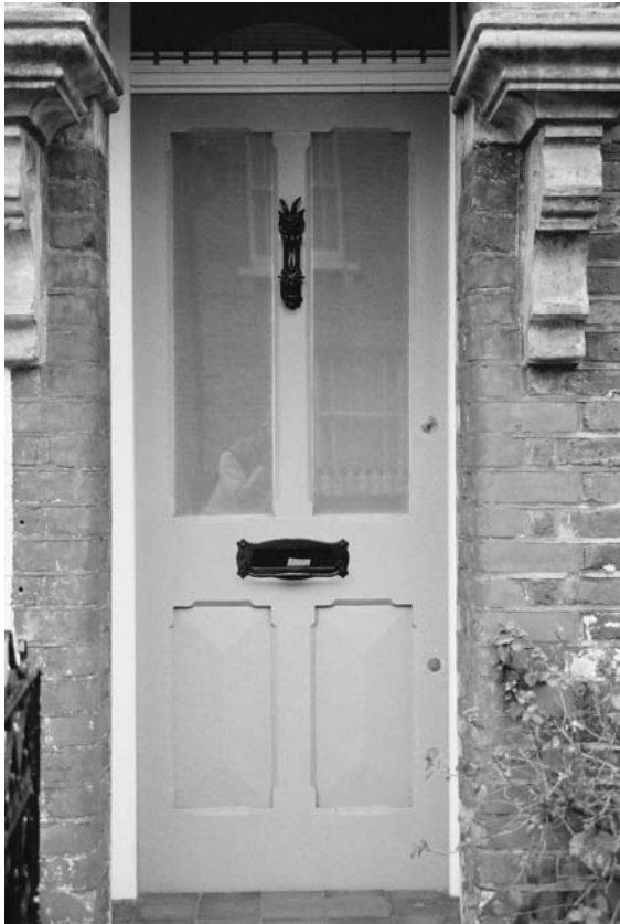
Figure 17: Typical door with cast iron goats head knocker and cast iron letter box.
