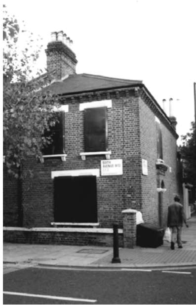
Figure 30. Boarded up windows and doors on Sixth Avenue
