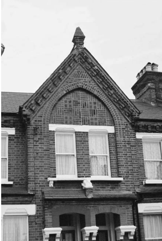
Gable with polychromatic brickwork
