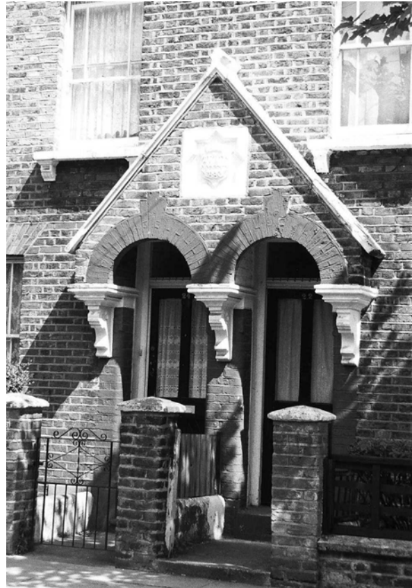
Figure 18: The most common type of porch hood, over double doorways, with pointed gable containing the badge of the artisans company and supported on corbels.
