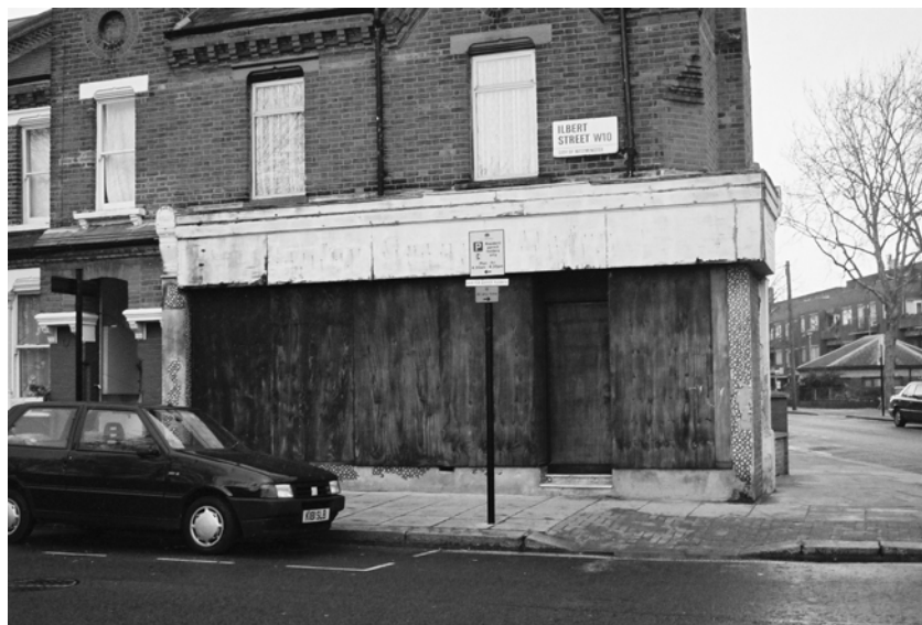
Figure 28. Disused shop on Ilbert Street
