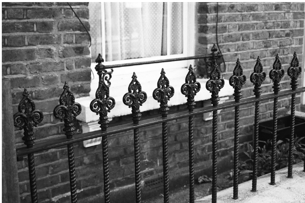
Figure 25: Typical front boundary railings, reinstated to traditional design.
