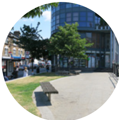
The elegant frontage of the recently refurbished library on Harrow Road
