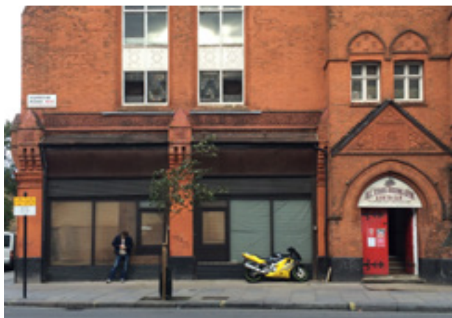
The vacant units on the ground floor of the Queen's Park Community Hall could be vibrant shop fronts to serve the local community as originally intended
