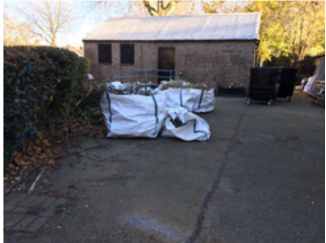
Maintenance hut as it is currently
