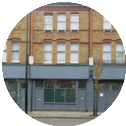
① Blank frontages along Canal Terrace where there once was an active retail parade
