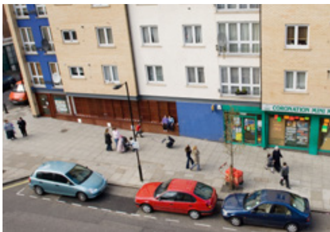
The community centre and convenience store on Dart Street
