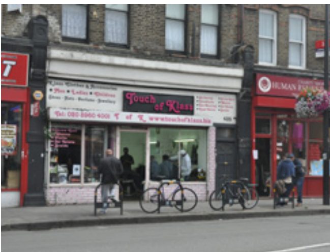
The high streets at the south, west and north edges of the area have more mixed uses
