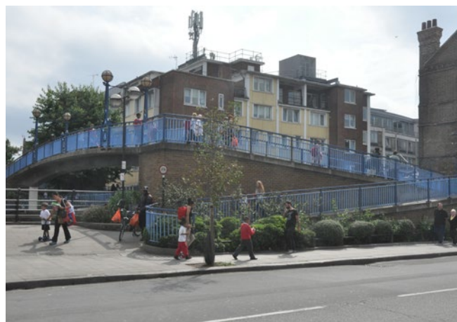
The busy Half Penny Steps crossing is the area's only pedestrian route across the canal which connects to the workspaces, parks and residential neighbourhoods of Kensal Road
