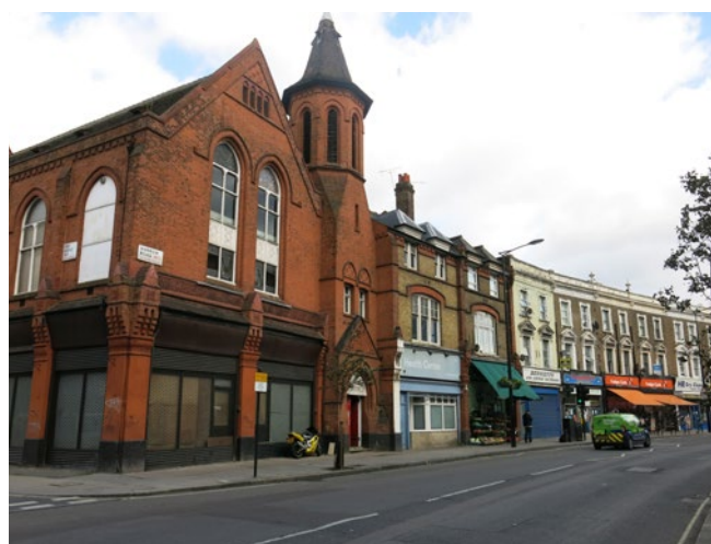
Grade II listed Queen's Park Meeting Hall, 578–580 Harrow Road. 1883–1884. Architect, Rowland Plumbe for the Artisans, Labourers and General Dwellings Company. The hall was built as a centre for the social life of the Queen's Park Cottage Estate, for meetings, non-alcoholic refreshment, entertainment and education with shops below for the use and profit of the community as a whole
