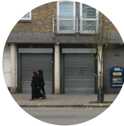
② There are a large number of apparently vacant units on the Harrow Road high street
