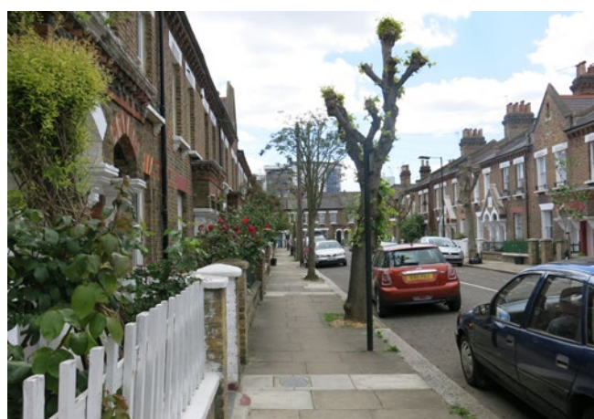
The majority of streets in the area are very quiet with little pedestrian activity
