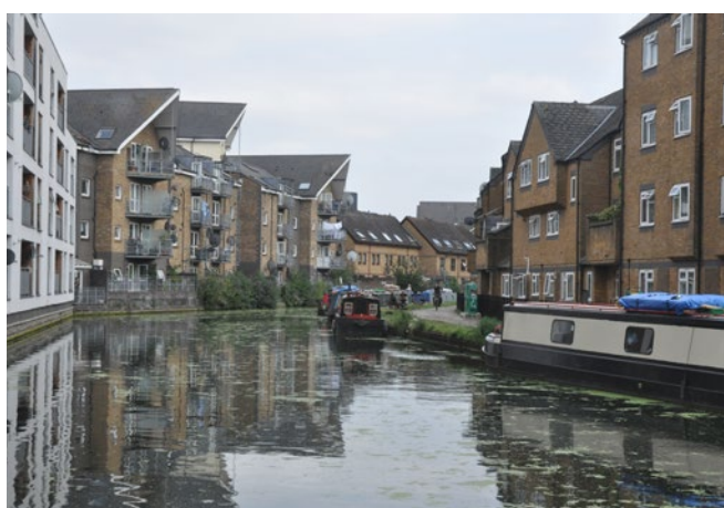
The adjacency of the Harrow Road to the Grand Union canal is an unusual and characterful feature of the high street
