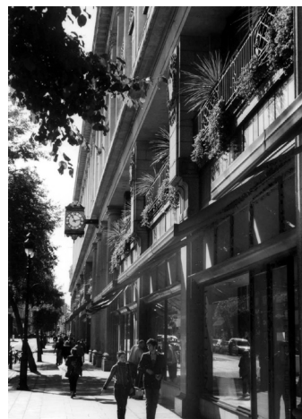
Figure 67: Whiteleys shopfronts detail, showing the traditional canvas blinds
