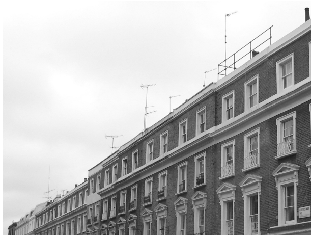
Figure 48: Victorian terraces with roofs set behind parapet cornice
