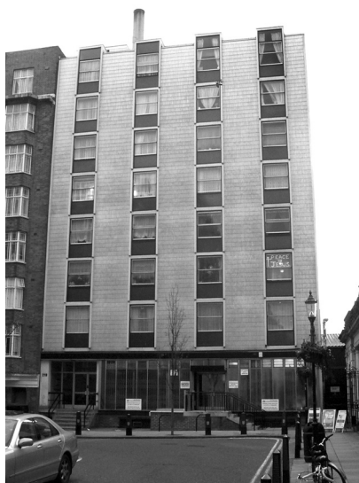
Figure 92: Bridge Field House
