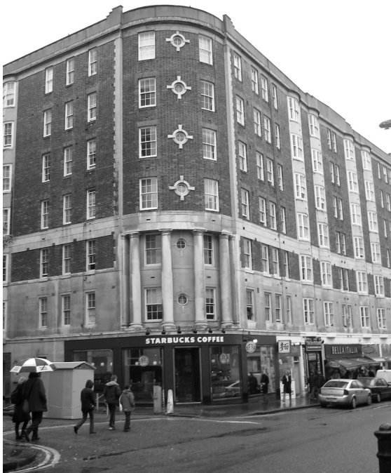
Figure 27: Princess Court, nos. 47 - 63 Queensway
