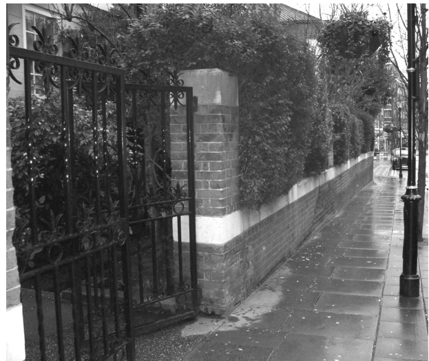
Figure 63: Boundary treatment, Claremont Court
