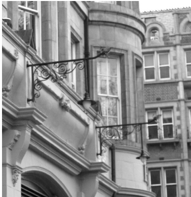
Figure 58: Ornate lamp brackets attached to Queensway Underground
