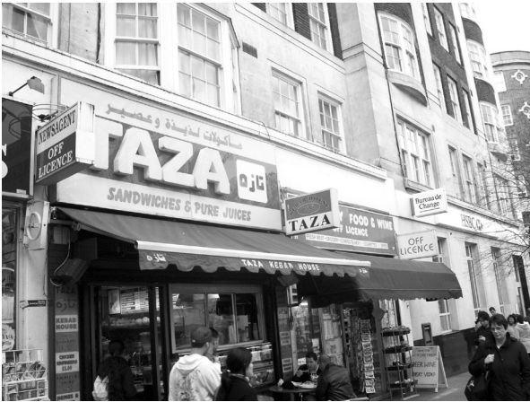
Figure 84: Projecting box signs, oversize plastic lettering and blinds
