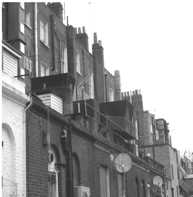
Figure 88: Plant to the rear of Queensway
