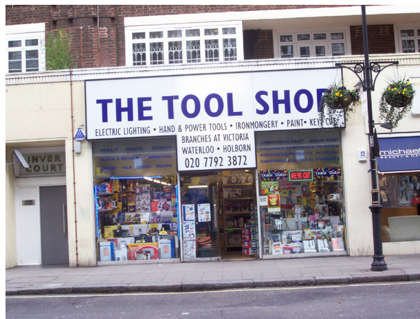
Figure 81: This over large fascia has been affixed to the original stone surround, ignoring the proportions established in the design of the original building
