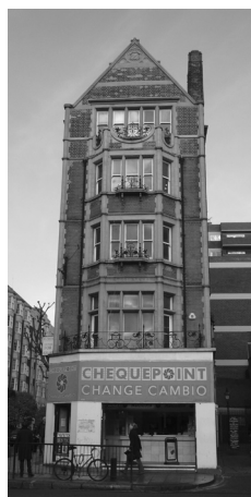
Figure 82: this shopfront to Bayswater Road has been built out, with a large unsubdivided fascia in modern materials which extends to the base of the window, overpowering and obscuring detail to Victorian building above.
