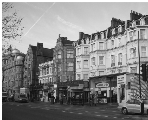
Figure 9: The Bayswater Road Frontage
