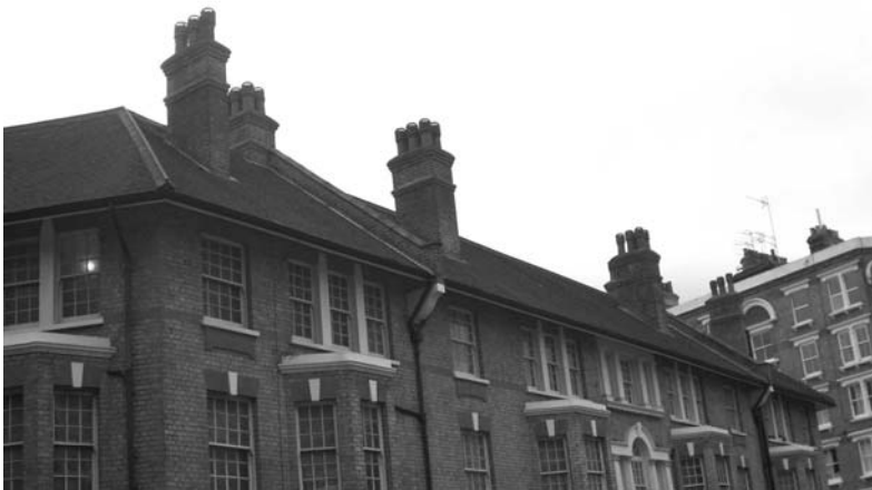
Figure 22: Chapter, Esterbrooke and Regency Street, dwellings have pitched tiled roofs with overhanging eaves. Roofs are subdivided by stout brick chimney stacks
