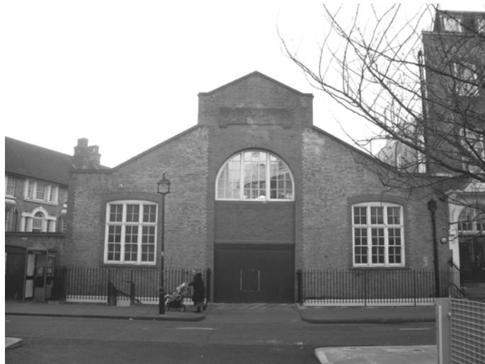
Figure 10: 56 Regency Street, rear (southern) block. Two tripartite windows flank a former entrance doorway, above which is a large semicircular window and raised, shaped gable
