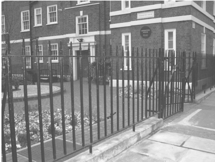
Figure 30 – Railings to Middleton House
