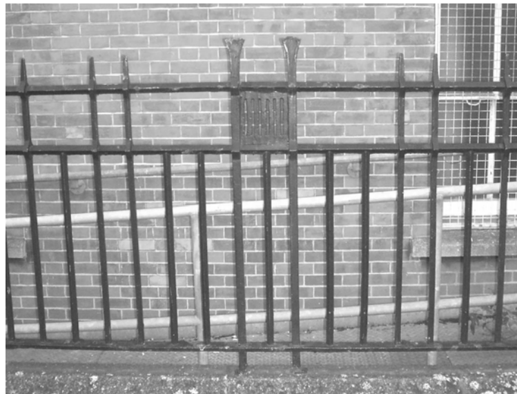
Figure 29 – Railings to Peel House
