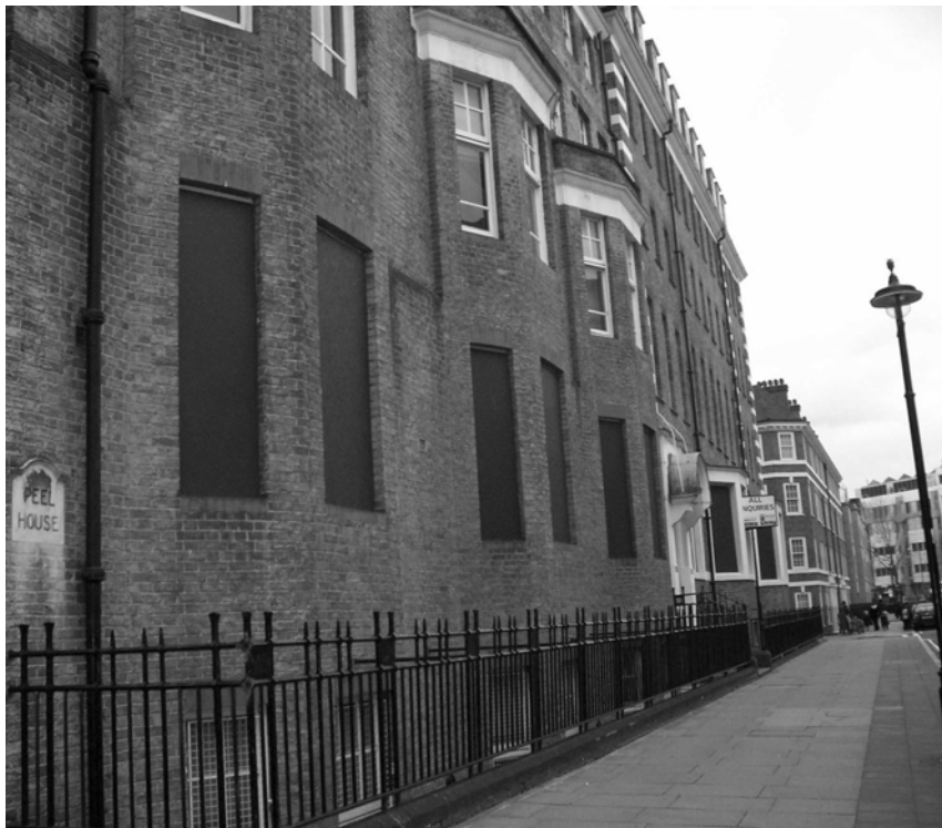
Figure 35: Boarded up windows to Peel House
