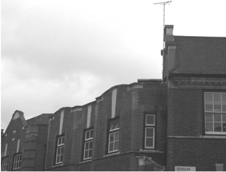
Figure 24: 112 Regency street has an unusual roof form with a pitched roof to the front block and flat roof set behind Dutch Gables to the rear. The rear has permission for a roof extension
