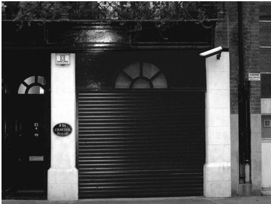
Figure 37: Roller shutter at 13 Chapter Street
