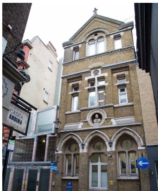
Soho Parish Primary School
