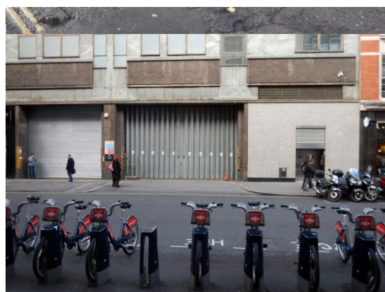
Service entrances along Great Marlborough Street.
