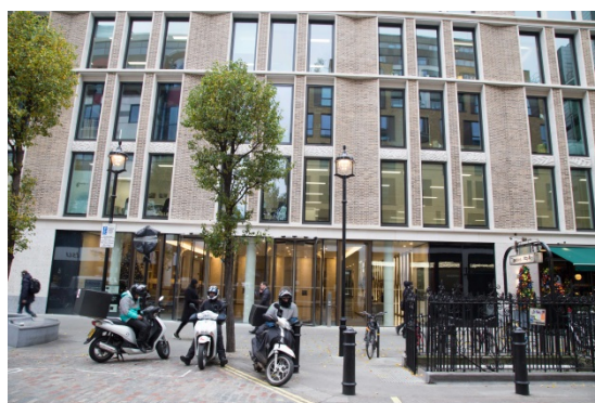
Vacant lobby along Broadwick Street
