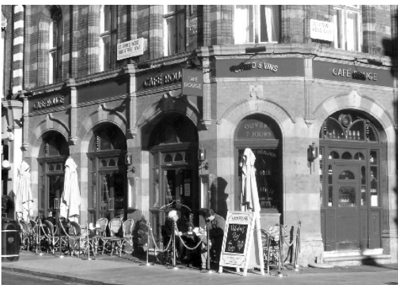
Figure 73 : 60 St John's Wood High Street
