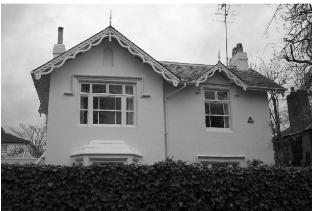
Figure 38: Barge Boards, Norfolk Road
