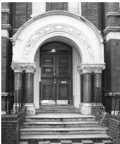
Figure 45-47: Left-right. Double timber doors in elaborate surround to Victorian Mansion block; 1950s flush door in simple surround; 1930s flush door, with projecting canopy above, Hamilton Terrace.
