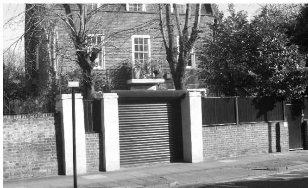
Figure 115: Roller shutter inserted in place of a front gate, Abbey Road
