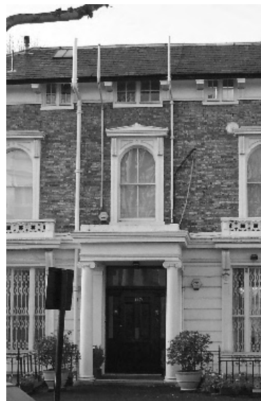
Figure 118: Pipework and burglar alarms can contribute to visual clutter
