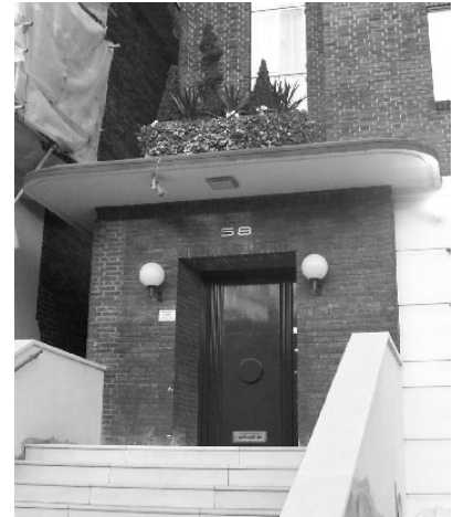
Figure 45-47: Left-right. Double timber doors in elaborate surround to Victorian Mansion block; 1950s flush door in simple surround; 1930s flush door, with projecting canopy above, Hamilton Terrace.
