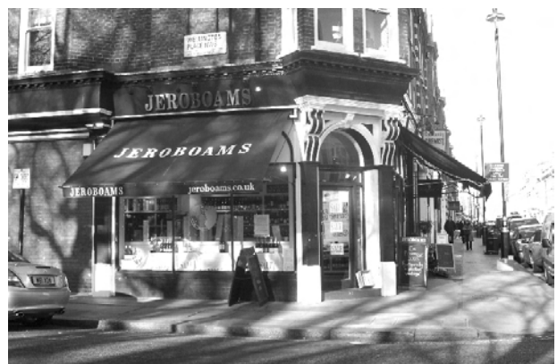
Figure 71: 1 St John's Wood High Street. An attractive early 20th Century corner shopfront with splayed corner entrance. The fascia is set below a projecting dentil cornice, a detail continued along the length of this group until no 59.
