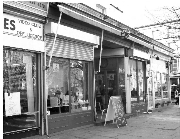
Figure 123: Security Shutters, Abbey Road
