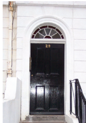
Figures 42-44: Examples of original four panelled timber doors, with a variety of fanlights.
