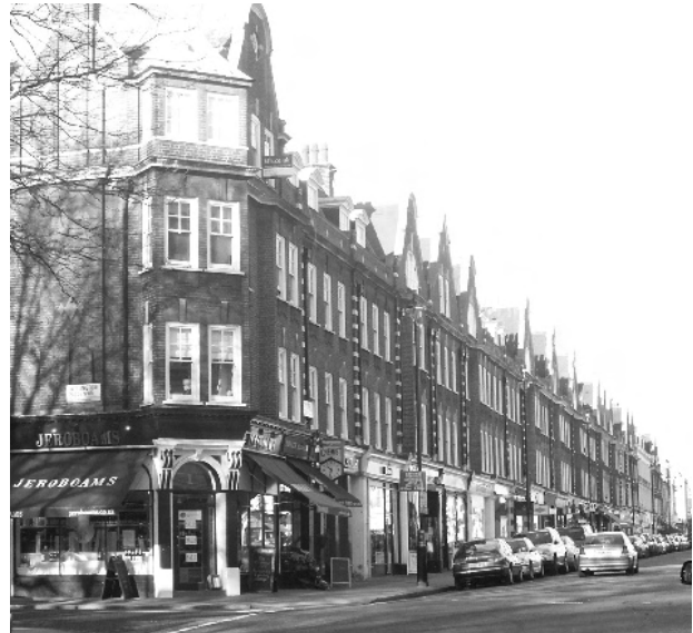
Figure 70: The western side of St John's Wood High Street
