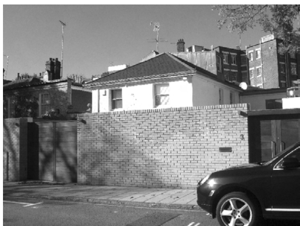
Figure 114: High boundary wall, rebuilt in materials which do not relate to the villa behind
