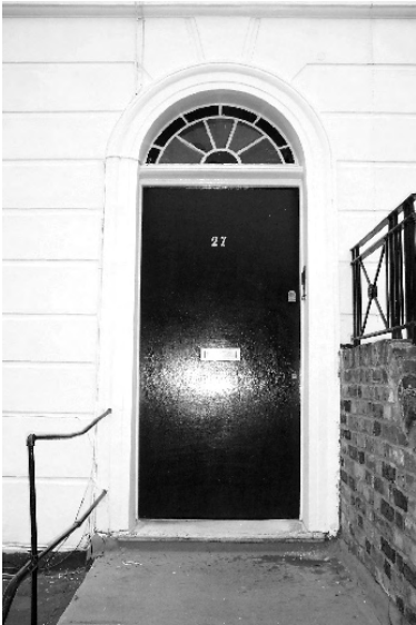
Figure 117: Replacement flush door
