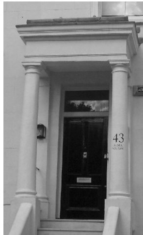
Figures 35-37: top left, simple gothic style porch with pointed arch; Top right, grander portico with Tuscan columns and Bottom left, most common style of plain stucco porch
