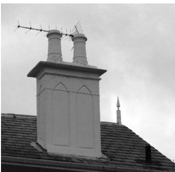
Figure 48: Chimney stack and pots, Norfolk Road
