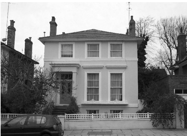
Figure 16: Typical Italianate villa in stucco, with low pitched roof
