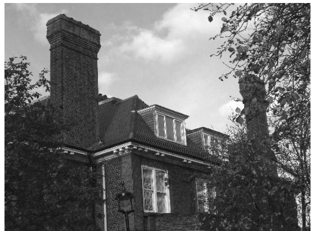
Figure 55: A clay tiled roof with distinctive red brick chimneys
