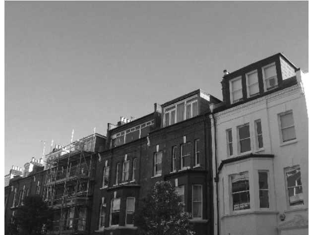
Figure 120: Large dormers to Hamilton Gardens
