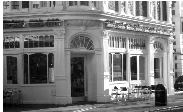
Figure 74: 120 St John's Wood High Street
