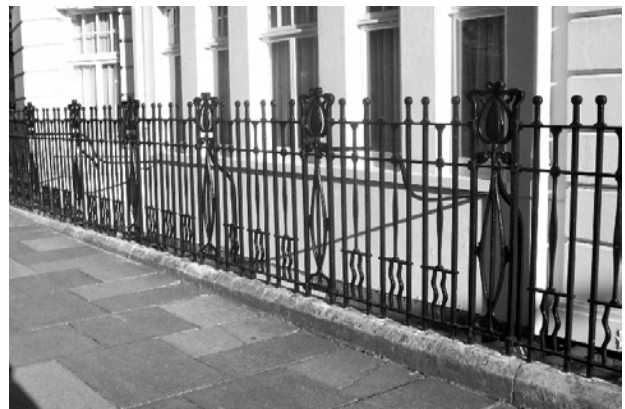
Figure 83: Edwardian railings to mansion block, set in low plinth. This is not a typical detail within the St John's Wood Conservation Area but found at its southern fringes
