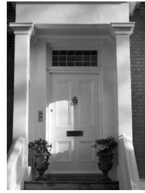
Figures 42-44: Examples of original four panelled timber doors, with a variety of fanlights.
