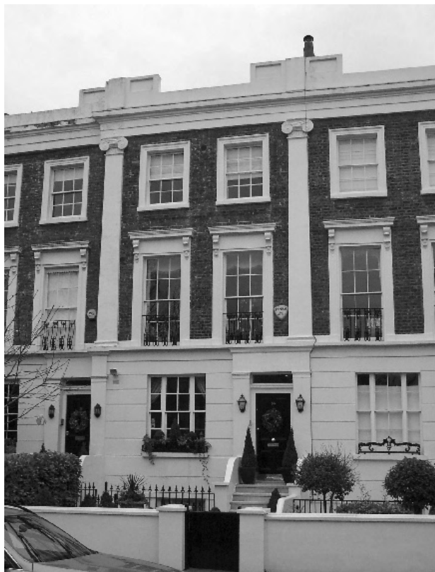
Figure 32: Sash windows with stucco surrounds, set between giant pilasters; Queens Grove Terrace
