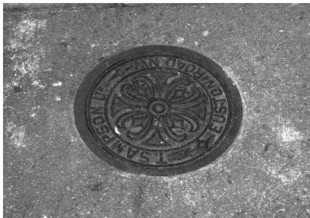
Figure 101: Coal hole cover
