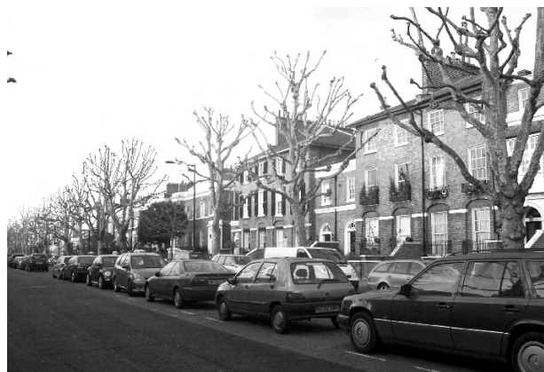
Figure 10: Hamilton Terrace, Southern end.
