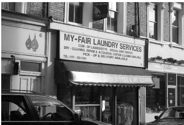
Figure 122: Shopfront, Nugent Terrace
