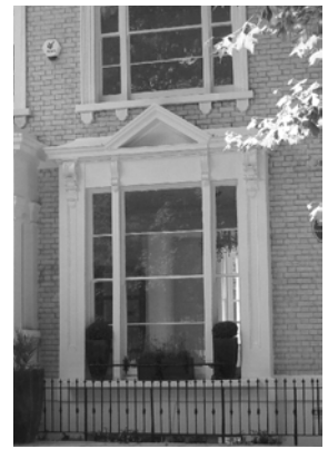
Figures 39-41: Top left, six-over-six round-headed window, Aberdeen Terrace; Timber casement window in Gothic surround, Loudon Road; Unusual tripartite 2-2 sash windows set in pedimented stucco surround, Malborough Hill.
