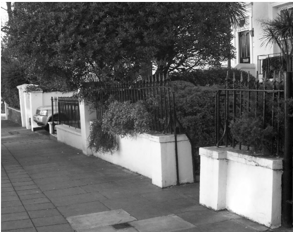
Figure 80: Spearhead railings to half stucco wall, Acacia Road
