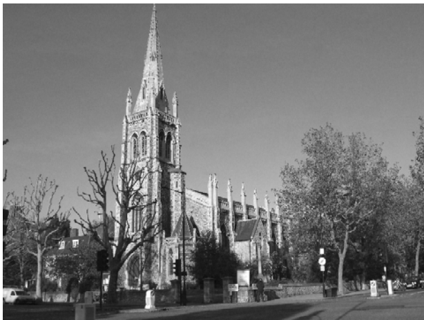
Figure 58: St Mark's Church
