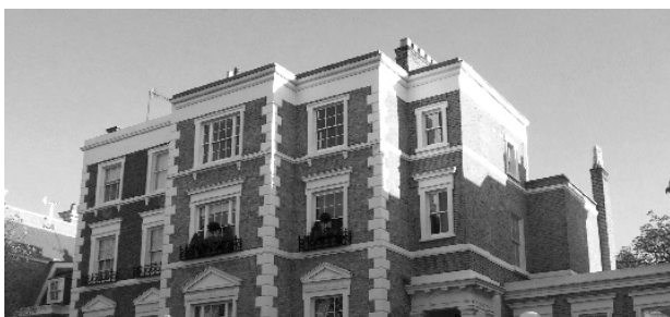
Figure 49: Roof set behind parapet
