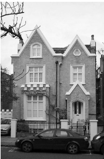
Figure 19: Gothic Villa on Carlton Hill, with castellated bay window, stone tracery, pointed gables and porch
