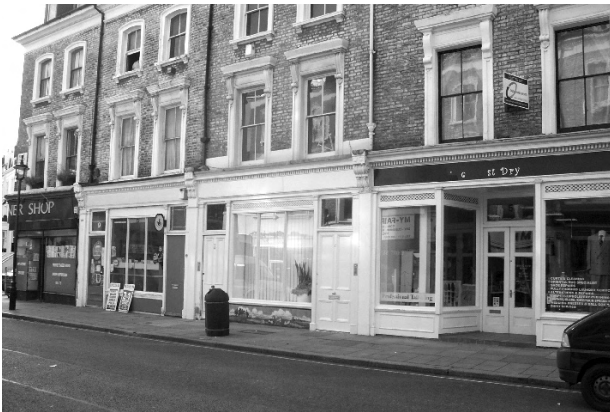
Figure 77: Shopfronts on Nugent Terrace
